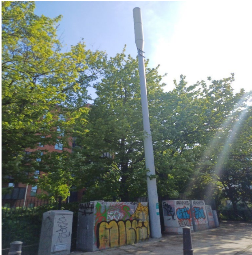
Figure 3.3 A well-designed pedestrian space incorporating DCI, where the monopole and cabinets are sited on the periphery to avoid restricting movement.
