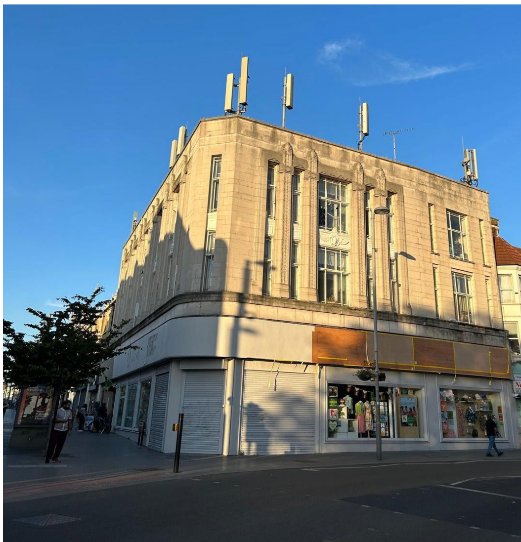
Figure 3.1 Building within a conservation area with poorly located DCI that is highly visible and dominates the building roofline.
