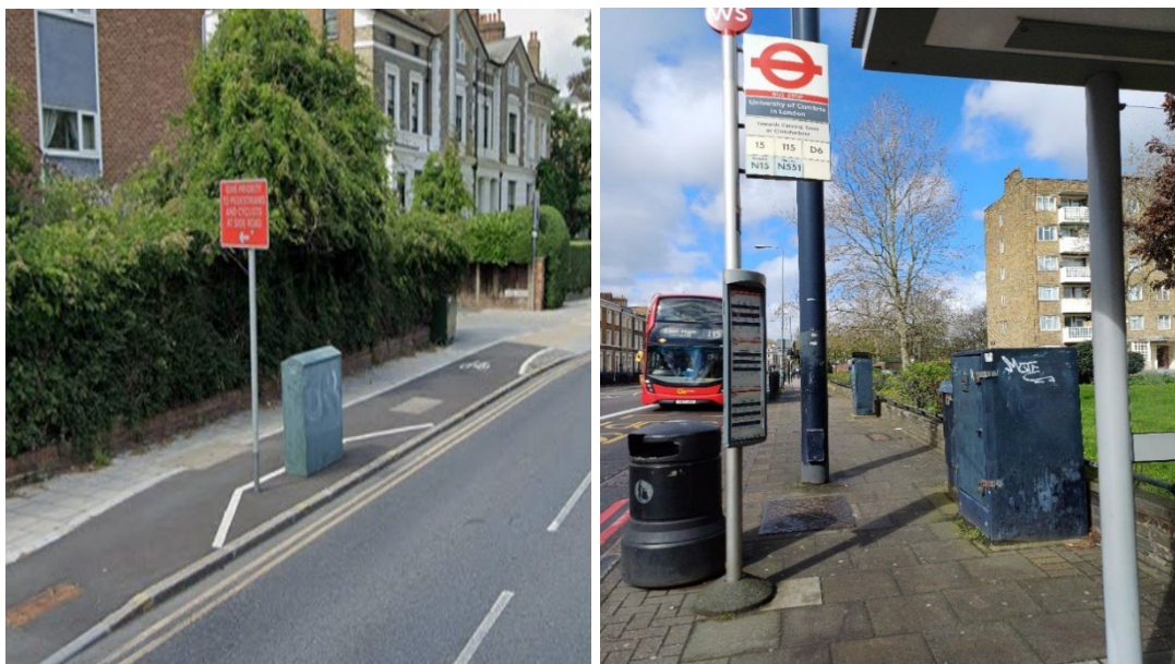
Figure 3.2 Examples of poor siting where siting of DCI obstructs and restricts movement for pedestrians and/or cyclists.
