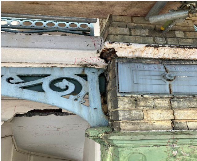
Steel arches are pulling out of the pier. Split Patress Plate. Cracked brickwork.
