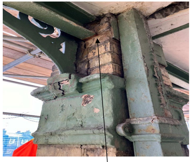
Beam ends are corroded.
