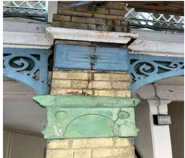
Steel arches are pulling out of the pier. Split Patress Plate. Cracked brickwork.
