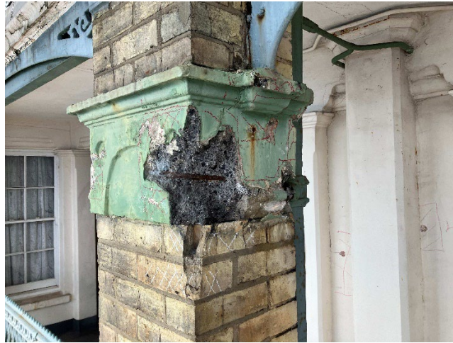
Concrete padstone constructed within the pier with rendered finish.
