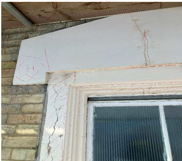
Render panels over the windows have blown.
