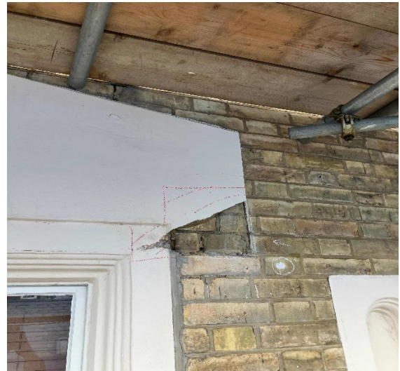
Render panels over the windows have blown.
