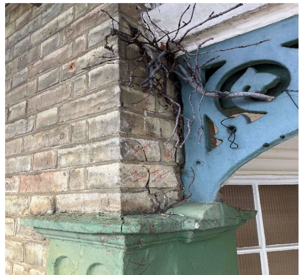
Vegetation growing out of the structure.
