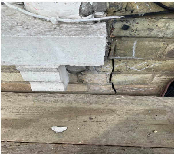
Cracking within the brickwork under the window.
