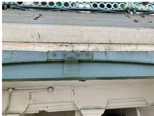
Brackets welded to the landing beams to support the steel arch.
