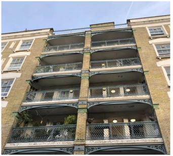
N.B. Only one side will be exposed at any time and one floor. Props will be installed top to bottom. Works to be carried out from the top down the structure.
