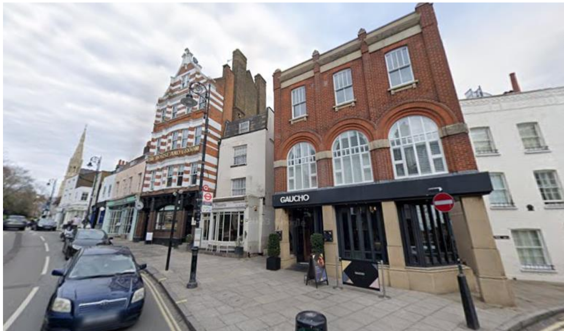
Figure 6. The no. 66 Heath Street and The Horse and Groom Public House (Source: Google Maps).
