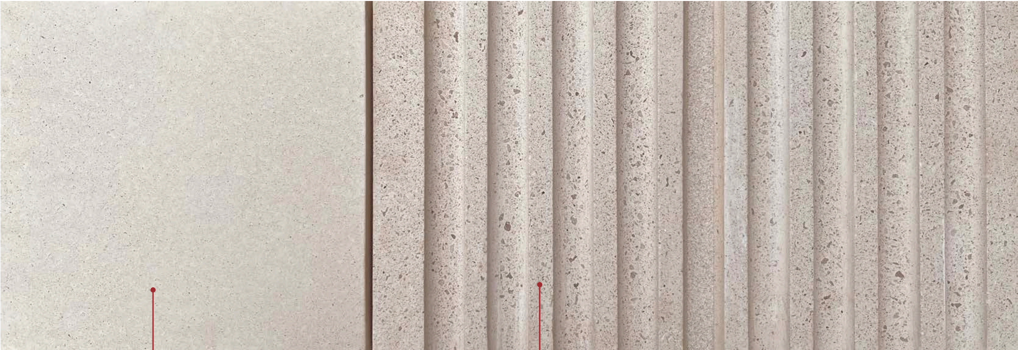
Proposed precast sample with light etch finish and no flutes for Ground Floor piers
