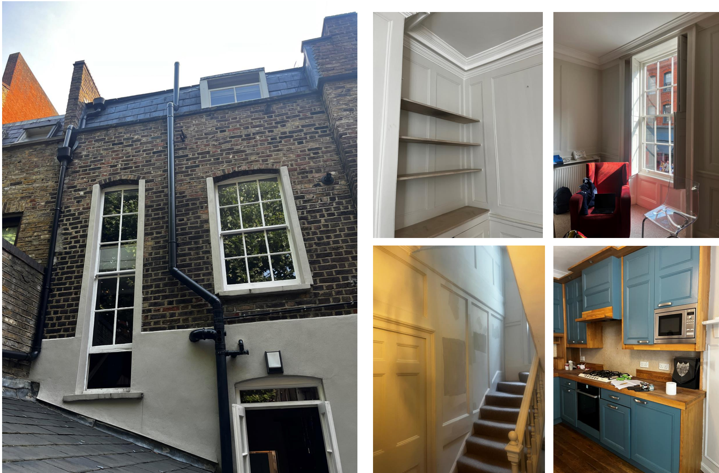
Figure 11: Left: existing rear elevation with cementitious render applied to first floor and to window reveals. Right from top left: Original panelling and cornice to first floor front room with modern shelving; historic window to first floor front room; panelling to stair compartment; and, modern kitchen to first floor rear room applied over original panelling with modern fire surround and applied modern mouldings to right.
