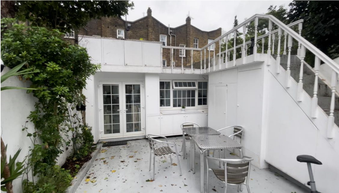
Figure 3 Existing View of 2004 Extension
