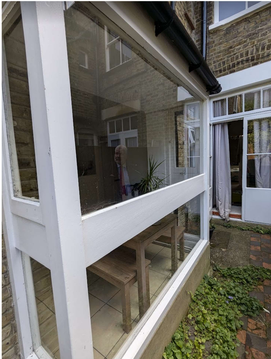
Projecting bay window on the existing side elevation
