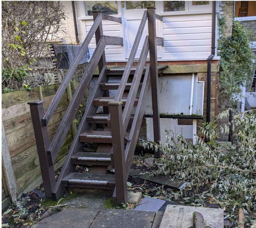
Existing rear staircase over redundant external WC
