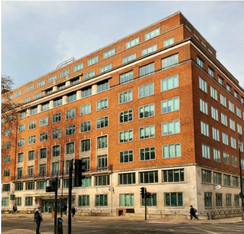
1. Front elevation of Tavis House
