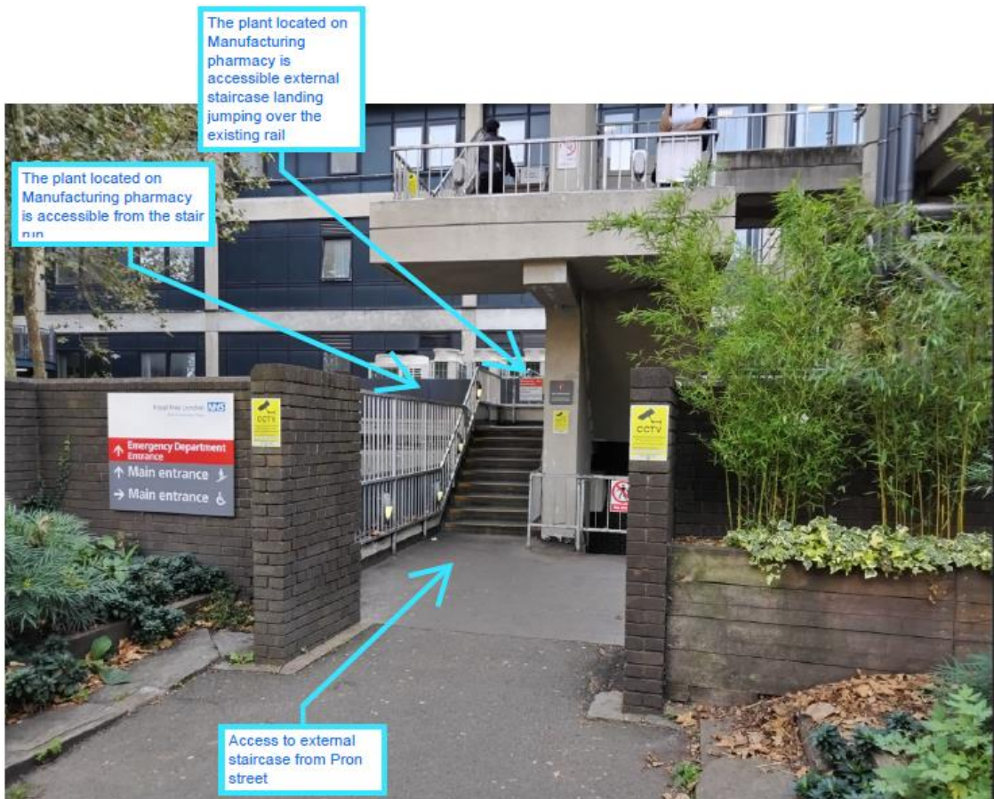
Image 2. Pond Street external concrete stair (Road access placed between Service level and LGF level)
