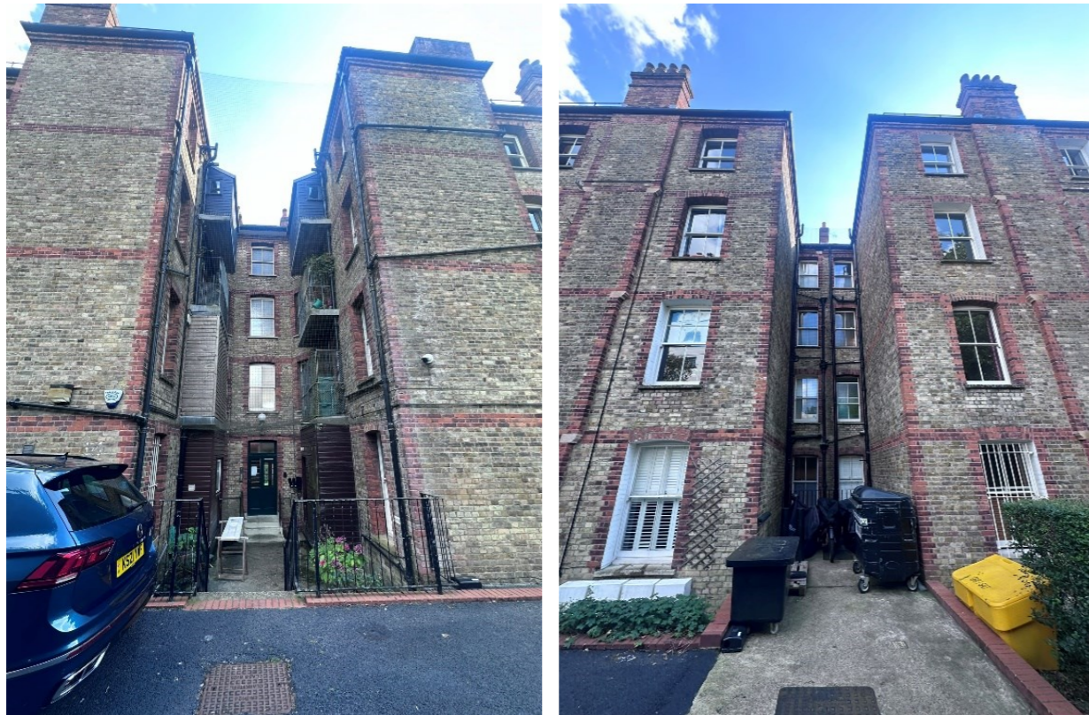
Figures 10 & 11: One of the larger entrance void between the rear outriggers (left) and one of the narrower voids which provides light into the flats (right).
