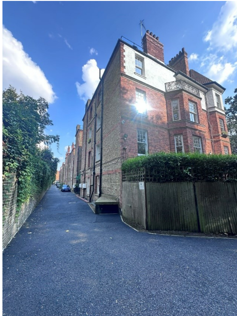
Figure 14: An oblique view looking east along the service road to the rear of the block.
