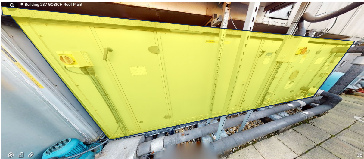
Fig 4. Existing AHU 58 Being Refurbishment
