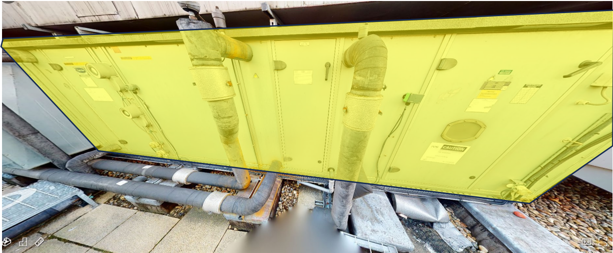
Fig 2. Existing AHU 55 Being Refurbished
