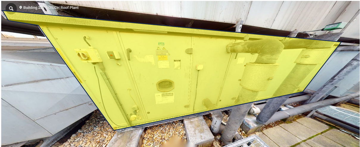
Fig 3. Existing AHU 57 Being Refurbishment
