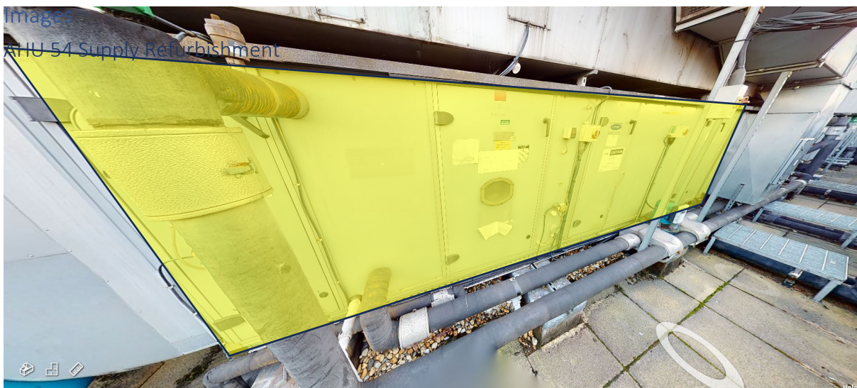
Fig 1. Existing AHU 54 Being Refurbished
