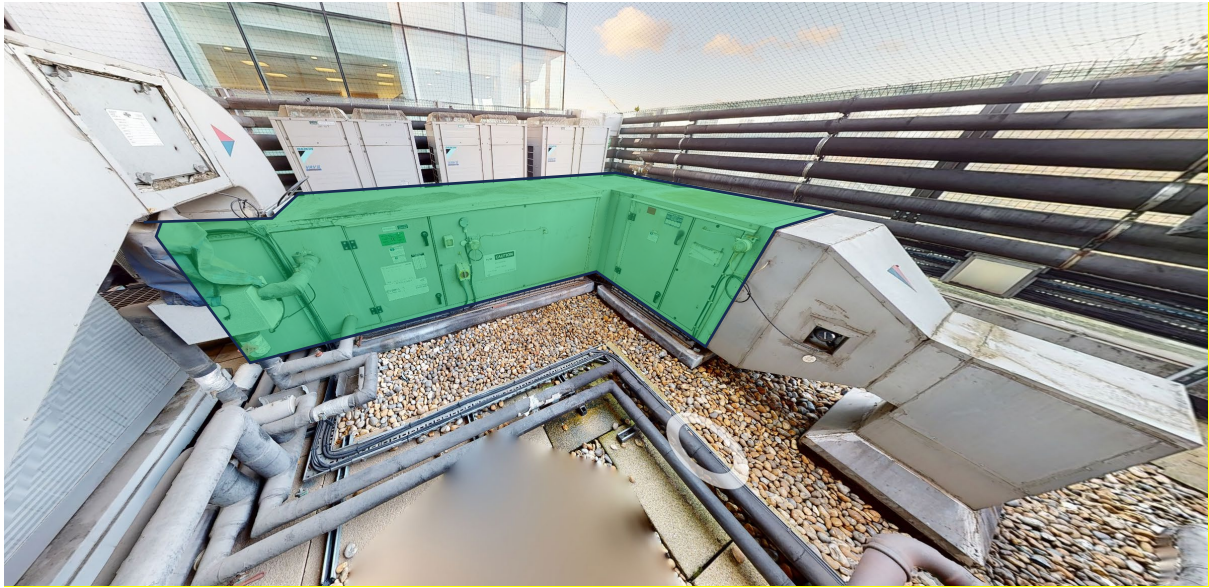
Fig 5. Existing AHU 3 being Replaced
