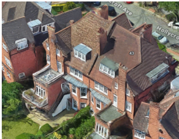
Roof terraces at No. 45 and 43
