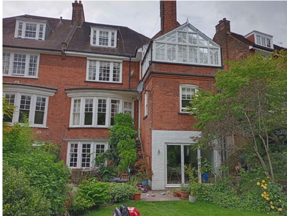
Glazed conservatory above the back addition
