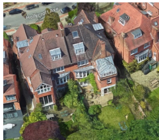
Rear of No 37 and 35
