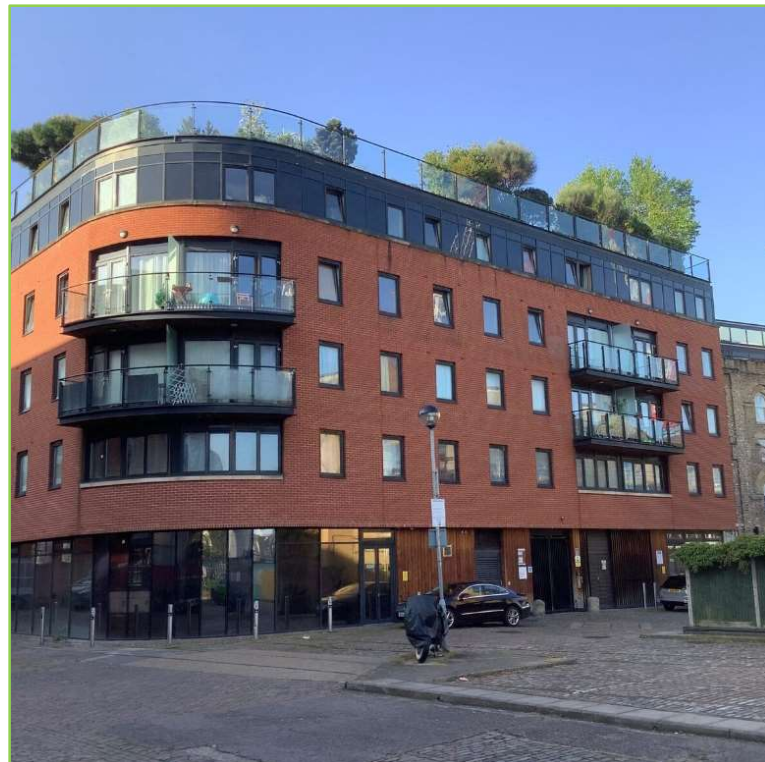
Figure 8.5: North facing Elevation showing masonry, aluminium spandrels and timber cladding at ground level.
