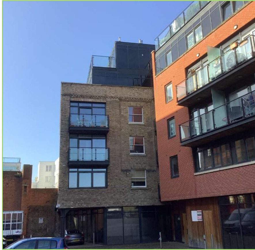
Figure 8.6: North elevation showing masonry and aluminium cladding at upper levels.
