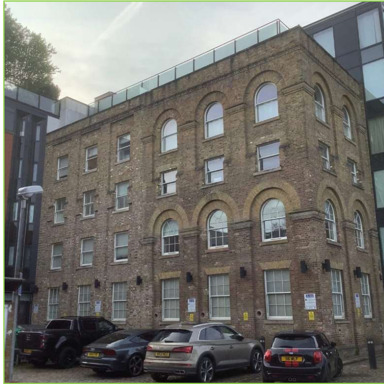
Figure 8.4: North-west Elevation showing original Victorian façade.
