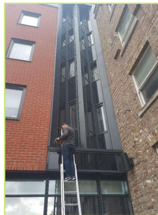
Figure 1.1: Aluminium cladding to be remediated under previous proposals
