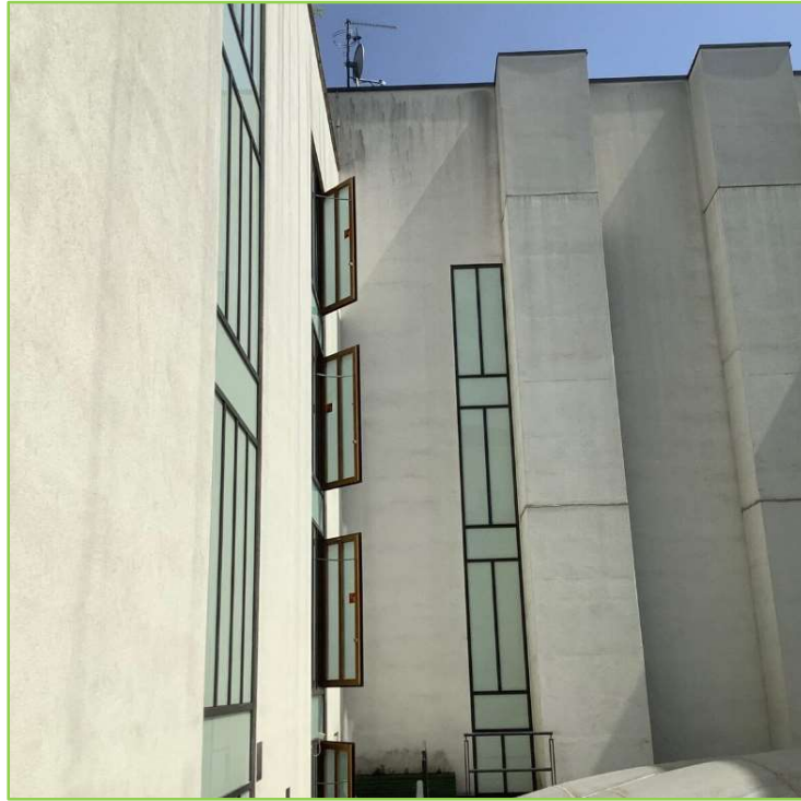
Figure 8.10: Courtyard North-west facing elevation showing the render system.
