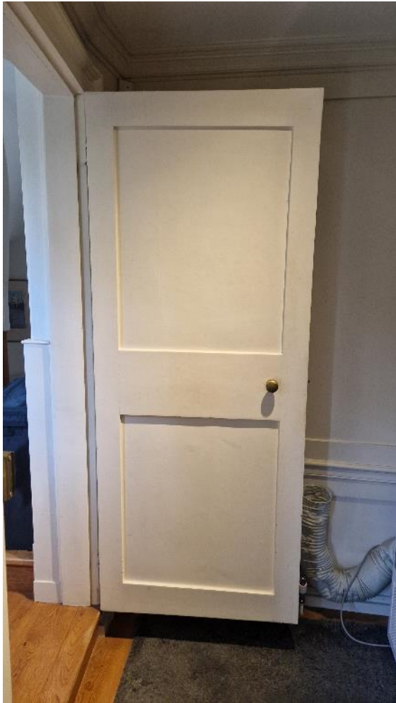
Second floor original door.
