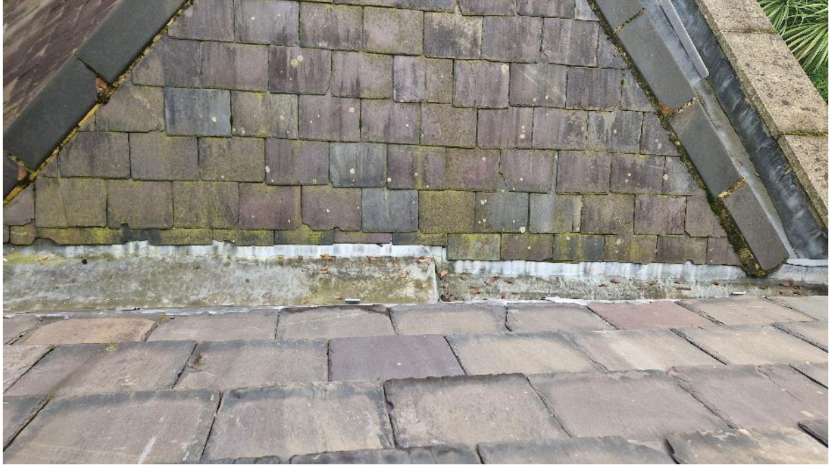
New slate beneath third floor dormer to match slate on roof slope below.
