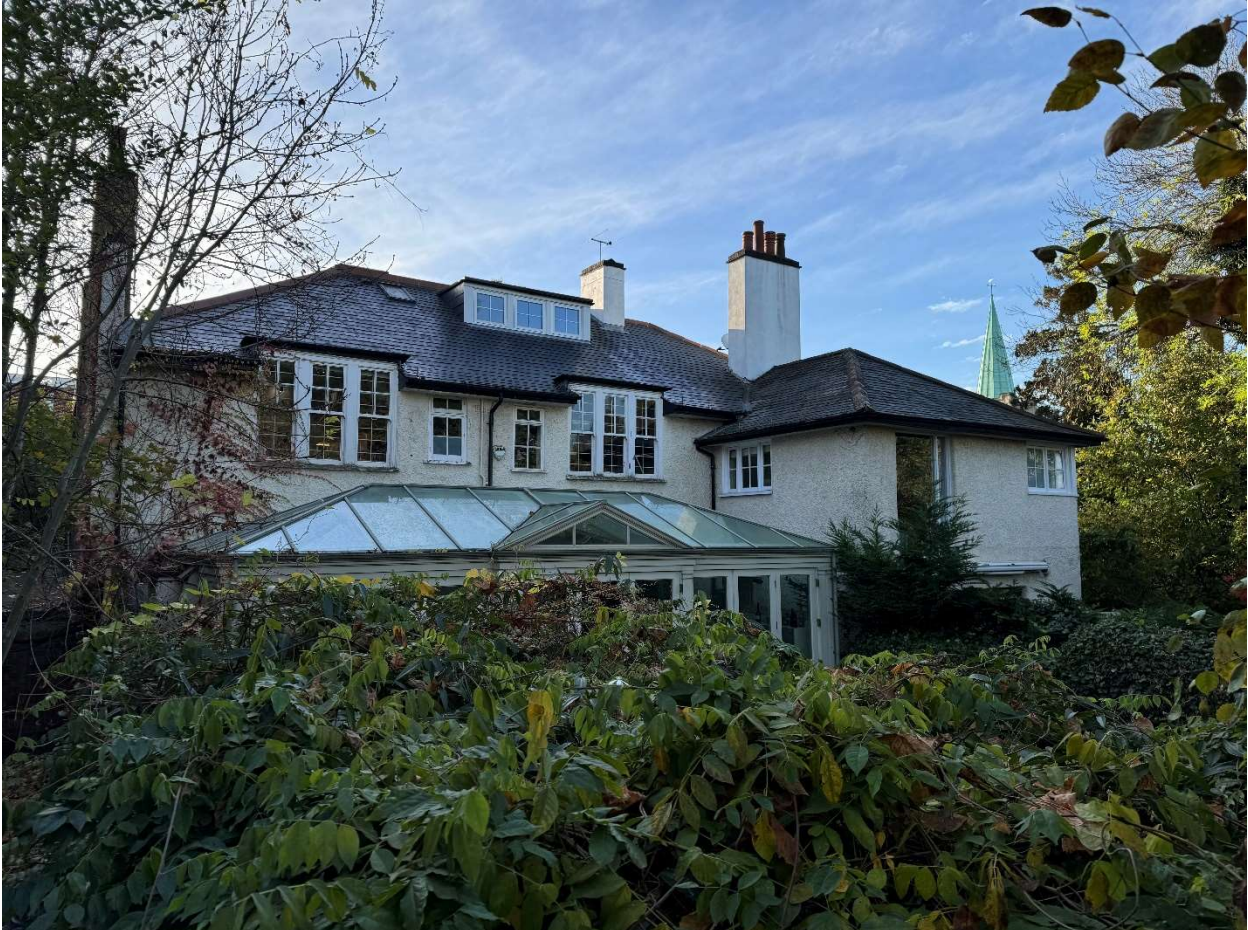
Fig 3.0_Rear elevation view of the as built small dormer in context showing partially the rear of 1 Froggnal Lane and the works granted permission in 2021.
