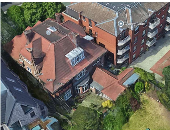
Fig 2.5 Aerial views of the local area showing similar dormers on nearby properties. Top left: Nos. 5 and 7 Bracknell Gardens, part of Bracknell Gate visible to the right of the image. Top right: 17 to 27 Bracknell Gate. Right: flats at 254 Finchley Road
