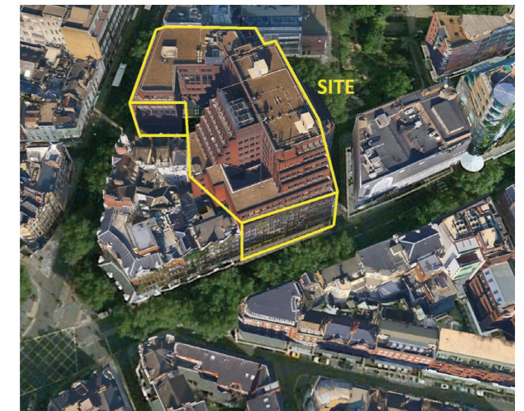
Figure 2.3 Existing building in contextual view
