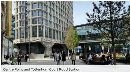
Centre Point and Tottenham Court Road Station
