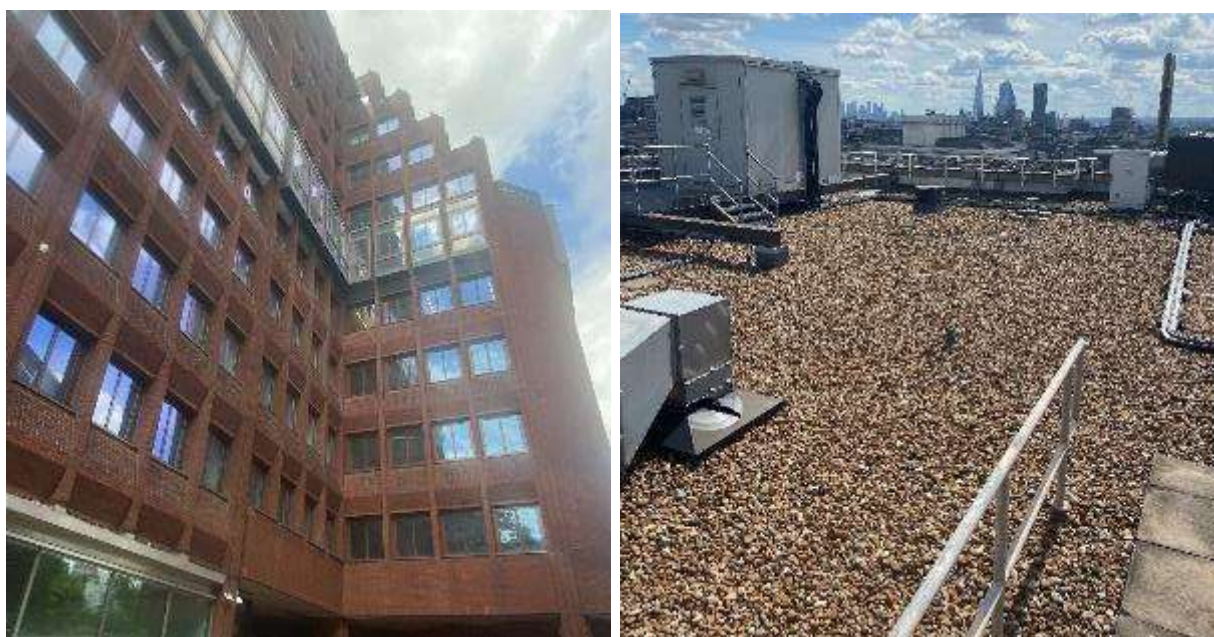
Figure 4.1 Building façade (left) and roof area (right)
