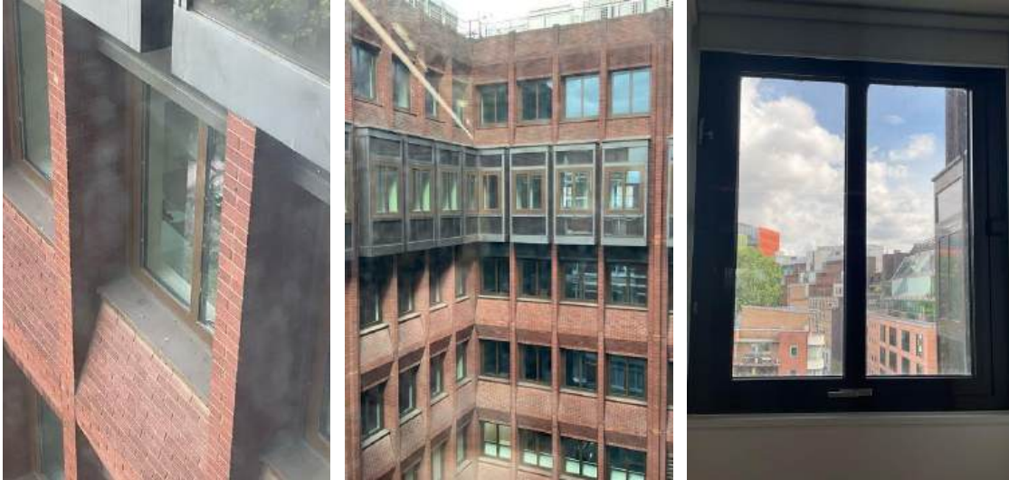
Punched window system (2019), within prefabricated brick facade.
