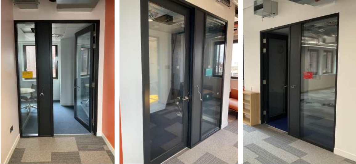
Glazed partitions with doors across 125 Shaftesbury Avenue.
