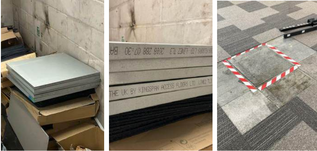
Raised access floor panels underneath various flooring types including carpet tiles.
