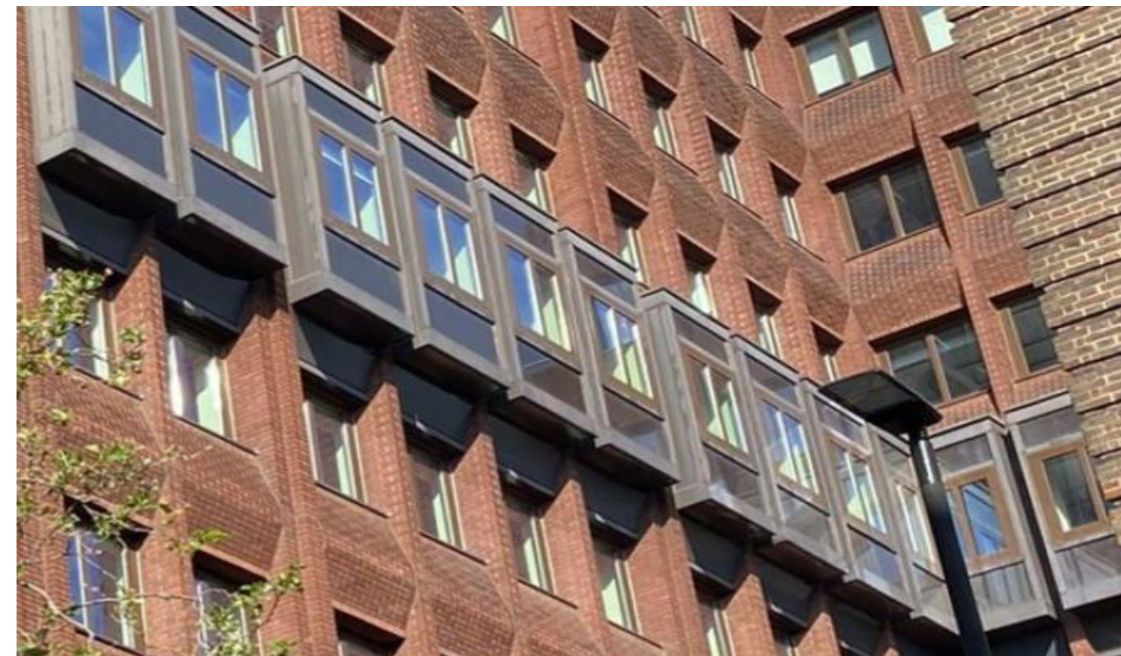
Figure 5.4.2: image to show the ‘bay window’ systems at L05.
