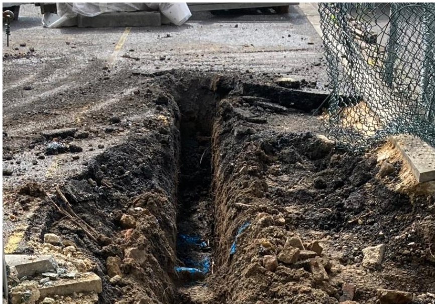
Figure 4: Photograph of tarmacadam carefully broken up with an excavator..
