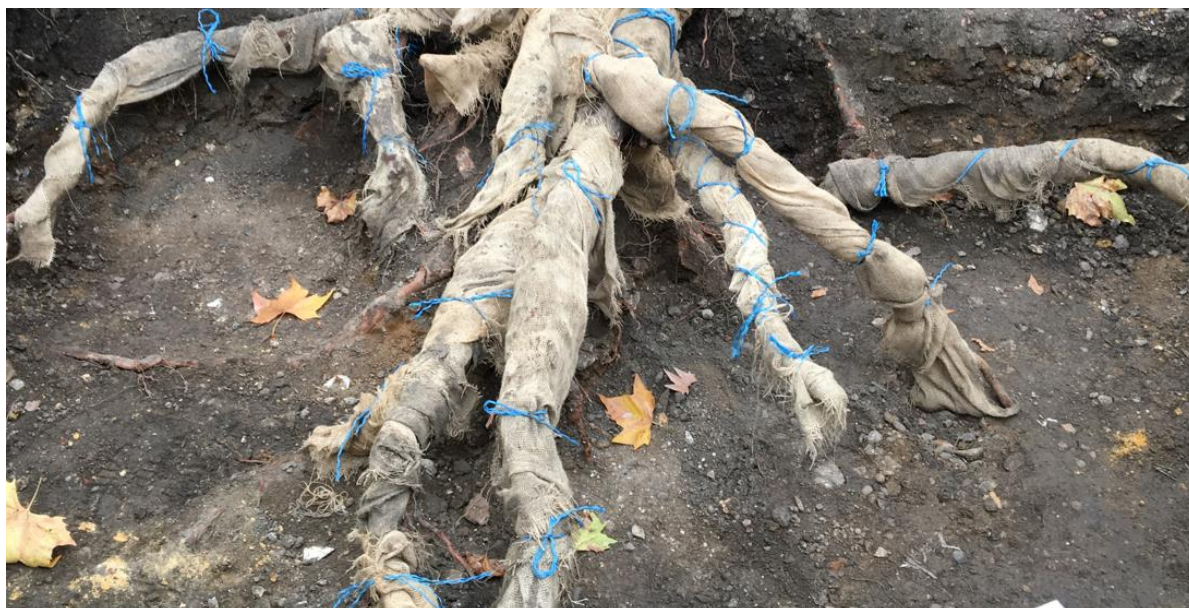
Figure 6: Photograph of successfully protected tree roots.
