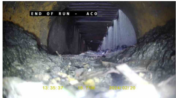
22bee4a0-d2d3-4263-8716-67b4931eaa3c.jpg, 00:02:46, 18.75 m Finish node, manhole, reference: Branch B, Aco
