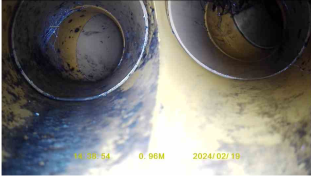
41f72c97-9439-41e7-b088-fc9b7d6f4cbe.jpg, 00:00:17, 0.96 m Junction at 3 o'clock, 100mm dia
