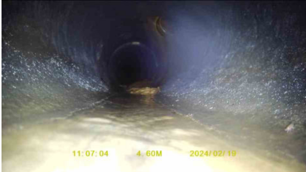
ea7c058d-daaaf-4996-92bc-a8d505804fc6.jpg, 00:00:48, 4.60 m Junction at 2 o'clock, 150mm dia
