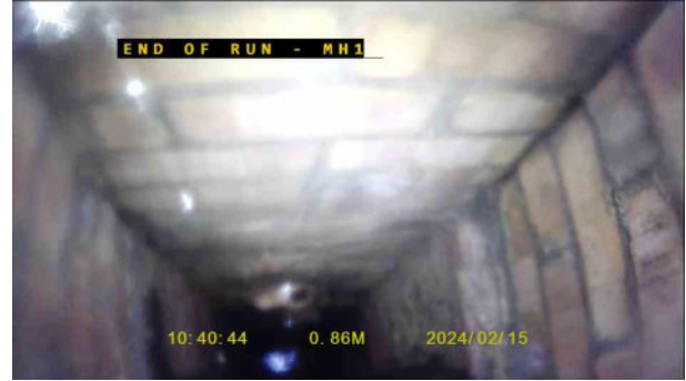
95952fe2-18de-4e60-bd62-6f9d13e47e82.jpg, 00:00:26, 0.86 m Finish node, manhole, reference: MH1
