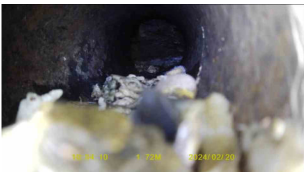
1dff81b8-6366-44e7-99e8-c7580857e882.jpg, 00:01:04, 1.82 m Survey abandoned, Camera unable to pass debris
