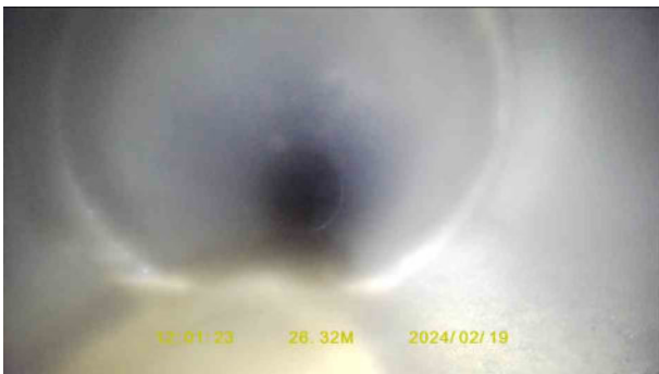
510d2746-6122-4fdc-ac3b-1094141f82cf.jpg, 00:03:03, 26.32 m Joint displaced, large
