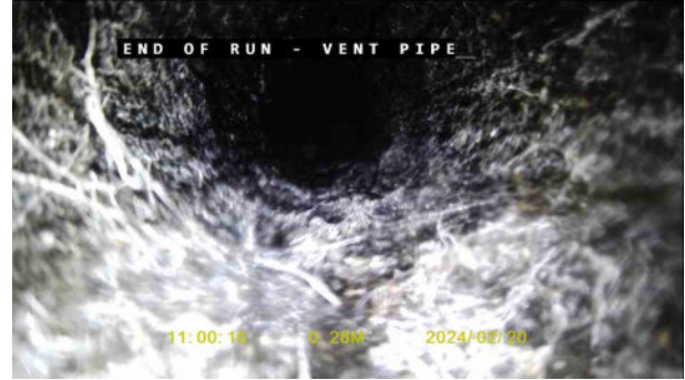
e4e9475f-69f9-45d8-8f38-04630cbdbdc6.jpg, 00:00:19, 0.28 m Finish node, manhole, reference: Branch D, Vent pipe
