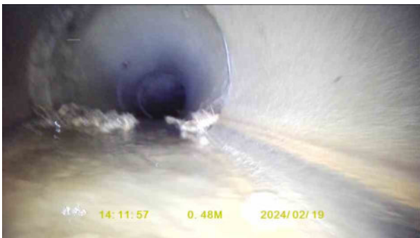
2e89adef-f018-4708-8a79-ba4d7296c35f.jpg, 00:00:12, 0.48 m Roots, mass at joint, 20% cross-sectional area loss, start
