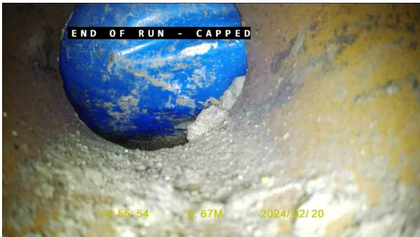
aea4d164-a499-4ccc-8d45-8b070c3022a0.jpg, 00:00:36, 0.67 m Finish node, manhole, reference: Branch B, Capped
