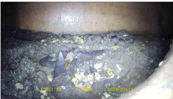
ac05824a-b069-45db-b62a-b17bfb3209f.jpg, 00:00:49, 1.92 m Finish node, manhole, reference: Downstream, Blind Junction
