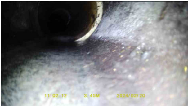
81136733-b89d-435f-a60c-a6bc873af195.jpg, 00:00:46, 3.45 m Joint displaced, medium
