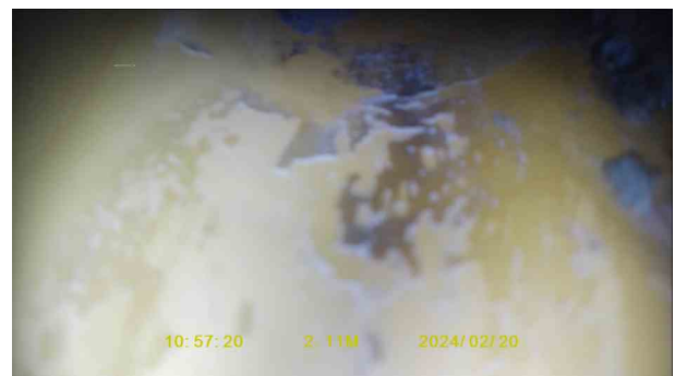
c6a34fc5-3739-4efc-8d4c-76213357c26a.jpg, 00:00:45, 2.11 m Finish node, manhole, reference: Branch C, Rest bend
