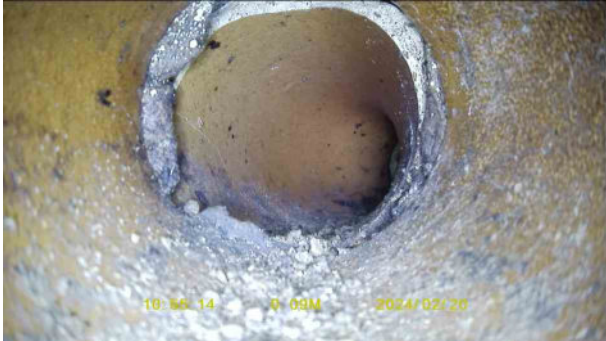
c9179bda-0f0a-4f25-a2db-2d0fef5be277.jpg, 00:00:13, 0.09 m Attached deposits, encrustation at joint from 7 o'clock to 11 o'clock, 15% cross-sectional area loss
