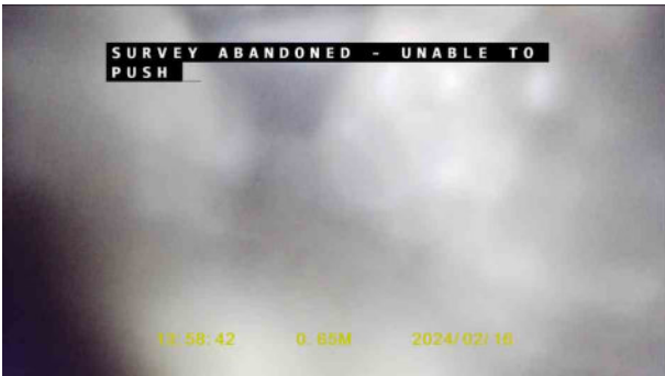
884ca6ea-9957-4bcf-a443-224242517dbb.jpg, 00:00:54, 0.65 m Survey abandoned, Camera unable to push further
