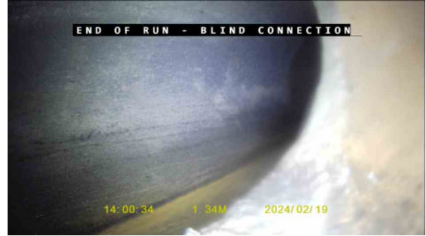
baeccc9c-6492-4e2f-8d1a-066f5c7e8907.jpg, 00:00:29, 1.34 m Finish node, manhole, reference: Downstream, Blind junction
