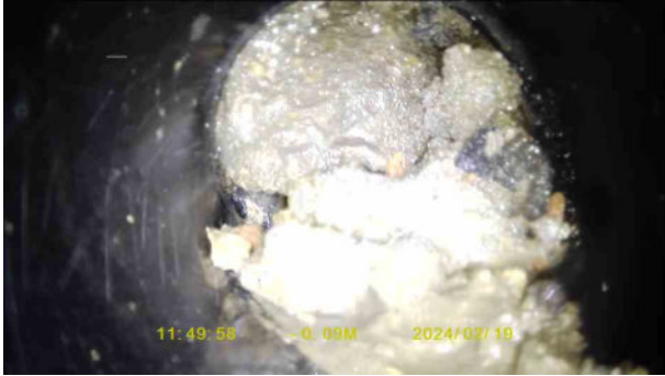
63c30535-253e-4492-9378-4942cecf6de7.jpg, 00:00:10, 0.09 m Settled deposits, coarse, 90% cross-sectional area loss
