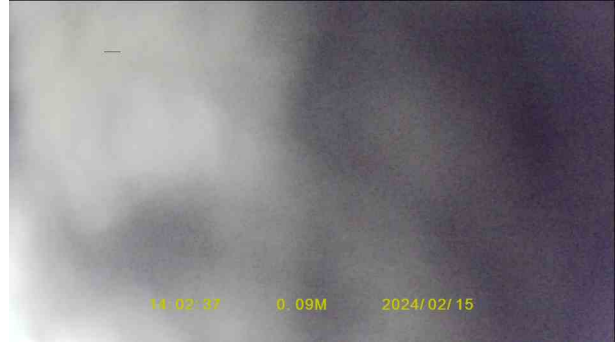
1f425de4-3b74-4eae-be3e-b771f1efb006.jpg, 00:00:43, 0.09 m Loss of vision, silt
