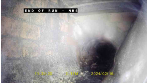
013e92c3-14a1-478c-99df-9637fabe5c0f.jpg, 00:00:59, 2.11 m Finish node, manhole, reference: MH4
