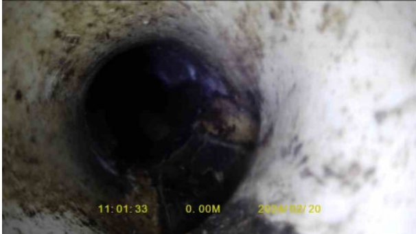
11f4fc9c-ba19-4aad-aca7-5fdd34d41401.jpg, 00:00:08, 0.09 m Junction at 6 o'clock, 100mm dia, Backdrop
