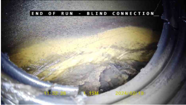
1dea0eed-7dfc-4c31-91b7-6f84a9db01eb.jpg, 00:00:30, 1.15 m Finish node, manhole, reference: Downstream, Blind
