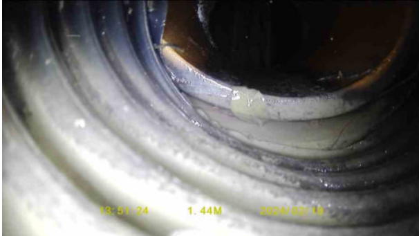
77433b44-5b3a-43c0-89b1-d2bb0d35f7f7.jpg, 00:00:17, 1.44 m Joint displaced, large
