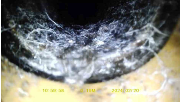
fe861bff-7a5c-4310-831e-8180078c008e.jpg, 00:00:16, 0.19 m Joint displaced, medium
