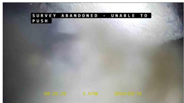
4968c8fc-aa45-4da5-a1a5-ef71bcf6ede3.jpg, 00:01:29, 3.07 m Survey abandoned, Camera unable to pass debris
