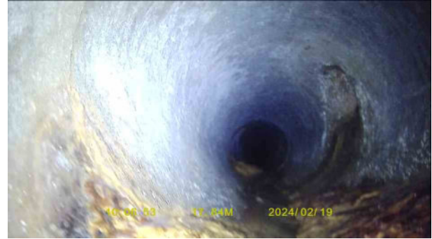
3d116580-de87-4474-93a6-ef091f7398f8.jpg, 00:05:39, 17.84 m Junction at 2 o'clock, 150mm dia
