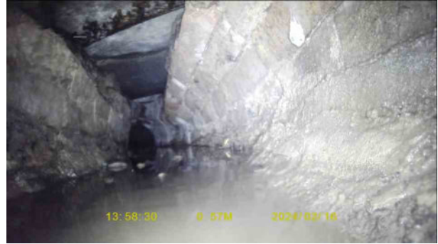
3827b171-7a46-40b8-8e18-5303ecc50257.jpg, 00:00:45, 0.57 m Water level, 20% of the vertical dimension
