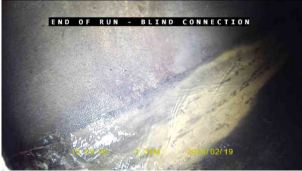
308ae893-16fb-4795-88ba-b6aba68d58e3.jpg, 00:00:30, 1.34 m Finish node, manhole, reference: Downstream, Blind
