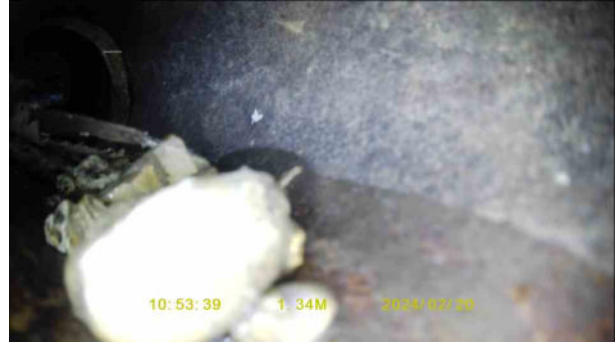
b1ec5c73-cb1b-4989-bafa-742f6e4b7188.jpg, 00:00:39, 1.15 m Settled deposits, fine, 20% cross-sectional area loss
