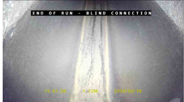
d49db12e-7dcc-40d2-ac65-b00e8a8d0aed.jpg, 00:00:25, 1.72 m Finish node, manhole, reference: Downstream, Blind junction
