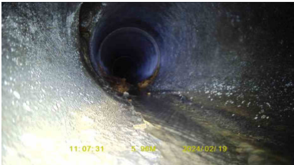
884efa80-ca89-4eb6-874e-267426a38cd7.jpg, 00:01:14, 5.96 m Junction at 10 o'clock, 150mm dia
