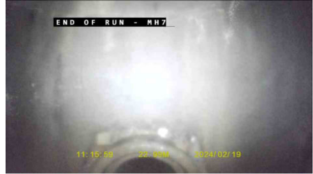
83ddbfa6-0a53-4e15-a2e9-e86f43170ad6.jpg, 00:03:59, 22.99 m Finish node, manhole, reference: MH7
