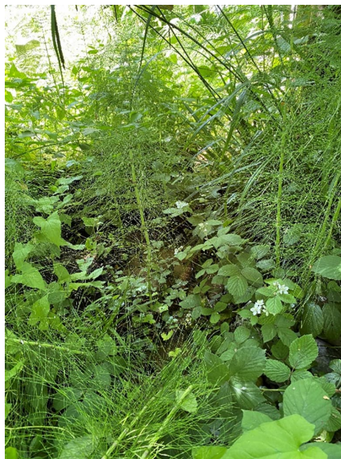
Figure 4 Our investigation identified ponding water, covered by vegetation, in the southwest corner of the west side.
