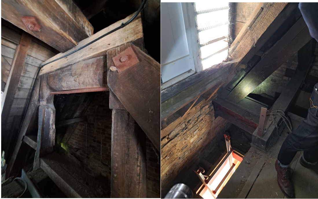
Figure 6. WYE site photos of existing timber truss within central chapel roof
