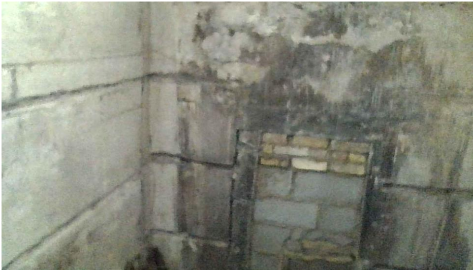
Photograph 23: Da Silva – partial view of interior looking towards the south-east
