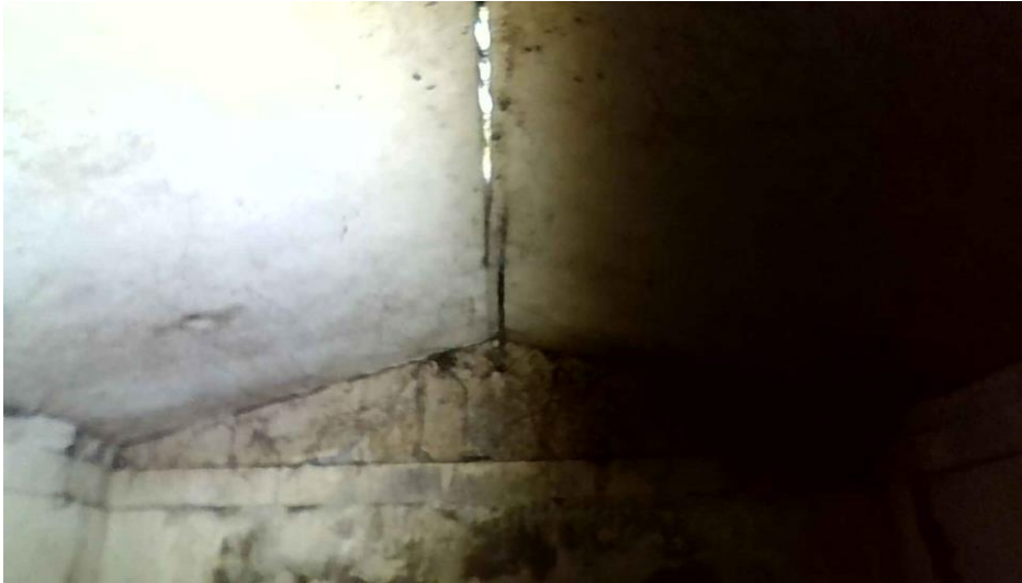
Photograph 22: Da Silva - roof structure
