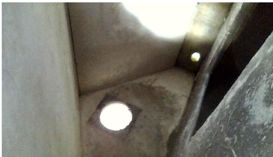
Photograph 13: Rosa – partial view of vault interior (rotated)
