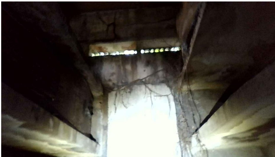
Photograph 19: Morgan – partial view of vault interior
