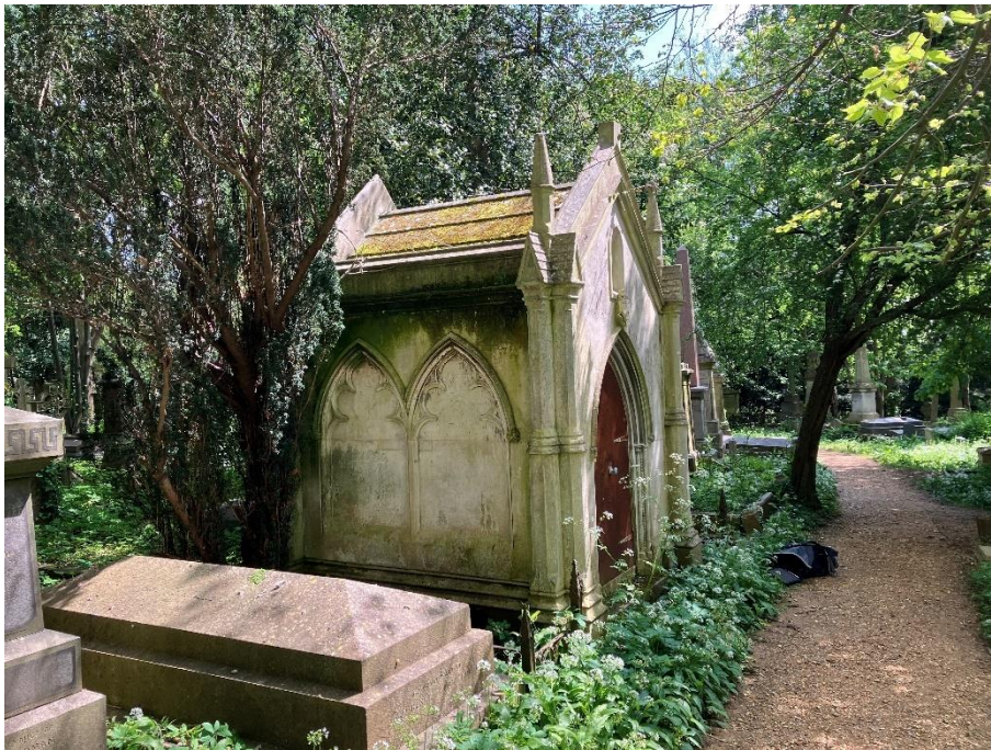
Photograph 17: Foster mausoleum – north elevation
