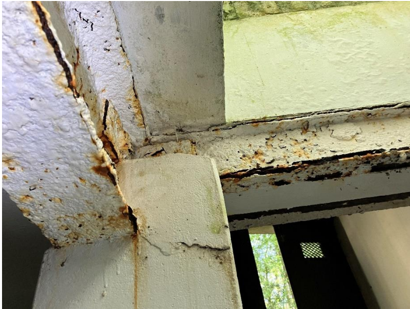
Photograph 14: Otway vault interior – entrance area
