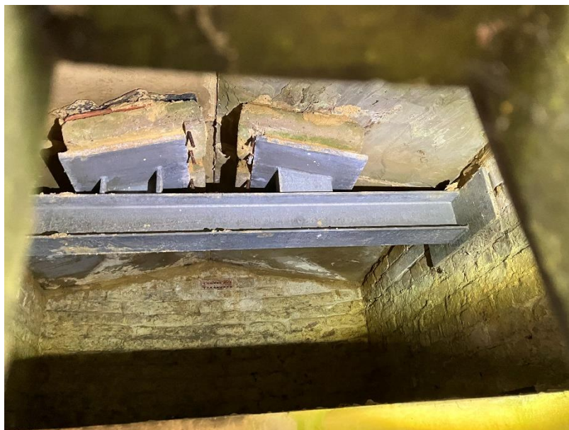
Photograph 9: Hawes vault – previous supplementary supports to roof slabs
