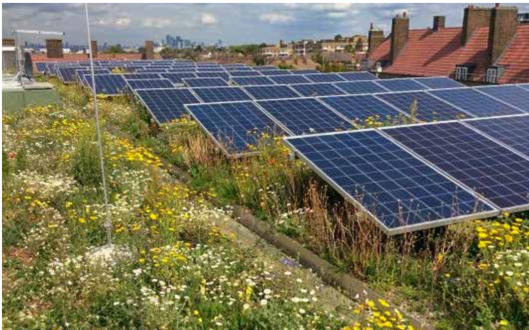
GR2 - Green Roof with PV (Gardener's Building)
