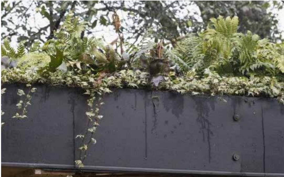
GR1 - Woodland Green Roof (Cafe Building)
