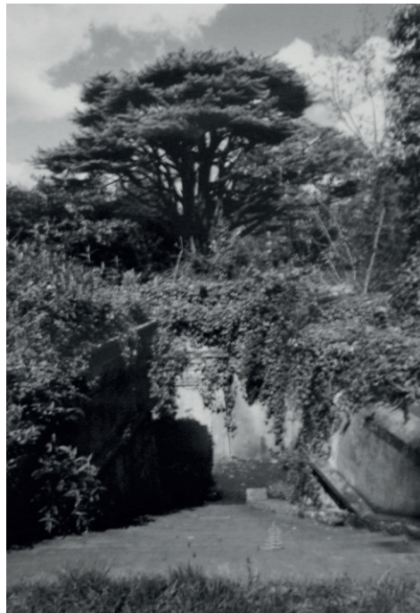
Figure 5.21 Circle of Lebanon, early 1980s (source: ABA)
