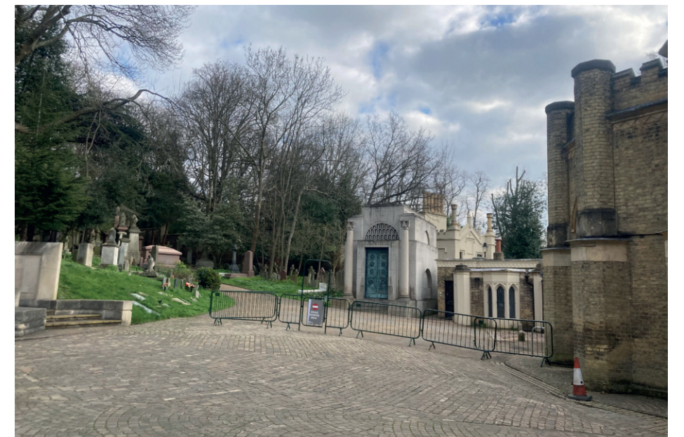
Figure 7.32 Recent photograph of the South Lodge. The Goldhammer Mausoleum, by Craig Hamilton, was built in 2017 and has changed the setting of the lodge
