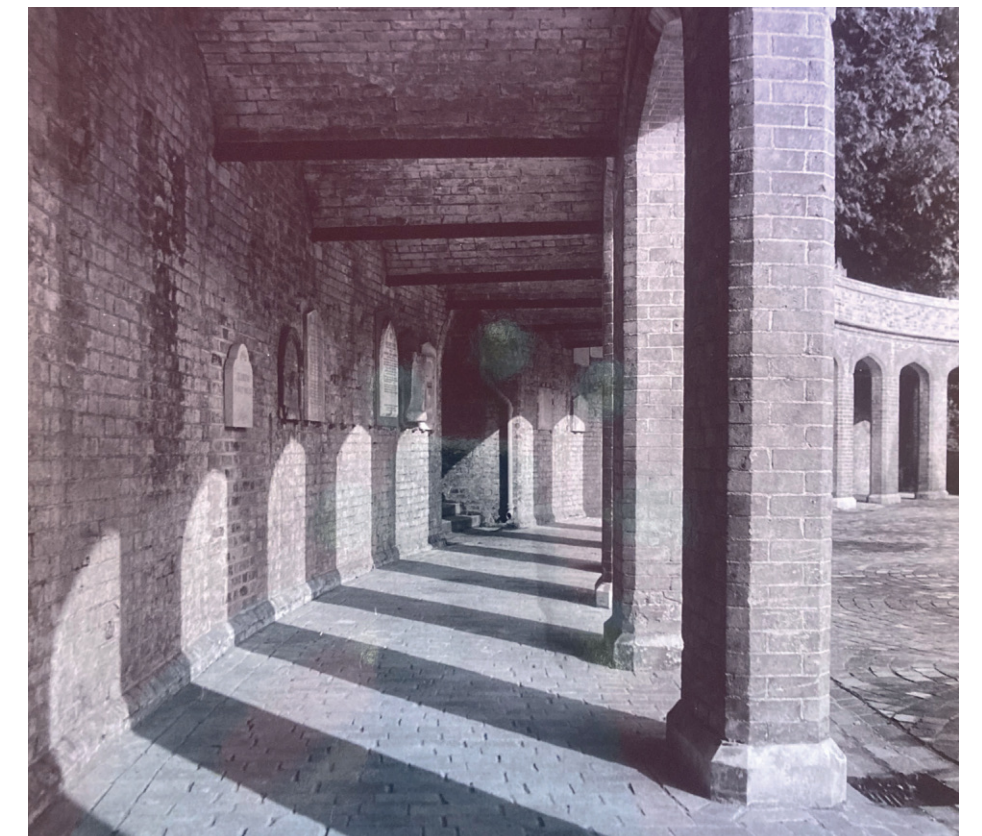
Figure 7.25 Photograph taken by John Gay c.1990 after the Courtyard paving and level change that obscured the base of the arches (source: FoHCT Archives)
