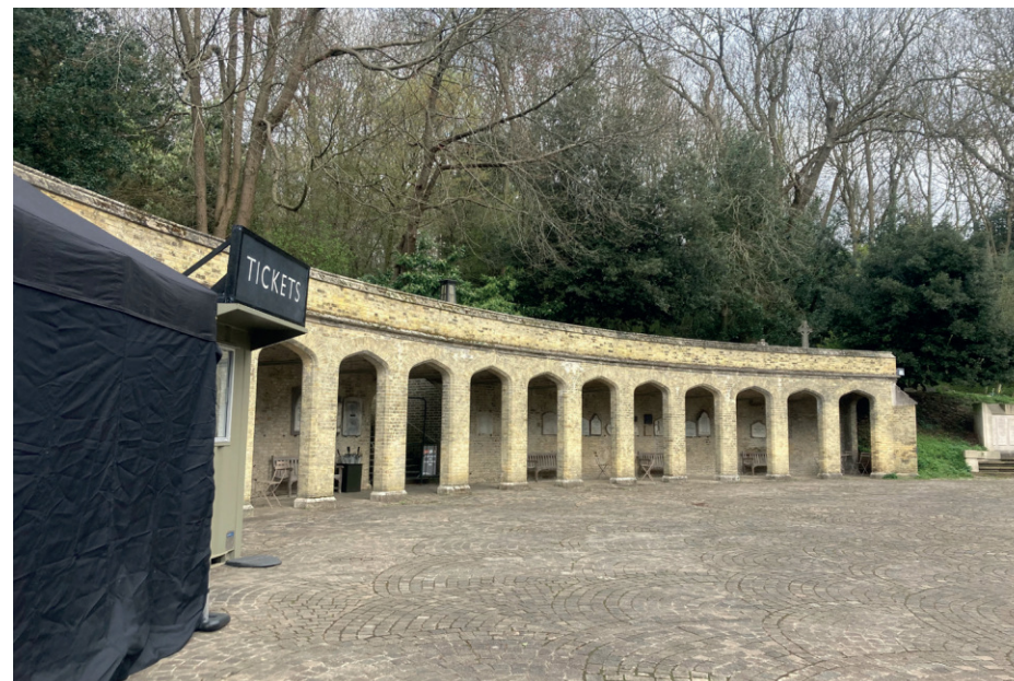
Figure 7.29 Recent photograph of the Colonnade. The temporary ticket office detracts from the Colonnade and its group value with the Chapels, as it obscures part of the Colonnade and interrupts the elliptical form of the Courtyard
