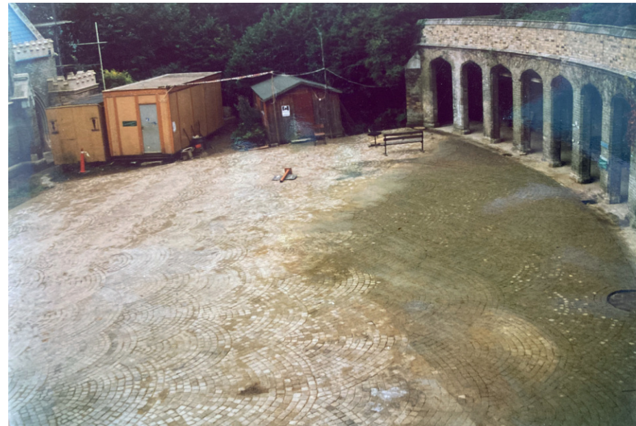
Figure 7.28 Photograph, undated but likely 1970s, showing Colonnade with temporary facilities buildings in the Courtyard (source: FoHCT Archives)
