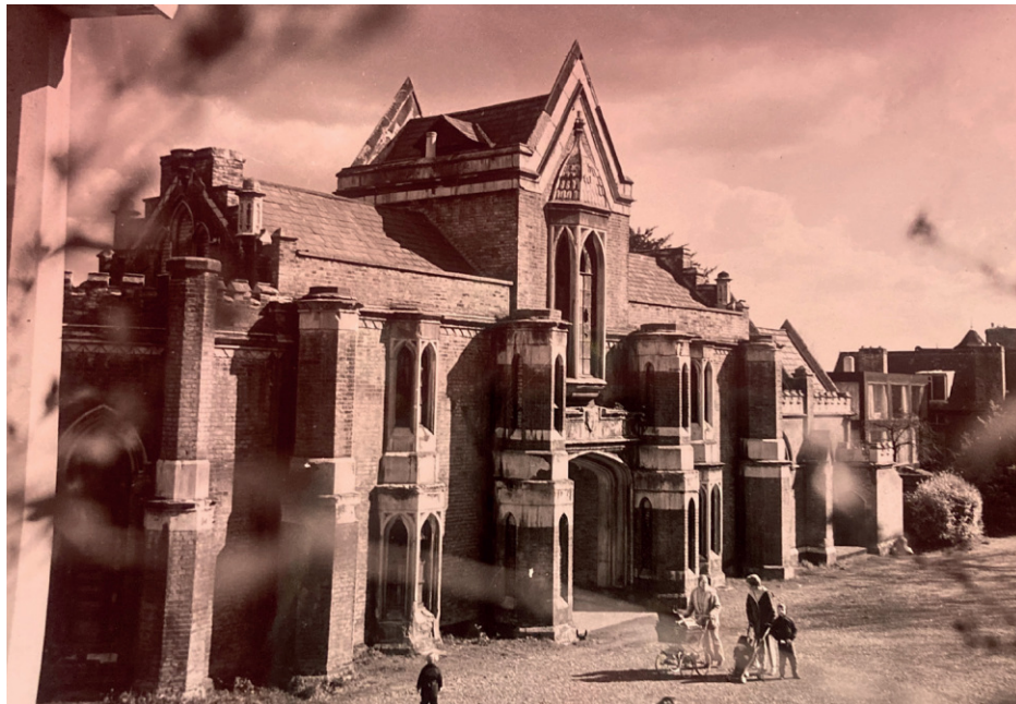
Figure 7.20 Photograph of the Chapel prior to repair works in the 1980s. Undated but likely taken by Gay in the 1970s / '80s (source: FoHCT Archives)
