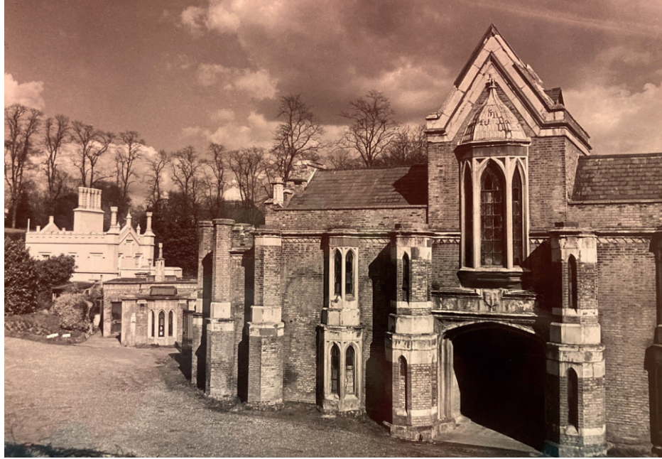
Figure 7.19 Photograph of the Chapel prior to repair works in the 1980s. Undated but likely taken by Gay in the 1970s / '80s (source: FoHCT Archives)
