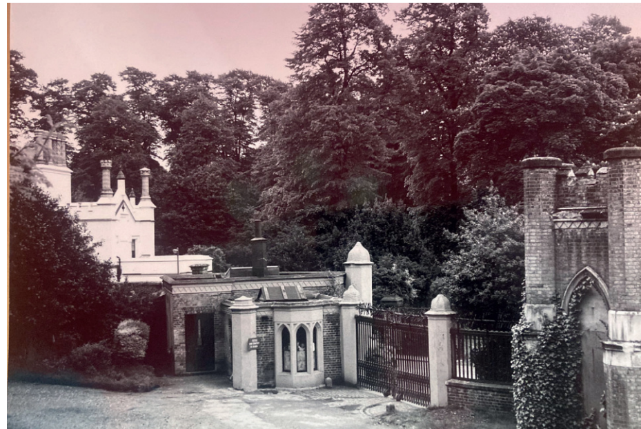
Figure 7.30 Early photograph of the South Lodge, undated but attributed to John Gay, possibly mid-20th century (source: FoHCT Archives)
