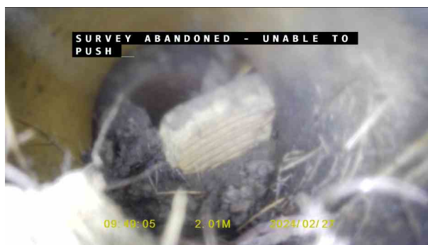
128e637e-cd87-4a72-8c57-c29339dc3771.jpg, 00:00:37, 2.01 m Other obstacles, protruding through wall at joint from 2 o'clock
