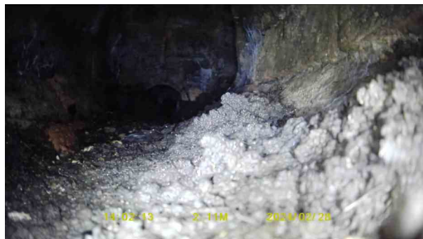
4e7e90c9-6055-4082-9f23-ab097ef6750d.jpg, 00:01:07, 2.11 m Settled deposits, fine, 15% cross-sectional area loss
