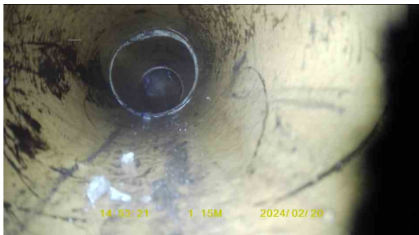
3228861e-72b9-4d30-991e-1a130143f395.jpg, 00:00:21, 1.24 m Broken pipe at joint from 10 o'clock to 2 o'clock
