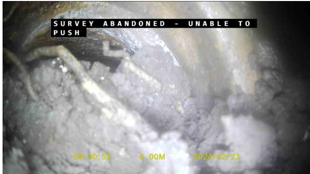
5e992185-dbe2-45d4-85b1-5bdc2159cca4.jpg, 00:00:33, 0.01 m Settled deposits, fine, 85% cross-sectional area loss
