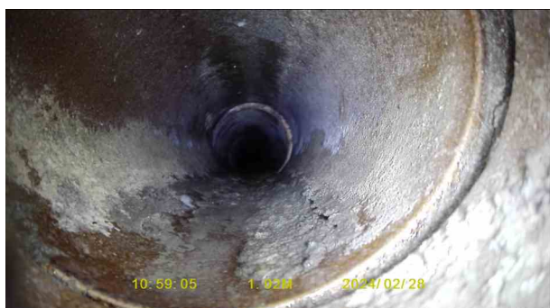
74221590-b06f-4585-a0a0-9d5b4a09d375.jpg, 00:00:43, 1.92 m Joint displaced, medium
