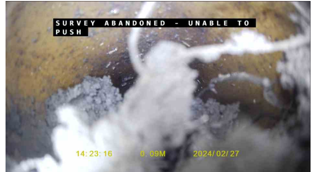
2f514dbb-dea1-4e8c-8afb-a16bb28beaf8.jpg, 00:00:03, 0.19 m Survey abandoned, Camera uable to pass debris
