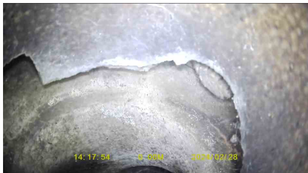
8f4116a7-56b5-4a17-b527-4a1083713b61.jpg, 00:00:07, 0.09 m Joint displaced, large
