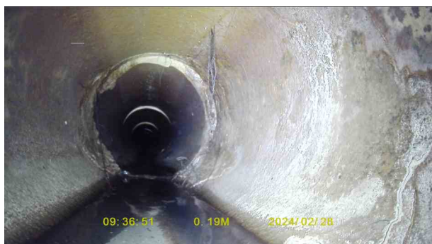
eac5d221-a645-4b00-abdd-63ef763cc8ca.jpg, 00:00:12, 0.19 m Broken pipe at joint from 12 o'clock to 12 o'clock
