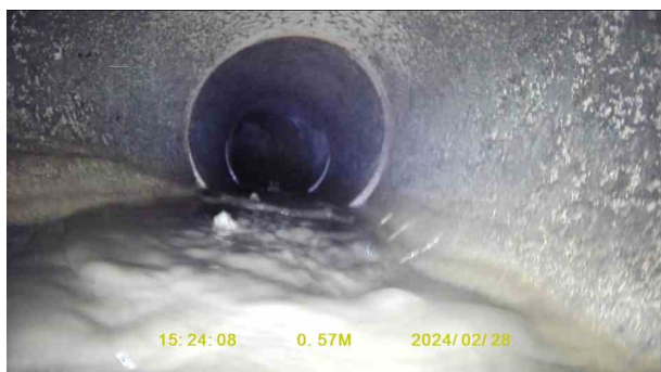
0ddb4aba-a1ce-4d32-bc0a-b2261925cef3.jpg, 00:00:18, 0.57 m Water level, 20% of the vertical dimension
