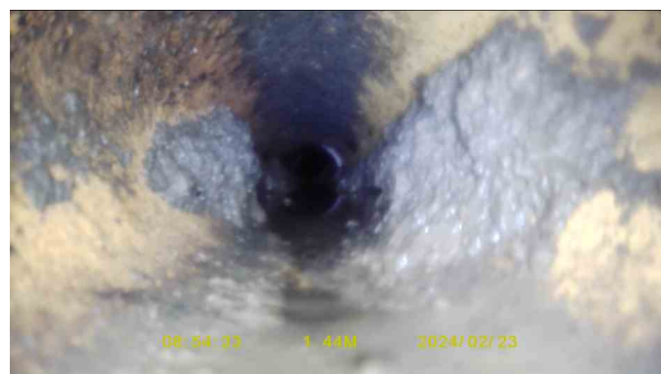
546aff71-f911-49c7-a11a-262728b180b8.jpg, 00:00:38, 1.44 m Attached deposits, encrustation from 2 o'clock to 10 o'clock,
