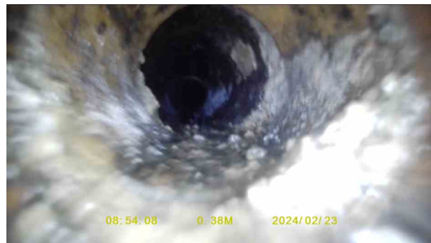
ebf9fdc8-6f5a-468e-87d7-fbdf5e8868cd.jpg, 00:00:24, 0.45 m Joint displaced, medium
