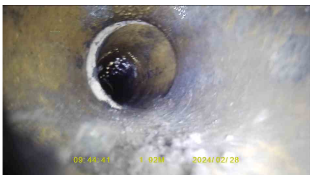
c9997a02-2eea-4949-9ba2-4ea5ffc0ecc9.jpg, 00:00:35, 1.92 m Joint displaced, medium
