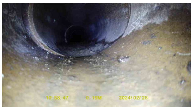
7dc46182-e677-44b7-b370-61bb35cd409f.jpg, 00:00:25, 0.19 m Joint displaced, medium
