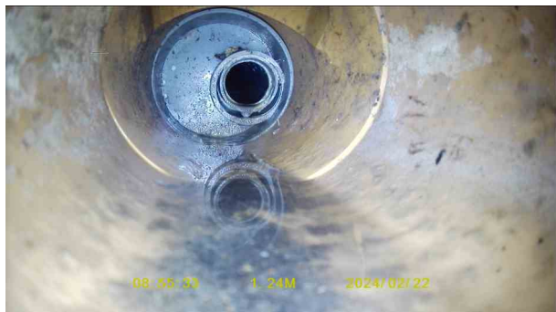
0e13f185-a7d5-4615-9ed7-2c318bcf77ef.jpg, 00:00:25, 1.24 m Junction at 12 o'clock, 100mm dia
