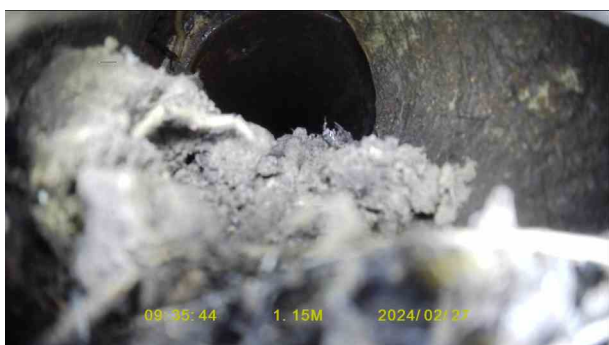
5fc00722-53eb-46b7-a6a4-6f525ee4e3e9.jpg, 00:00:30, 1.15 m Joint displaced, large
