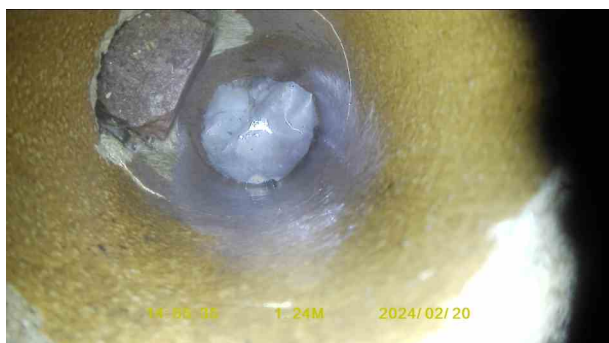
f605058b-0125-4a6f-a3c6-09ad687fb065.jpg, 00:00:45, 1.24 m Hole in drain or sewer from 8 o'clock to 12 o'clock
