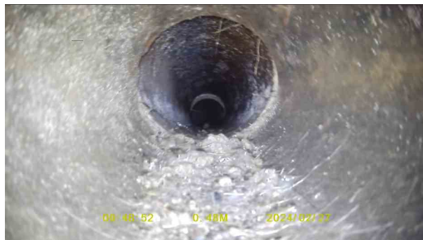
6428489e-c5d8-452f-aa2d-1e93e38ba1ff.jpg, 00:00:25, 0.48 m Roots, fine at joint
