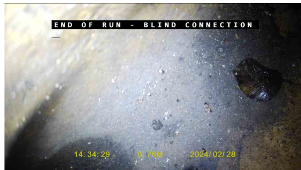
3ad7a6ca-192f-467a-892b-f84485627985.jpg, 00:00:32, 0.76 m Finish node, manhole, reference: Downstream, Blind junction
