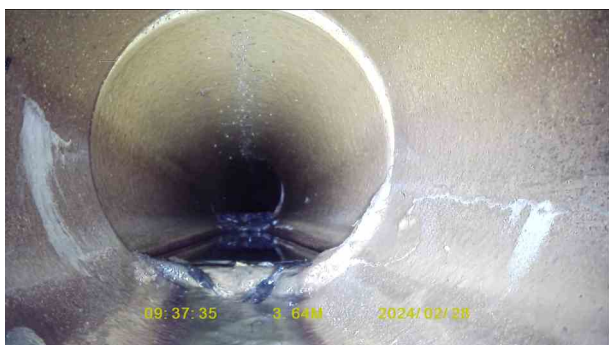
aa3d0a73-6d35-404b-b941-38d745a7c16a.jpg, 00:00:56, 3.64 m Attached deposits, encrustation at joint from 4 o'clock to 7
