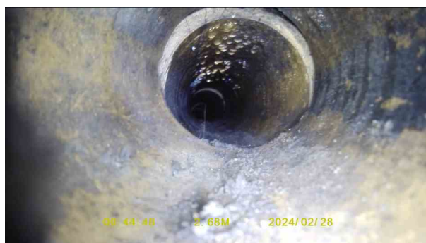
c4737226-e4db-47d8-aabd-d6bc6b44d135.jpg, 00:00:42, 2.68 m Joint displaced, large
