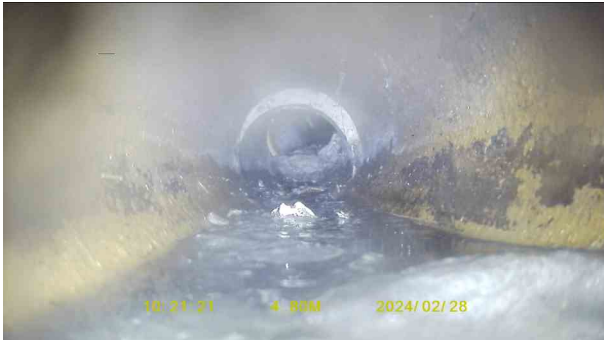
2f091c8d-fe10-47cb-b418-9ad9284ce3d8.jpg, 00:00:12, 0.01 m Settled deposits, fine, 20% cross-sectional area loss
