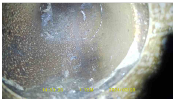
bf2f9e8d-0c9c-493f-a354-865791b645ab.jpg, 00:00:24, 1.72 m Joint displaced, medium, At Rest bend
