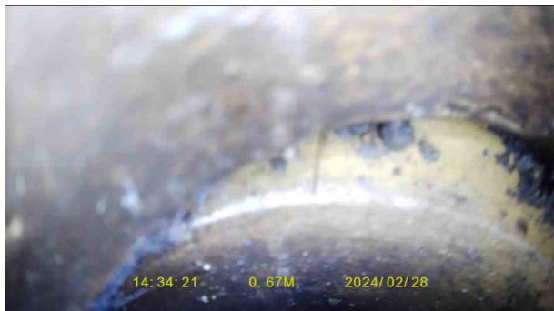
0e816eaf-fb99-41fb-bdc6-a8c9d913ec43.jpg, 00:00:25, 0.67 m Joint displaced, large, Just before blind junction
