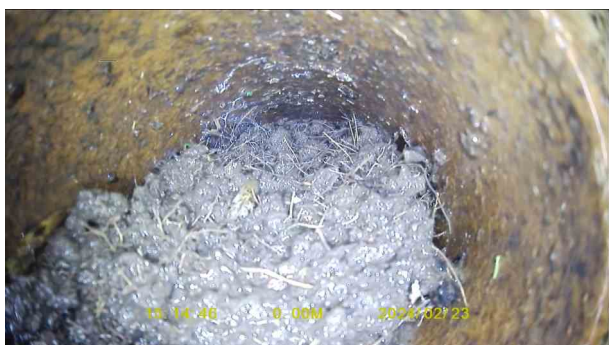
71eb3025-57c9-4381-b2e4-7fcef2da41a.jpg, 00:00:20, 0.01 m Survey abandoned, Camera unable to pass mass
