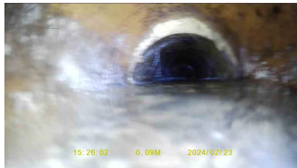
6ee41bfa-2c6b-4ab7-b077-affa711075f3.jpg, 00:00:13, 0.09 m Joint displaced, large
