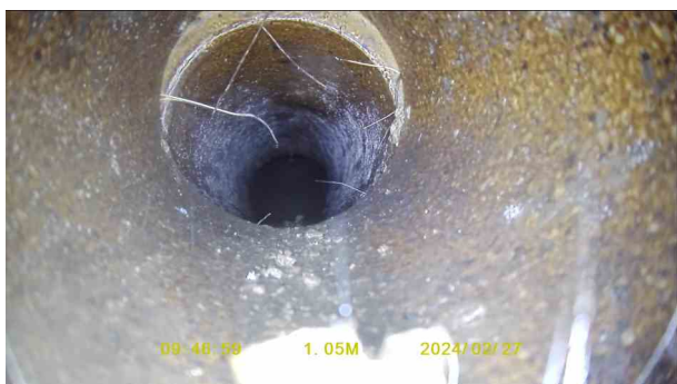
7d1c609c-6dcd-4a59-b297-f576f69144cf.jpg, 00:00:32, 1.15 m Roots, fine at joint
