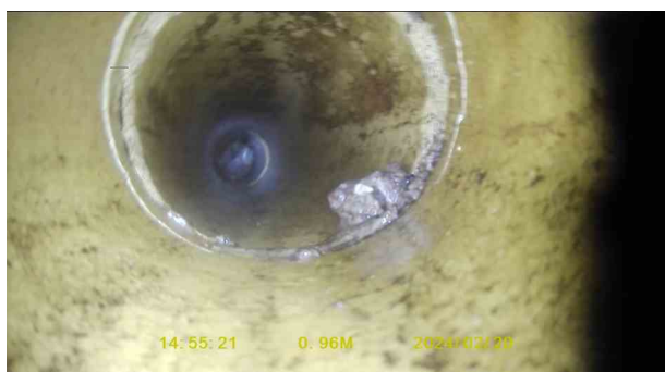
13642834-7cb8-4aee-88aa-db777bf3f6f5.jpg, 00:00:30, 0.96 m Fracture, circumferential at joint from 7 o'clock to 4 o'clock
