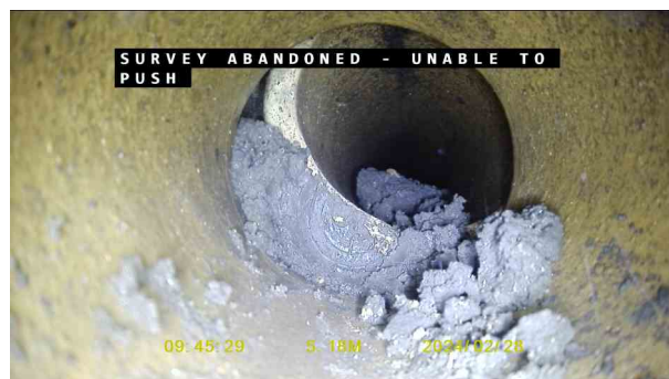
4b256e0b-1001-45ce-892c-500a0a41122e.jpg, 00:01:08, 5.18 m Survey abandoned, Camera unable to pass JDL
