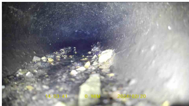
3669f89d-96e6-42b7-ada0-360456e60483.jpg, 00:00:22, 0.36 m Settled deposits, fine, 25% cross-sectional area loss, start
