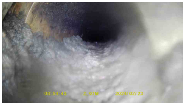
5bde52ec-05ae-43d4-9be4-8f5e391d23ae.jpg, 00:00:58, 2.97 m Joint displaced, large
