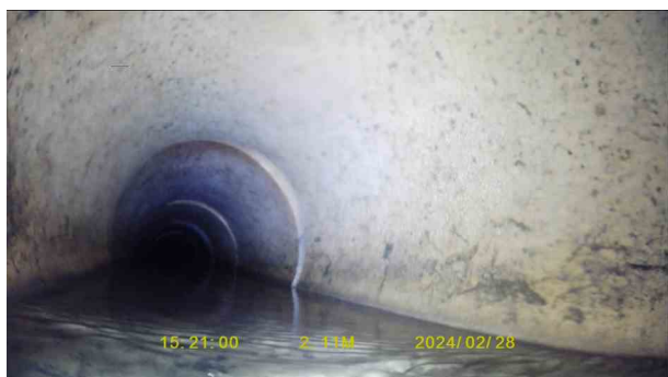
6ab524fc-49ec-4ec2-b2e6-076abcf96f41.jpg, 00:00:51, 2.11 m Attached deposits, encrustation from 5 o'clock to 7 o'clock, 20% cross-sectional area loss, start
