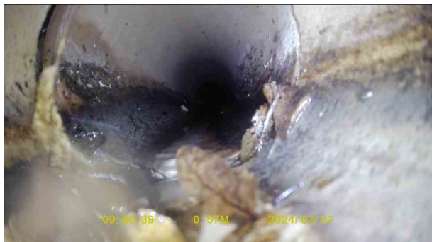
4e79300f-1ec5-462c-bc77-3e3706d264e5.jpg, 00:00:21, 0.57 m Joint displaced, medium
