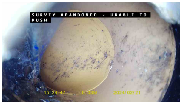
ddf39acd-cb91-4bac-8121-3f3a5a6882cd.jpg, 00:00:19, 0.09 m Survey abandoned, Camera unable to pass obstruction
