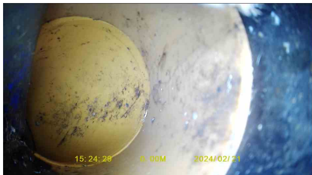
e627b005-8a7f-405c-83c2-5149833629f4.jpg, 00:00:07, 0.01 m Other obstacles at joint from 8 o'clock to 11 o'clock, 20%
