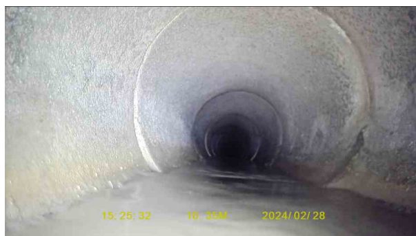
f8c42220-fb22-455e-a4fb-0b886136aeeb.jpg, 00:01:42, 10.35 m Water level, 20% of the vertical dimension
