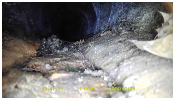
bd31d3c1-edec-4323-81ff-9816ca29f87c.jpg, 00:00:22, 1.05 m Displaced bricks, single brick false from 5 o'clock to 7 o'clock, start
