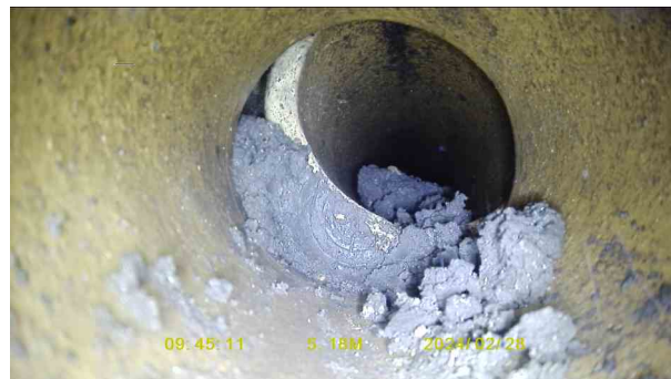
0b86901a-c5d3-4acb-8172-bbdfff70f9fe.jpg, 00:01:05, 5.18 m Open joint, large
