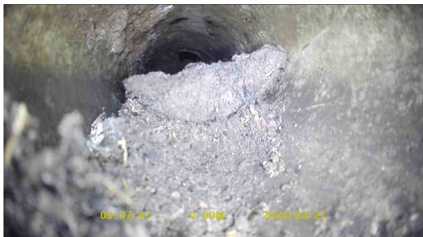
cbedb70e-1abb-451e-8590-e41d940529c4.jpg, 00:00:17, 0.01 m Settled deposits, fine, 60% cross-sectional area loss
