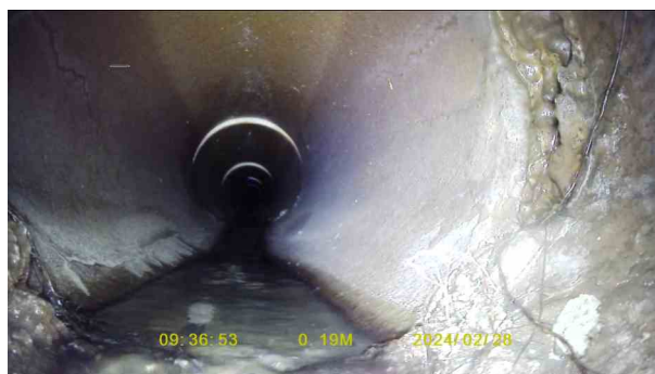
8a625499-afd1-44cf-a783-82c76817da85.jpg, 00:00:15, 0.19 m Roots, fine at joint
