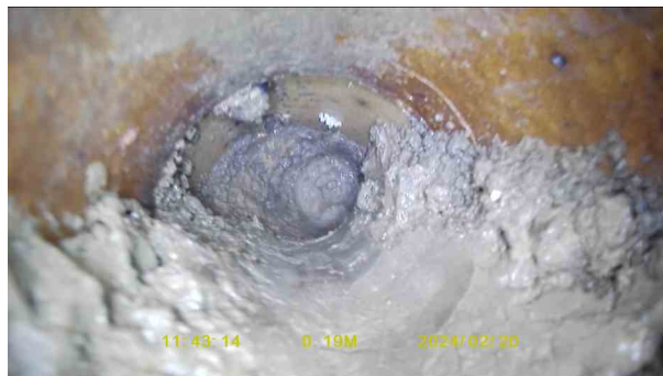
b482562e-aadc-44c9-9627-b559e6baef05.jpg, 00:00:25, 0.19 m Crack, circumferential at joint from 12 o'clock to 3 o'clock
