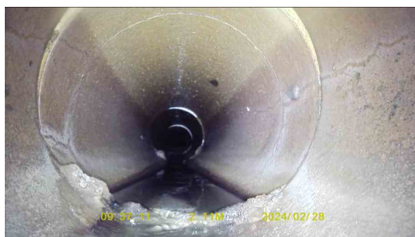
fb6a5d86-324c-4a40-b619-137fa61fdd51.jpg, 00:00:33, 2.11 m Attached deposits, encrustation at joint from 5 o'clock to 7 o'clock
