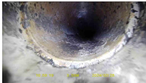
ef59b3cd-38a9-45ec-a904-49bcb886006c.jpg, 00:00:57, 3.55 m Joint displaced, medium
