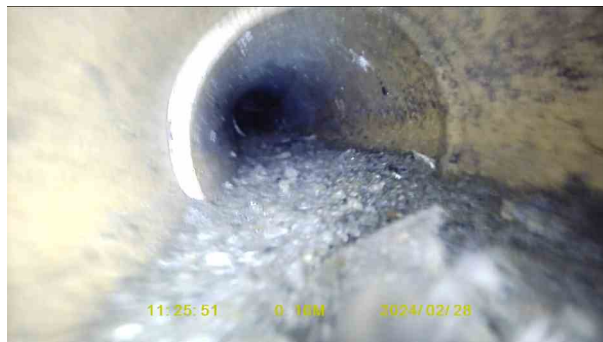
a5bb8a15-44ea-4299-932a-bd0cf48bb56d.jpg, 00:00:15, 0.16 m Joint displaced, medium
