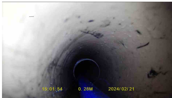
cf5a5643-07b3-4b04-872f-a1eb41d5d638.jpg, 00:00:15, 0.28 m Other obstacles from 5 o'clock to 7 o'clock, 25%
