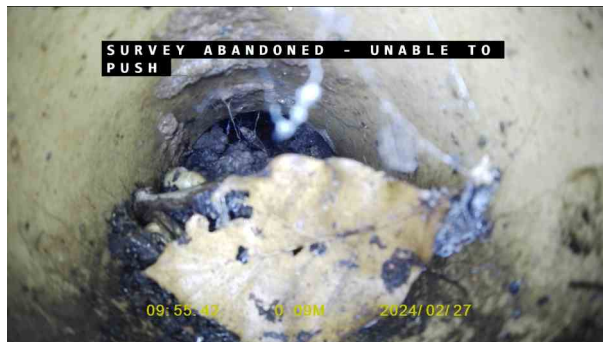
c41e8986-3fa4-49c2-81e9-a6df2293c256.jpg, 00:00:23, 0.09 m Survey abandoned, Camera unable to pass debris/Possibly
