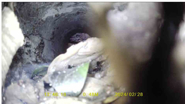
e6148df6-479e-471a-969a-ecfed70f1506.jpg, 00:00:19, 0.48 m Settled deposits, fine, 30% cross-sectional area loss, start
