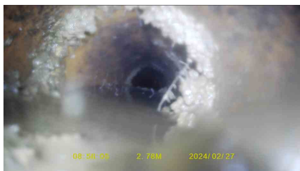
476f513a-e145-4712-aba0-0c70bedffb96.jpg, 00:00:48, 2.78 m Roots, fine at joint
