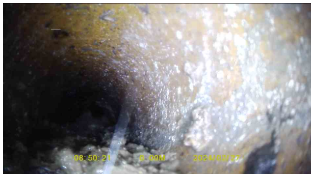
30e5672e-07dd-453b-9b6f-79ff09f2d35b.jpg, 00:00:10, 0.01 m Settled deposits, fine, 25% cross-sectional area loss, start
