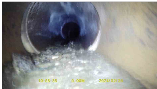
59989cb7-882d-4cad-8231-0d4c84c6b221.jpg, 00:00:13, 0.09 m Joint displaced, medium
