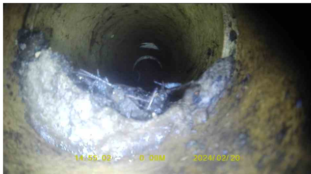
54fe3fcb-6687-4a68-904e-116084061c3e.jpg, 00:00:12, 0.09 m Joint displaced, medium
