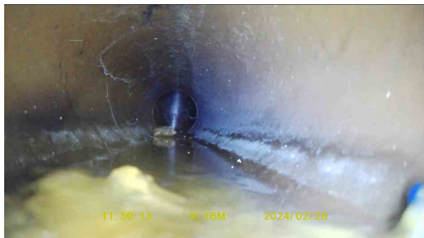
7f1e18e7-65cc-4e0b-8342-9da276334a4a.jpg, 00:00:13, 0.01 m Settled deposits, fine, 15% cross-sectional area loss
