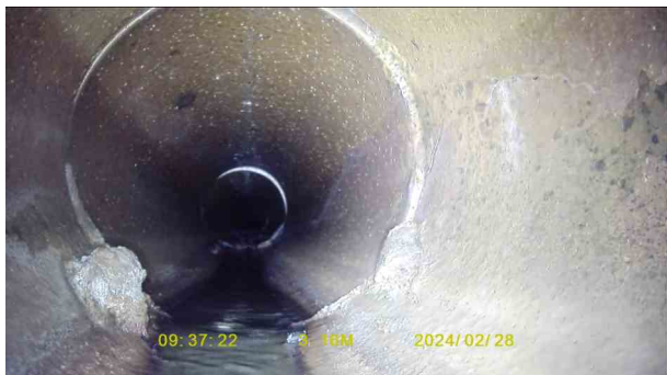
f4ffd01f-f25a-4200-a2ab-bb432de9a09f.jpg, 00:00:44, 3.16 m Attached deposits, encrustation at joint from 7 o'clock to 8 o'clock, 15% cross-sectional area loss
