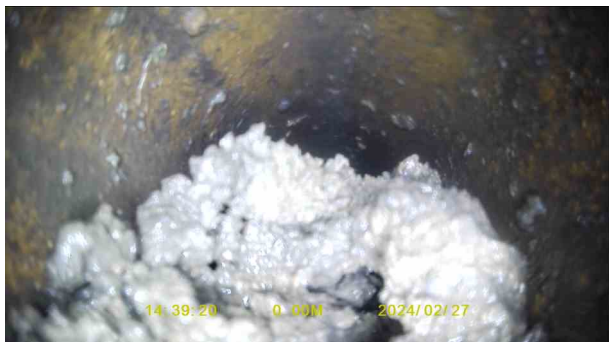
24f01336-08e8-4b56-bea3-61ae8406c6f1.jpg, 00:00:12, 0.01 m Settled deposits, fine, 75% cross-sectional area loss
