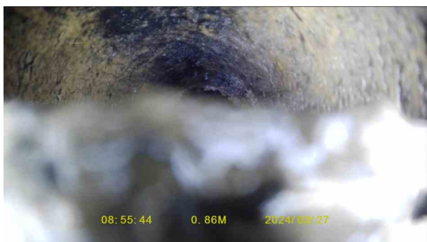
f2d62bf4-19ff-4ca9-a24b-e97f0c05f77f.jpg, 00:00:27, 0.86 m Settled deposits, fine, 60% cross-sectional area loss, start
