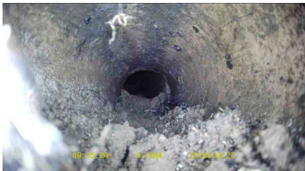
cb26f994-a3e6-44ee-abe5-ce6e57f387f1.jpg, 00:00:10, 0.01 m Settled deposits, fine, 25% cross-sectional area loss, start
