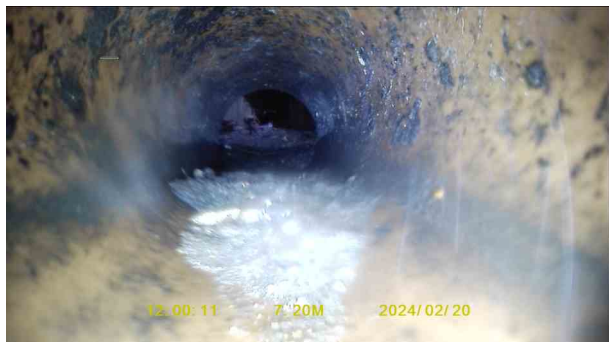
bc17b186-e1f3-43d7-ba4f-f5fee1ec2c81.jpg, 00:01:22, 7.20 m Settled deposits, fine, 20% cross-sectional area loss
