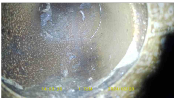
8c6600a3-79e4-415c-8466-92a3d7a63583.jpg, 00:00:24, 1.72 m Fracture, circumferential from 2 o'clock to 6 o'clock, In Rest
