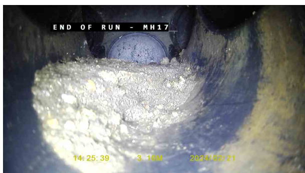
4e2be326-f855-49ca-b772-5fb7d57c2b38.jpg, 00:01:09, 3.16 m Settled deposits, fine, 30% cross-sectional area loss, In
