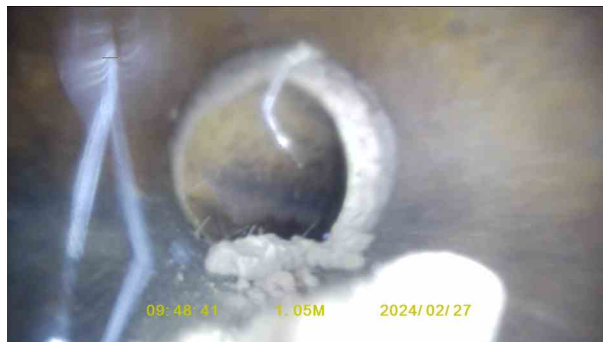
c7163da9-020a-44f5-8fdf-cd71268ab28b.jpg, 00:00:22, 1.05 m Joint displaced, large
