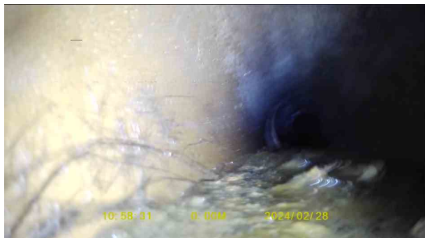
132c5efe-8fb1-4b9e-a824-f4bad41f3c98.jpg, 00:00:13, 0.01 m Settled deposits, fine, 25% cross-sectional area loss, start
