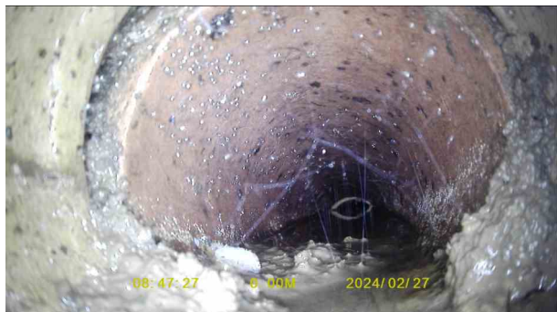
f0e37fa7-f24e-4e91-8c76-1c56c7c197a6.jpg, 00:00:12, 0.01 m Joint displaced, large
