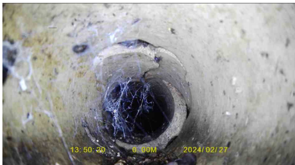
a23b21ca-4fe4-4630-a8de-9b8184f37973.jpg, 00:00:09, 0.01 m Broken pipe from 10 o'clock to 4 o'clock
