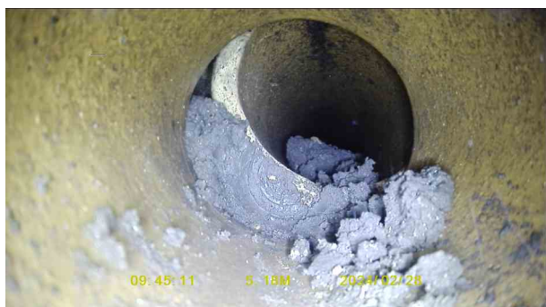
1bdab721-5f99-49eb-8ed6-be60724c47cc.jpg, 00:01:05, 5.18 m Joint displaced, large
