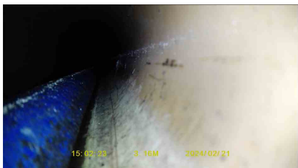
652aefee-05cd-425f-ba92-9fda5dc48866.jpg, 00:00:44, 3.16 m Other obstacles from 6 o'clock to 8 o'clock, 25%
