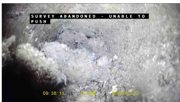
8a9a1b1c-7982-42b2-9fa4-973232a10f63.jpg, 00:00:37, 0.09 m Survey abandoned, Camera unable to pass debris
