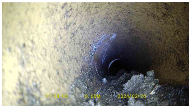
3db440e9-94a5-444e-aeac-e60b9c2334fc.jpg, 00:00:08, 0.01 m Settled deposits, fine, 20% cross-sectional area loss, start
