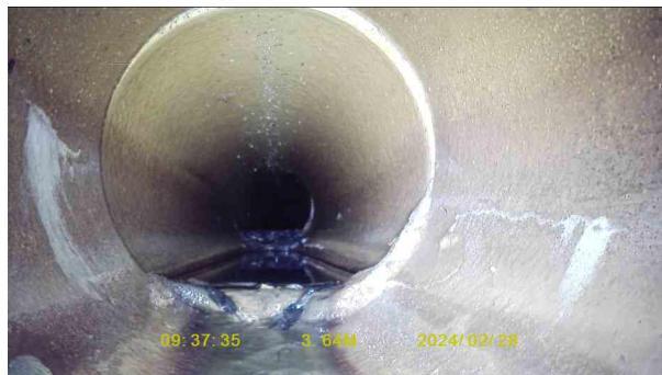
ebd01911-c836-4e43-8486-2d7c7b590947.jpg, 00:00:56, 3.63 m Crack, longitudinal at joint at 3 o'clock
