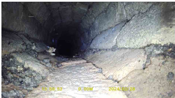
9daad588-bbf3-4842-9033-69c1b1e0e1ac.jpg, 00:00:09, 0.01 m Displaced bricks, single brick false from 5 o'clock to 8 o'clock,
