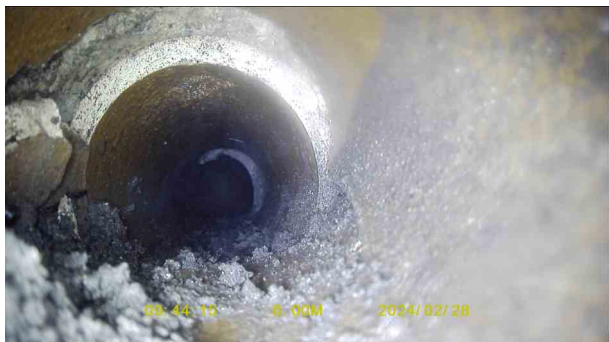
4a8f413a-cc03-46a9-92d0-e4acb1491967.jpg, 00:00:09, 0.01 m Broken pipe from 8 o'clock to 3 o'clock
