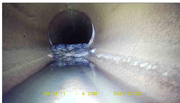
9f9a7e00-1543-4050-ab4a-f11bd25f1c40.jpg, 00:01:32, 4.22 m Water level, 15% of the vertical dimension
