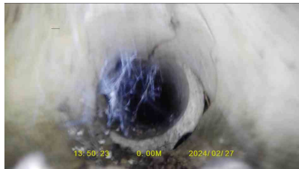
92024dd2-a8b9-4d84-8ba3-8be0c819b077.jpg, 00:00:12, 0.01 m Broken pipe from 12 o'clock to 12 o'clock
