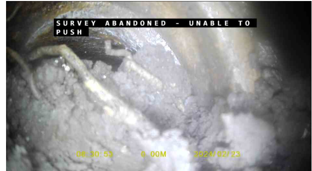
4e1a3962-058e-4481-b28a-02a7cbf8a1ee.jpg, 00:00:32, 0.01 m Survey abandoned, Camera unable to pass debris/Possibly
