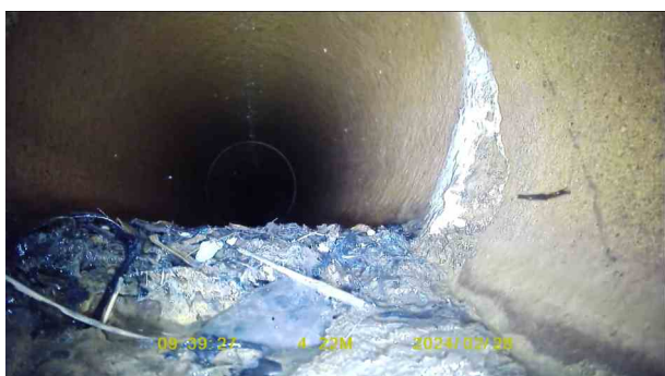
439848db-f8dc-43ef-937d-ba36c4278371.jpg, 00:01:46, 4.22 m Attached deposits, encrustation at joint from 4 o'clock to 8
