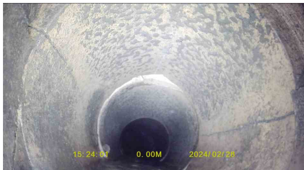
c5435cb3-f286-4d64-b0fc-d3581c1df6cc.jpg, 00:00:11, 0.01 m Fractures, multiple at joint from 12 o'clock to 12 o'clock
