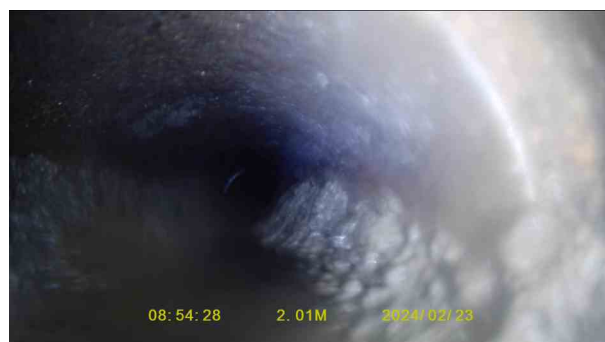
bc94ba6c-7dc1-47db-8010-2a48c268674e.jpg, 00:00:44, 2.01 m Attached deposits, encrustation from 2 o'clock to 10 o'clock,
