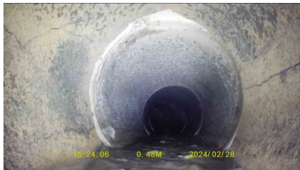
97553212-8f60-4b8f-9d8c-d75e09502bee.jpg, 00:00:16, 0.48 m Settled deposits, fine, 20% cross-sectional area loss, start
