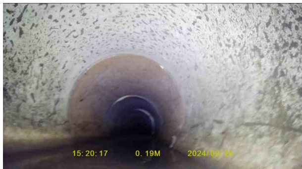
5f63d655-58e9-4f14-acae-1c6df74d127f.jpg, 00:00:08, 0.19 m Water level, 20% of the vertical dimension
