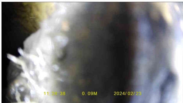
83037877-9036-41bc-b3b6-ba671c318e4d.jpg, 00:00:13, 0.09 m Roots, mass, 50% cross-sectional area loss, start
