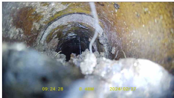
4d362faa-fbf3-4b0d-93b6-bd9cc255c001.jpg, 00:00:17, 0.48 m Joint displaced, large
