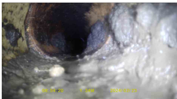
030d482c-0287-4418-866d-885ec74c349b.jpg, 00:00:35, 1.34 m Joint displaced, medium
