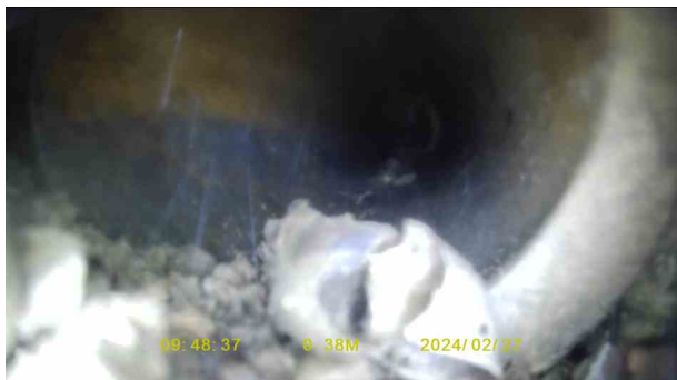
d3045543-19c3-4219-abd9-ac87c87991d2.jpg, 00:00:17, 0.38 m Joint displaced, large
