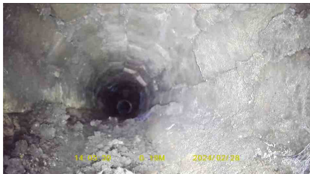
50f3a794-5c57-475e-ba55-f575440f4af4.jpg, 00:00:24, 0.19 m Displaced bricks, single brick false from 7 o'clock to 8 o'clock
