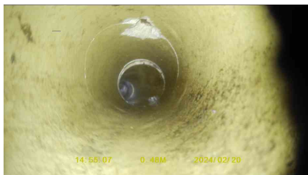
14c3398a-5bdd-49f0-861f-f12273c32275.jpg, 00:00:17, 0.48 m Hole in drain or sewer from 12 o'clock to 1 o'clock
