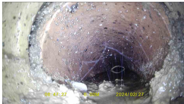
9e581c3b-0d3d-4f9a-bb58-4cf67137c14b.jpg, 00:00:12, 0.01 m Settled deposits, fine, 20% cross-sectional area loss, start
