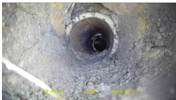
ad9bbb0e-e704-4fa8-9e06-0d4233ff08e1.jpg, 00:00:23, 1.15 m Broken pipe from 10 o'clock to 2 o'clock
