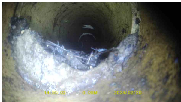
86856354-1afa-42c1-84d1-0830337bb99e.jpg, 00:00:12, 0.09 m Attached deposits, encrustation at joint from 4 o'clock to 9
