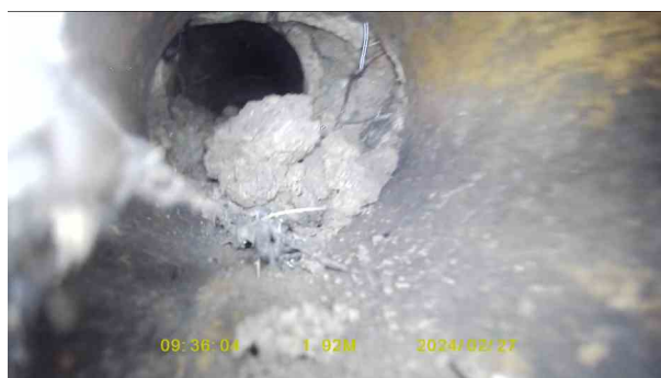
0f05dd2b-d91f-47c4-bc70-f34ff8dd0329.jpg, 00:00:51, 2.01 m Joint displaced, large
