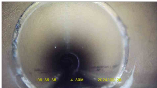
7328ea28-93b8-4f4c-a440-c1fadb94a412.jpg, 00:01:57, 4.80 m Crack, circumferential at joint from 4 o'clock to 8 o'clock
