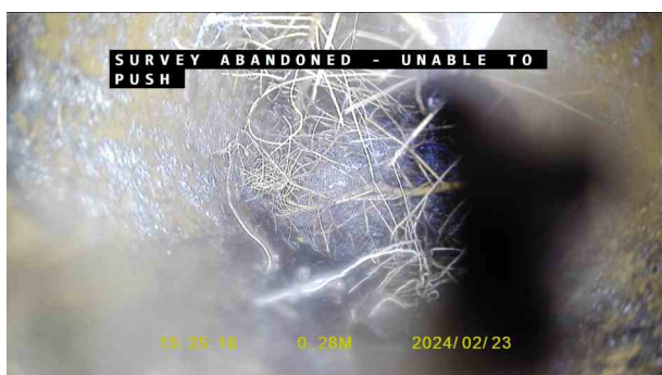
109917c3-37bb-4af2-9d07-aedc3303c8ab.jpg, 00:00:31, 0.28 m Survey abandoned, Camera unable to pass mass roots
