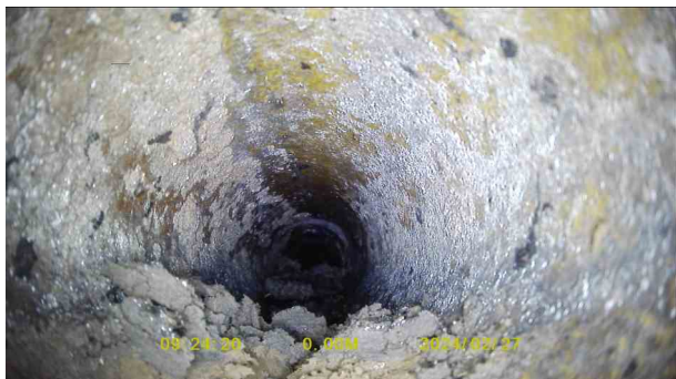
92345a1f-0f0d-44f6-92a0-a963a50cfe03.jpg, 00:00:09, 0.01 m Settled deposits, fine, 25% cross-sectional area loss, start
