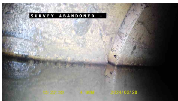
258a5039-6818-4d26-9350-7e27743fc4ad.jpg, 00:02:00, 4.99 m Fracture, circumferential from 7 o'clock to 9 o'clock
