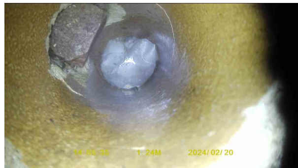
b9f3094d-c5e4-45d2-978c-aa296296d0ac.jpg, 00:00:45, 1.24 m Crack, circumferential from 12 o'clock to 3 o'clock
