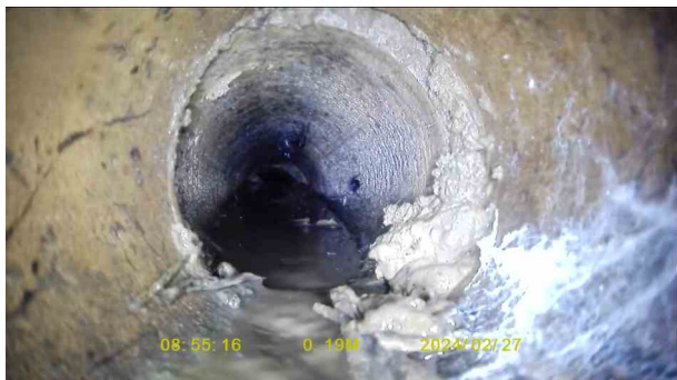
edf2ff39-8159-4d78-86fe-ecea74ac22b2.jpg, 00:00:18, 0.19 m Settled deposits, fine at joint, 20% cross-sectional area loss
