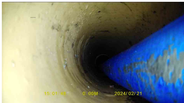
6eec8299-352a-41db-8875-d1e1097aca18.jpg, 00:00:09, 0.01 m Other obstacles from 3 o'clock to 5 o'clock, 25%
