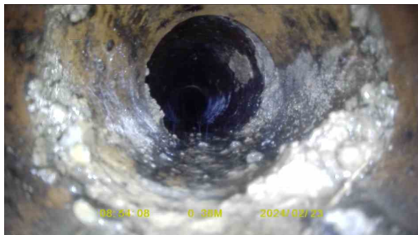
0fcb1316-8cc2-4809-8ee1-7c4c127165c4.jpg, 00:00:23, 0.38 m Settled deposits, fine, 15% cross-sectional area loss
