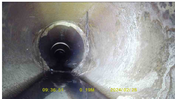
66e9acdb-f6cc-4229-983f-89ccea8f57cd.jpg, 00:00:12, 0.19 m Fracture, circumferential at joint from 12 o'clock to 12 o'clock
