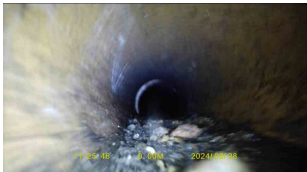
bcbbea21-a523-4d4e-80ec-5267102d0d3b.jpg, 00:00:09, 0.01 m Settled deposits, fine, 20% cross-sectional area loss, start
