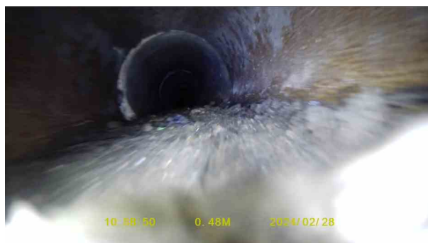
e9bc0550-c807-4021-97ad-5c5421ae3788.jpg, 00:00:28, 0.48 m Settled deposits, fine, 25% cross-sectional area loss, start
