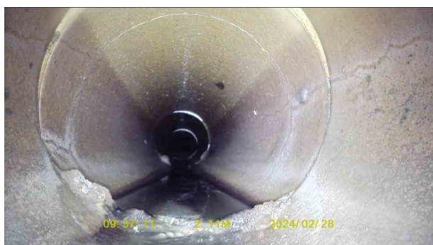
7d2cf0bc-76b2-4766-a352-9a3c8d94249f.jpg, 00:00:33, 2.11 m Crack, circumferential at joint from 8 o'clock to 3 o'clock
