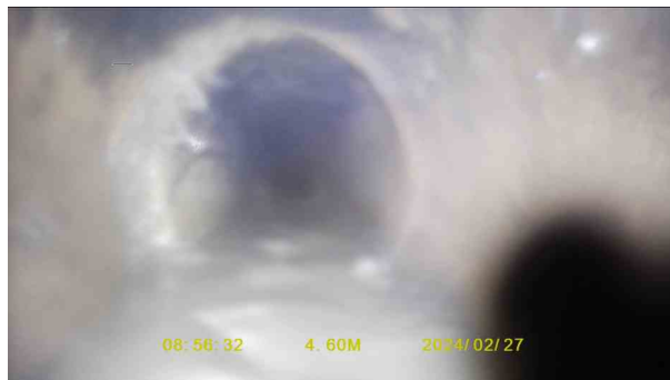
94d5bec5-9cc4-4bfd-a7b9-cdf28f2dc7ed.jpg, 00:01:14, 4.60 m Roots, fine at joint
