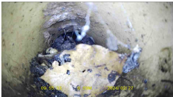
038250da-519e-4f8b-abdf-91c0b59accfb.jpg, 00:00:18, 0.09 m Settled deposits, fine, 80% cross-sectional area loss
