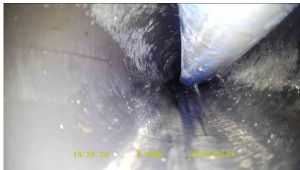
61b9777f-1c7e-484a-86c6-67b1151ca9d6.jpg, 00:00:15, 0.01 m Other obstacles from 1 o'clock to 3 o'clock, 25%
