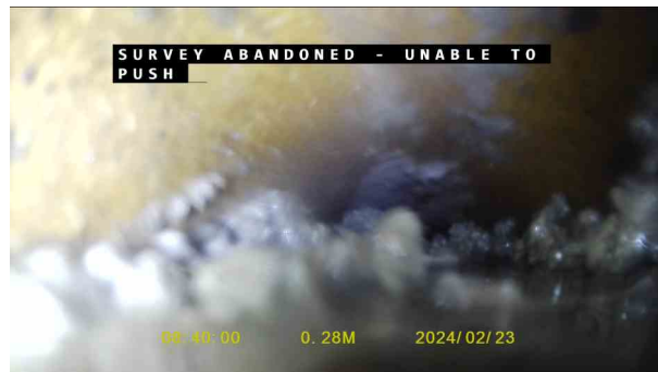
de872583-4a3d-46e0-893b-da2d77759cbe.jpg, 00:00:50, 0.28 m Survey abandoned, Camera unable to pass debris
