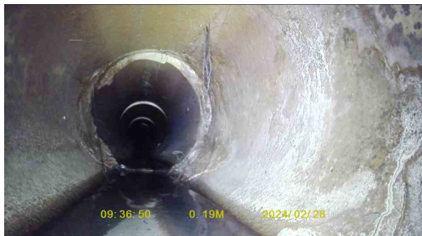
a05d4d2b-05ea-4f8a-a87e-ca702cdcea58.jpg, 00:00:12, 0.19 m Crack, circumferential from 1 o'clock to 6 o'clock
