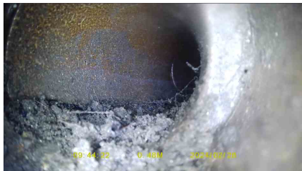
44d792b6-eefa-4f40-84b7-02f252e14b46.jpg, 00:00:16, 0.48 m Joint displaced, large
