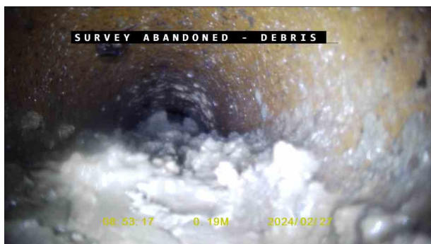
1f51dcea-61a5-4b26-9188-32764b45a606.jpg, 00:00:37, 0.19 m Survey abandoned, Camera unable to pass debris
