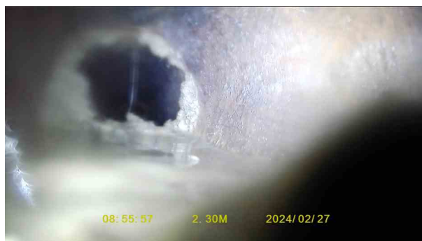
94d3f8ef-6a0a-4c91-97d6-7b3c1c3a0ecc.jpg, 00:00:41, 2.30 m Attached deposits, encrustation at joint from 12 o'clock to 12
