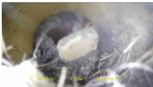
a2ef8350-c24e-4a74-906e-d14d4f6ba4c4.jpg, 00:00:32, 1.92 m Open joint, large
