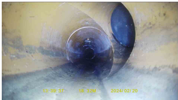
21236195-deea-4b79-833b-3a6f211d368c.jpg, 00:02:11, 18.32 m Junction at 3 o'clock, 100mm dia
