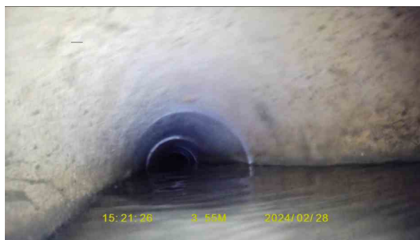
7016f20e-0a01-442c-bf39-0fb44cff4202.jpg, 00:01:17, 3.55 m Water level, 50% of the vertical dimension
