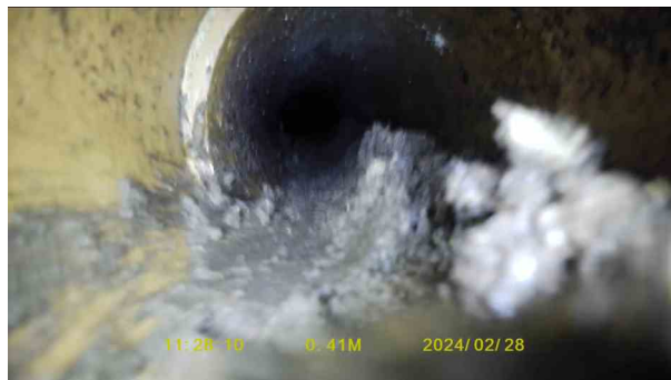
77367d56-7a45-45eb-ad78-ac012a2018e5.jpg, 00:00:13, 0.41 m Joint displaced, medium
