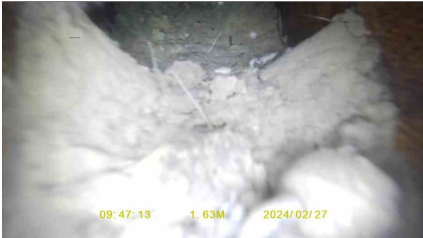
5b71ba6d-9ab2-4946-b49b-98612d70ad92.jpg, 00:00:46, 1.53 m Settled deposits, fine, 40% cross-sectional area loss
