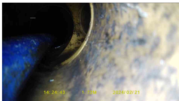
0192e6c5-b6d1-4465-baa0-62ceb47c332e.jpg, 00:00:32, 1.72 m Junction at 3 o'clock, 100mm dia
