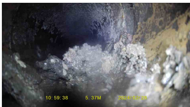
9f08fd98-dd8b-4de9-b0cf-8636eb958aed.jpg, 00:01:16, 5.37 m Joint displaced, medium
