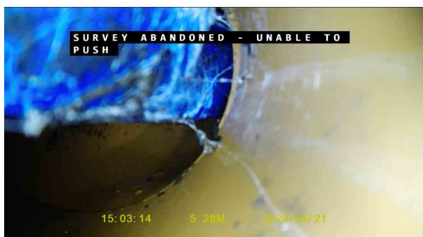
13e196f7-a1fd-4559-91dd-398bd99d5d88.jpg, 00:01:14, 5.28 m Survey abandoned, Camera unable to pass obstruction/Hose
