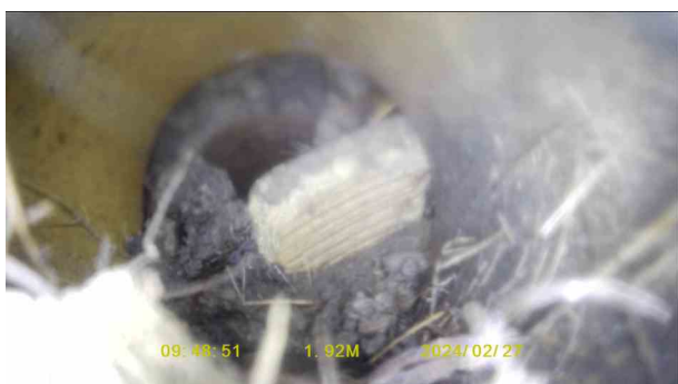
dbfd739f-4c9a-4591-864d-0acc2a40ff49.jpg, 00:00:32, 1.92 m Joint displaced, large
