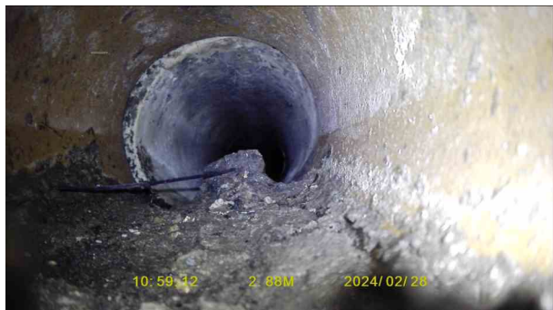
0b1fa437-c79c-4ffa-b5a3-a789f1c390e5.jpg, 00:00:51, 2.88 m Joint displaced, medium
