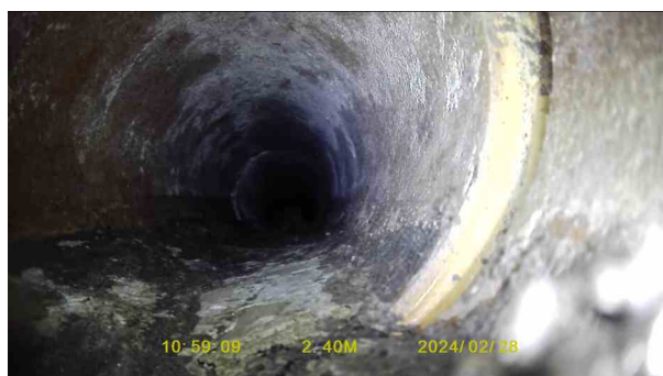
e160bc27-03a4-4946-b649-9492332ef6a9.jpg, 00:00:47, 2.40 m Joint displaced, large
