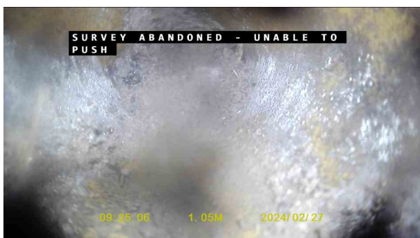
84c7cce2-2a40-4e68-aa6e-d7318382164e.jpg, 00:00:50, 1.05 m Survey abandoned, Camera unable to pass debris
