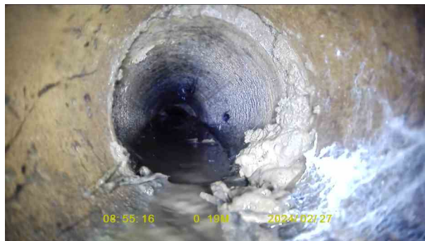
3238a81c-6958-485b-b282-015487cfd794.jpg, 00:00:18, 0.19 m Joint displaced, large
