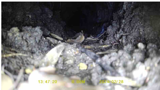
30f79e78-da89-42c6-84c5-4574d547f018.jpg, 00:00:08, 0.01 m Settled deposits, fine, 25% cross-sectional area loss, start
