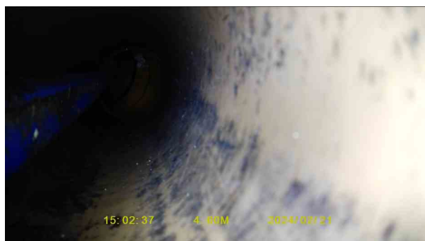
5cd0ca3e-c510-414e-ae2b-2ca209c616e0.jpg, 00:00:58, 4.60 m Other obstacles from 6 o'clock to 8 o'clock, 25%
