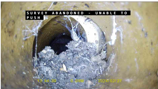
c211d4ed-8ad2-490d-99f5-3b7fd11bd9a1.jpg, 00:00:36, 0.09 m Survey abandoned, Camera unable to pass JDL/Debris
