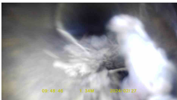
4ea99f23-bac5-42f2-9322-835a3e4b6740.jpg, 00:00:26, 1.34 m Roots, fine at joint
