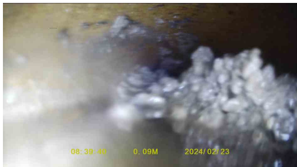
a1b0107d-d7ec-4e34-8021-ecfc20320749.jpg, 00:00:33, 0.09 m Settled deposits, fine, 70% cross-sectional area loss
