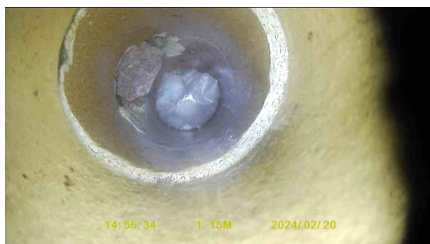
e56fef0e-9556-4087-b72a-802cf6ebdea5.jpg, 00:00:44, 1.15 m Broken pipe at joint from 1 o'clock to 9 o'clock
