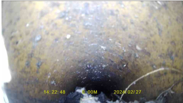
29adea43-d6da-44fe-9536-0bfdcf06eeb1.jpg, 00:00:11, 0.01 m Settled deposits, fine, 40% cross-sectional area loss, start
