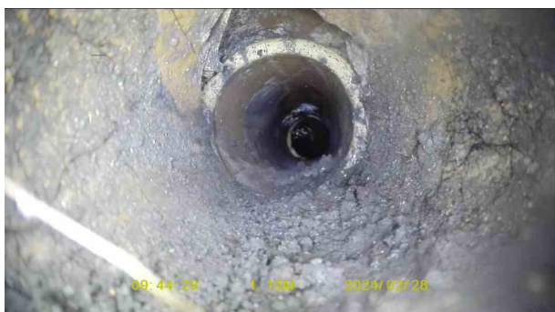
09995635-ead1-4dc6-a789-c8a85ced25e2.jpg, 00:00:23, 1.15 m Hole in drain or sewer from 10 o'clock to 2 o'clock
