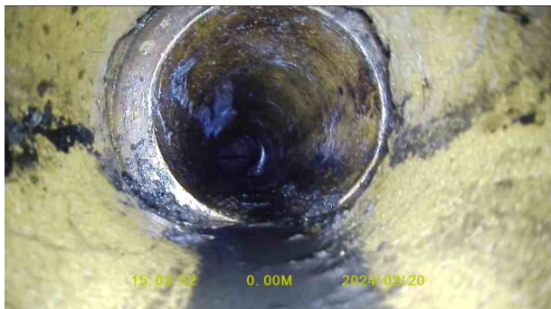
a1961974-abd4-454e-83a3-83ffb079b3ef.jpg, 00:00:12, 0.09 m Joint displaced, large
