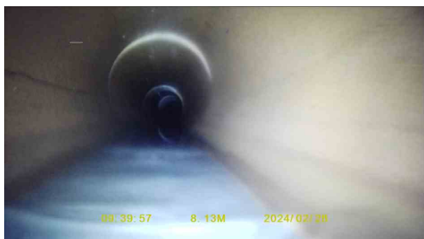
772c8bb4-0770-416f-ab1f-b12b07e31e7f.jpg, 00:02:16, 8.13 m Water level, 20% of the vertical dimension
