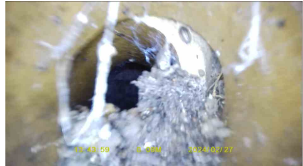
81f01e4d-074d-4ef4-9457-19227b9b81f1.jpg, 00:00:23, 0.09 m Joint displaced, large
