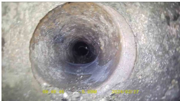
8c62f773-bc83-49bf-bd68-917fa7667e2e.jpg, 00:00:19, 0.09 m Joint displaced, large
