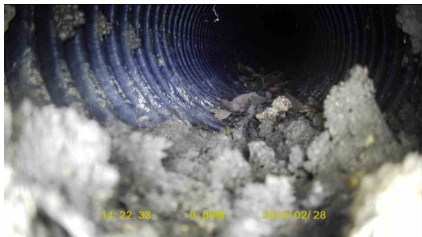
e2e8edde-2345-4477-b8a3-180d35a8a02e.jpg, 00:00:08, 0.01 m Settled deposits, fine, 15% cross-sectional area loss, start
