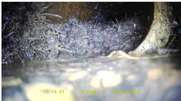
eea82ff6-2144-4d2e-9e73-eba508647f3c.jpg, 00:00:15, 0.01 m Joint displaced, large
