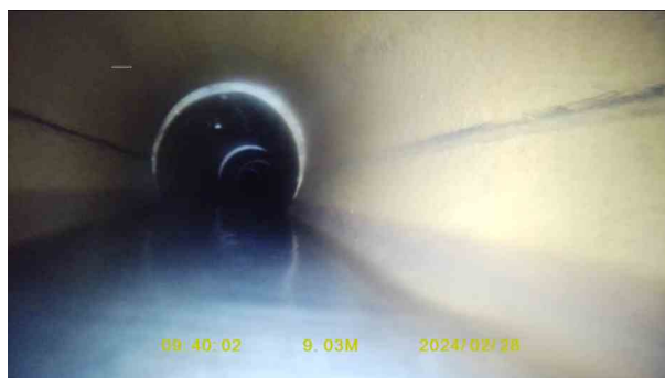
bf1ace71-eab4-4379-88e5-22d3930213c0.jpg, 00:02:21, 9.03 m Water level, 30% of the vertical dimension
