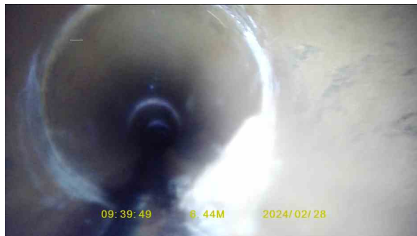
23bb68e0-1434-4e0c-94b2-39e2347e44b9.jpg, 00:02:08, 6.44 m Attached deposits, encrustation at joint from 4 o'clock to 6
