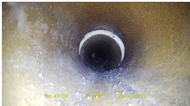
c20c070b-aacd-424d-af35-588278e04c77.jpg, 00:00:57, 4.51 m Joint displaced, large
