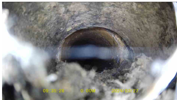
f4f2aa38-92dc-416a-a2d8-a88f5b1b0635.jpg, 00:00:15, 0.09 m Joint displaced, large
