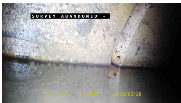
771b3f43-9f23-488c-9af6-9b8f4fbe956f.jpg, 00:02:00, 4.99 m Joint displaced, medium
