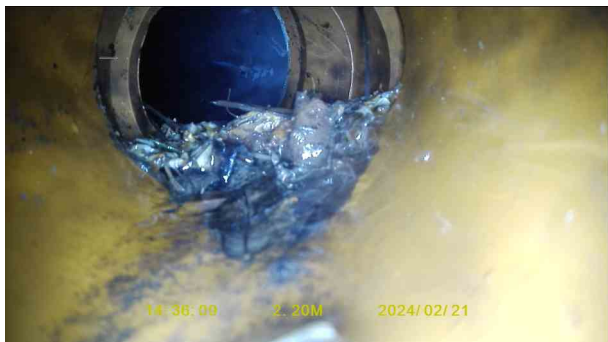
427972de-5d68-4789-ad3f-4aa0ecc2116b.jpg, 00:00:34, 2.20 m Settled deposits, fine, 20% cross-sectional area loss
