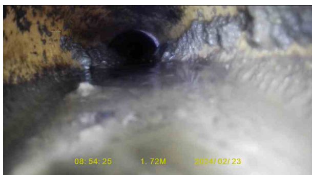
0d4ebd95-336b-45f2-a5d9-61bf48dd46ee.jpg, 00:00:40, 1.72 m Water level, 30% of the vertical dimension
