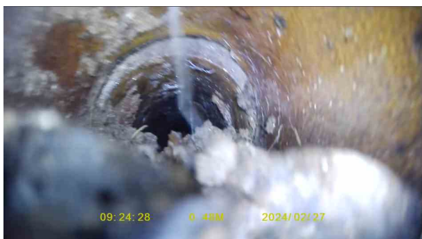
8f6fcdb9-4400-49c7-a77a-26d86cdce044.jpg, 00:00:17, 0.48 m Settled deposits, fine, 45% cross-sectional area loss, change
