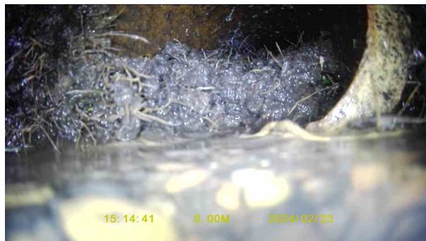
ef91b1b6-ac73-4e48-985f-3cedd3c1e5b7.jpg, 00:00:15, 0.01 m Roots, mass, 55% cross-sectional area loss
