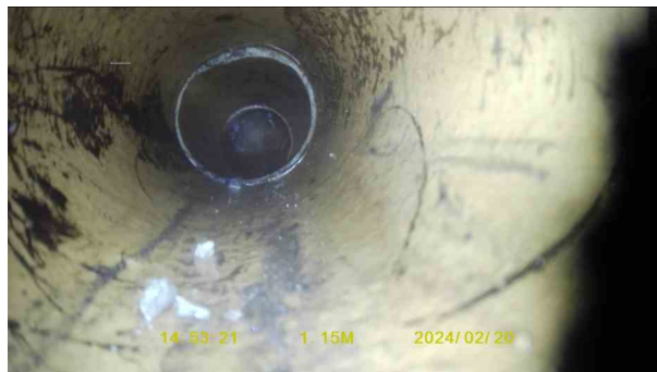
68a53500-c64f-4f04-ad8f-55b714a53d05.jpg, 00:00:21, 1.24 m Fracture, circumferential at joint from 12 o'clock to 6 o'clock
