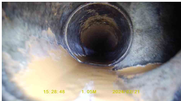
494195b3-7c1c-425d-8b00-7dca94b7ae42.jpg, 00:00:17, 1.05 m Junction at 3 o'clock, 100mm dia
