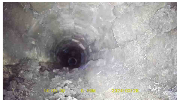
62f9f226-191d-46b7-b105-37053ebf86d5.jpg, 00:00:24, 0.19 m Settled deposits, fine, 15% cross-sectional area loss, start
