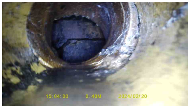
e629018d-3448-4f52-b7a0-6eb6e9a4e77e.jpg, 00:00:20, 0.48 m Joint displaced, large
