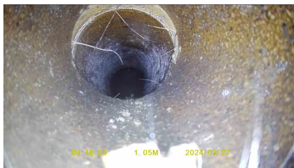
dde8d0b9-63c0-4fd6-a86c-80250d7e6d3d.jpg, 00:00:32, 1.15 m Joint displaced, large
