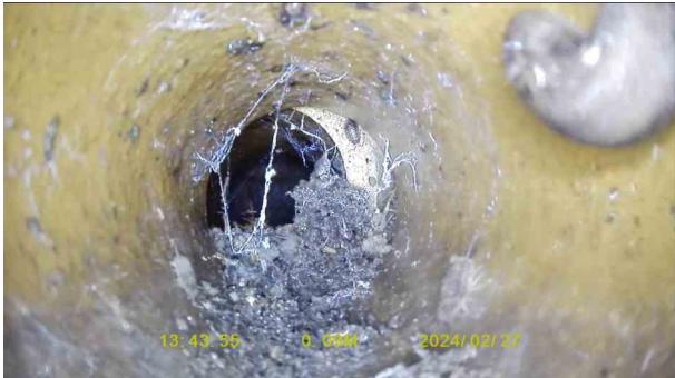
cfa26202-8514-4663-b057-0c61602bc071.jpg, 00:00:19, 0.09 m Settled deposits, fine, 20% cross-sectional area loss
