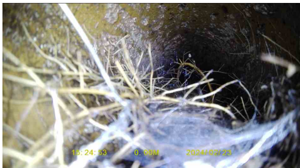
c31913d6-3e81-4ddb-a528-c2514a0cdac8.jpg, 00:00:08, 0.01 m Roots, mass, 40% cross-sectional area loss, start
