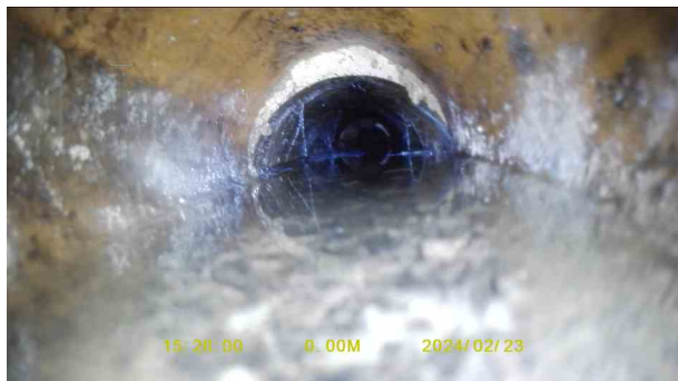
5a7b3d60-6fba-4a38-9700-a8aaf6fb1e0.jpg, 00:00:11, 0.00 m Water level, 50% of the vertical dimension
