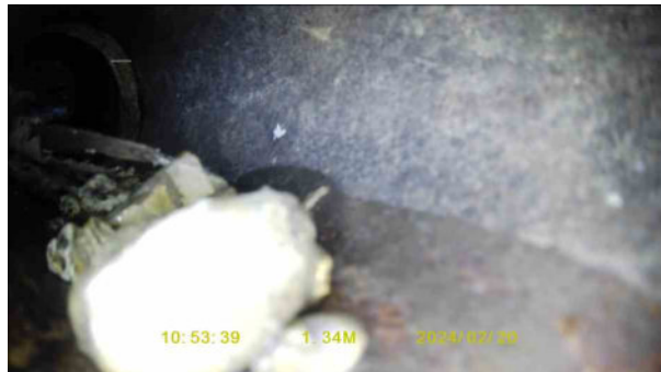
b1ec5c73-cb1b-4989-bafa-742fbe4b7188.jpg, 00:00:39, 1.15 m Settled deposits, fine, 20% cross-sectional area loss
