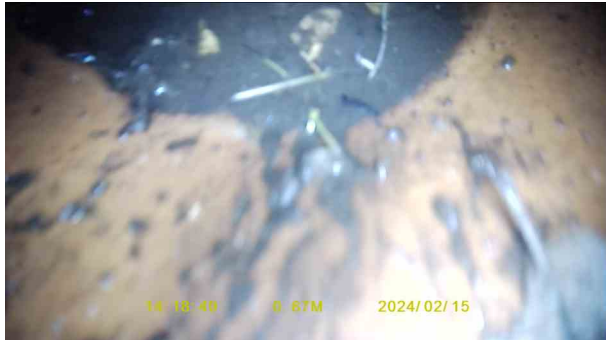
ccde89bb-de1f-44ef-bd98-8822d6aa2ec0.jpg, 00:00:28, 0.67 m Settled deposits, fine, 25% cross-sectional area loss, start
