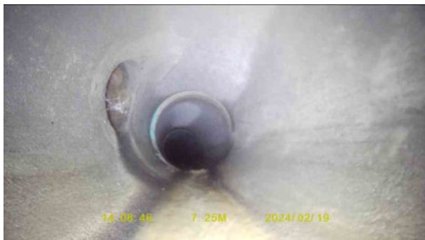
ed25be0b-d9fb-40a3-b387-61b8707a9e33.jpg, 00:01:22, 7.25 m Junction at 9 o'clock, 150mm dia
