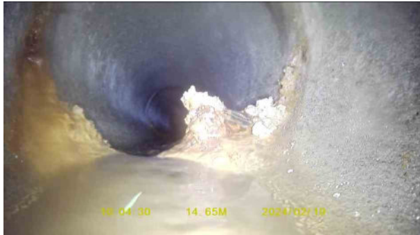
9b1df465-ba5a-4281-bed4-713f3c375753.jpg, 00:04:53, 14.65 m Attached deposits, encrustation at joint from 3 o'clock to 7
