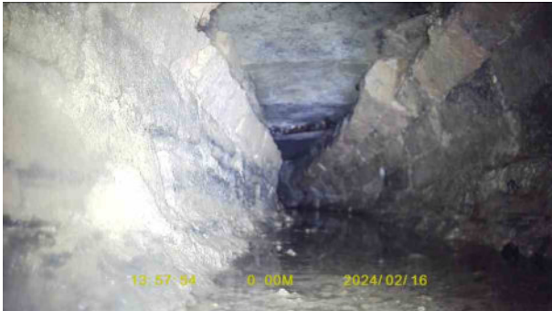
fe6ca740-4cf9-47e2-9136-ef9903ed7e3e.jpg, 00:00:09, 0.01 m Hole in drain or sewer from 10 o'clock to 2 o'clock, start
