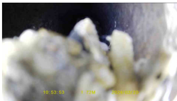
2972d6b0-2d48-4596-bb9a-7648fd527920.jpg, 00:00:47, 1.82 m Settled deposits, coarse, 30% cross-sectional area loss, start
