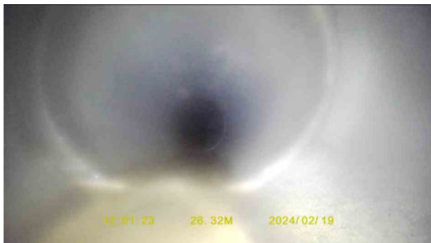
510d2746-6122-4fdc-ac3b-1094141f82cf.jpg, 00:03:03, 26.32 m Joint displaced, large
