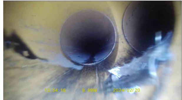
f28f0d2e-5a81-457a-95b7-6385d09598fa.jpg, 00:01:41, 9.99 m Junction at 3 o'clock, 100mm dia
