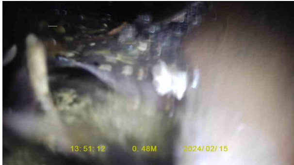
20c95e4e-6e9c-4eee-b96d-9d31401beb11.jpg, 00:00:22, 0.48 m Settled deposits, fine, 25% cross-sectional area loss, start
