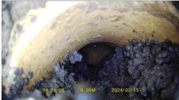
7ba87c9a-6b39-42d4-ae10-ec3c1a5078b6.jpg, 00:00:19, 0.01 m Settled deposits, fine, 30% cross-sectional area loss
