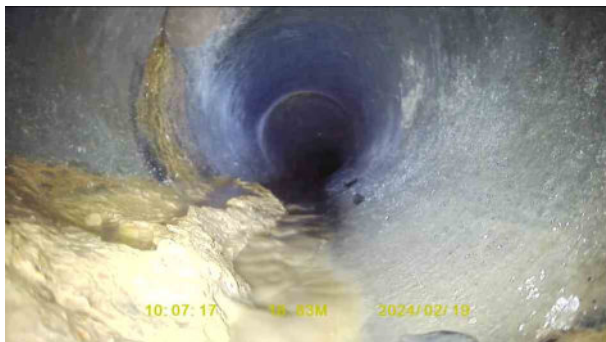
5fc6656d-dacf-4208-bb80-f0a318aef99e.jpg, 00:06:04, 18.83 m Junction at 11 o'clock, 100mm dia
