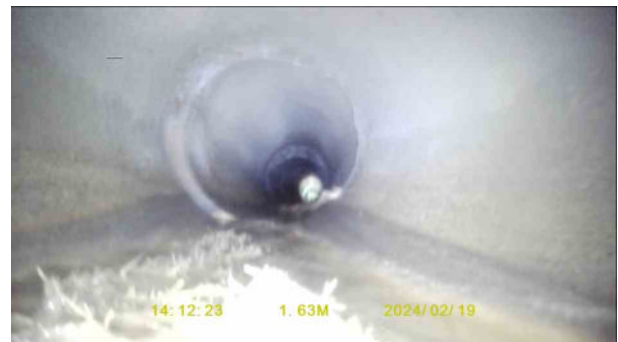
979dab86-6af4-43fd-83df-ea5f15483789.jpg, 00:00:39, 1.63 m Joint displaced, large
