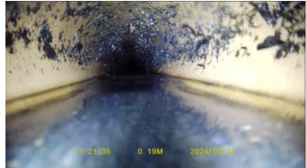
0a57784d-e58e-4407-8287-cf7a23f7a03b.jpg, 00:00:18, 0.19 m Settled deposits, fine, 20% cross-sectional area loss, start
