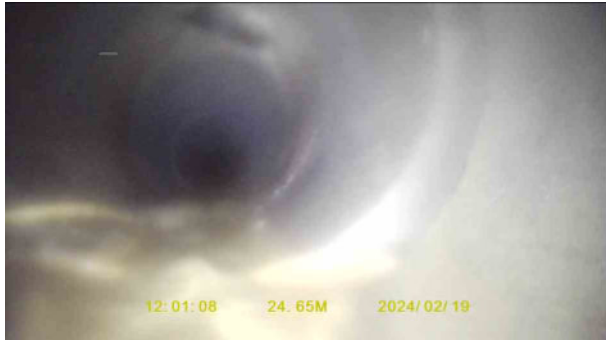
48778814-9246-4c73-ba73-c912ead5b075.jpg, 00:02:49, 24.65 m Joint displaced, large
