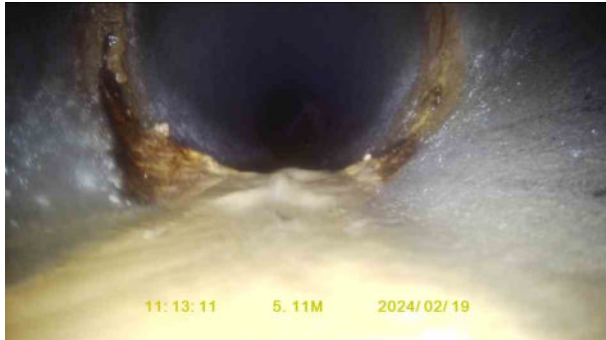
d7657106-80da-4f98-885f-3660c731a98d.jpg, 00:01:17, 5.11 m Attached deposits, encrustation at joint from 12 o'clock to 12
