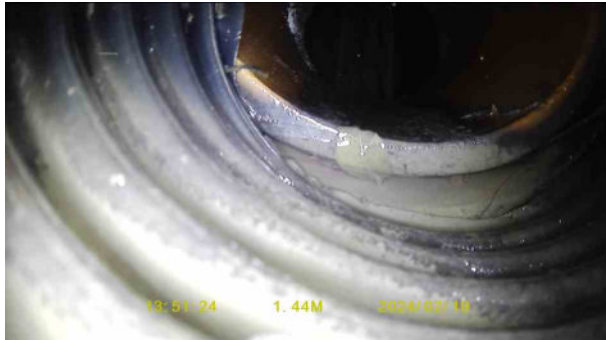
77433b44-5b3a-43c0-89b1-d2bb0d35f7f7.jpg, 00:00:17, 1.44 m Joint displaced, large
