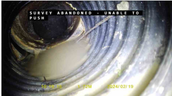
46a9c229-a384-4b90-8825-e392ff907ccf.jpg, 00:00:21, 1.72 m Pipe material changes to vitrified clay at this point
