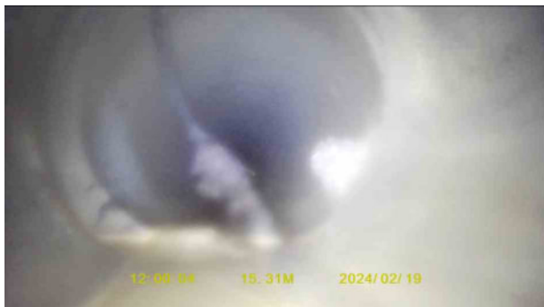
cfd37089-f5b5-48ce-ac96-437949ebdf9e.jpg, 00:01:44, 15.31 m Roots, tap at joint
