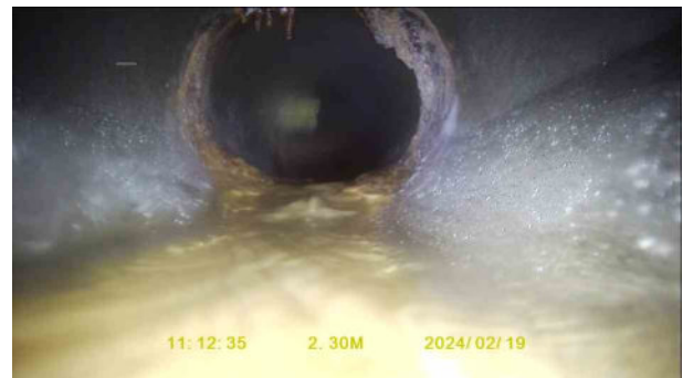
32e4f982-7d43-48bf-8c44-f932a7952cc4.jpg, 00:00:41, 2.30 m Attached deposits, encrustation at joint from 12 o'clock to 12 o'clock, 15% cross-sectional area loss
