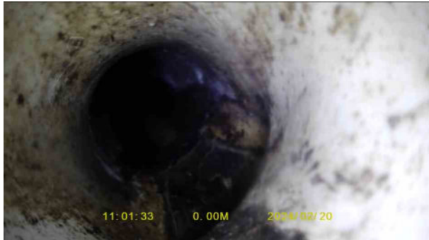
11f4fc9c-ba19-4aad-aca7-5fdd34d41401.jpg, 00:00:08, 0.09 m Junction at 6 o'clock, 100mm dia, Backdrop
