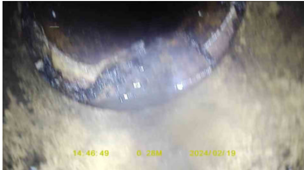
19414010-d444-4786-ba73-fbb897affb06.jpg, 00:00:18, 0.28 m Joint displaced, large
