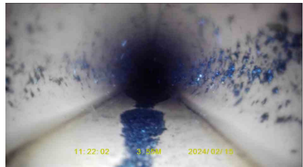
ed78403e-130b-4de6-bf97-45cb9d68f741.jpg, 00:00:45, 3.55 m Water level, 15% of the vertical dimension
