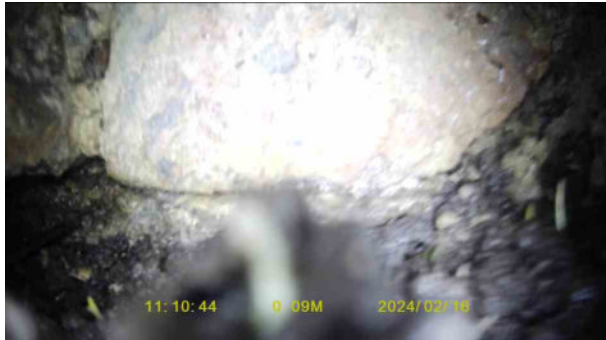
f02a77e9-e2f1-4c09-8064-3d1f006b46ec.jpg, 00:00:26, 0.09 m Settled deposits, fine, 30% cross-sectional area loss
