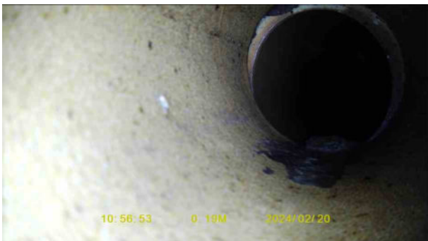
205e2d51-6137-455f-aa65-6f6f489f32b0.jpg, 00:00:18, 0.28 m Joint displaced, medium
