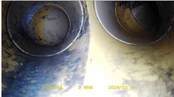
41f72c97-9439-41e7-b088-fc9b7d6f4cbe.jpg, 00:00:17, 0.96 m Junction at 3 o'clock, 100mm dia
