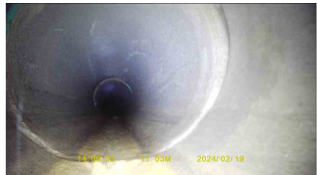
c0b29321-b805-4a0e-ad8a-f4155bcd4b7.jpg, 00:01:41, 11.03 m Joint displaced, medium
