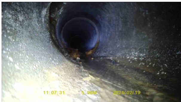
884efa80-ca89-4eb6-874e-267426a38cd7.jpg, 00:01:14, 5.96 m Junction at 10 o'clock, 150mm dia
