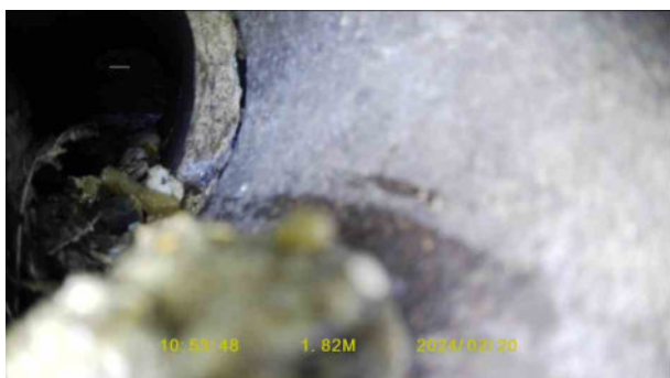
d2831d65-8e38-403f-8a5f-c8cc4d858d74.jpg, 00:00:42, 1.82 m Joint displaced, medium
