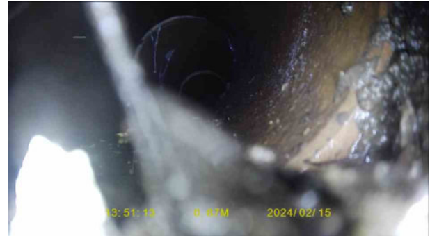
afcd81bb-6da3-4ec1-b5c4-cda859859e55.jpg, 00:00:23, 0.67 m Joint displaced, large
