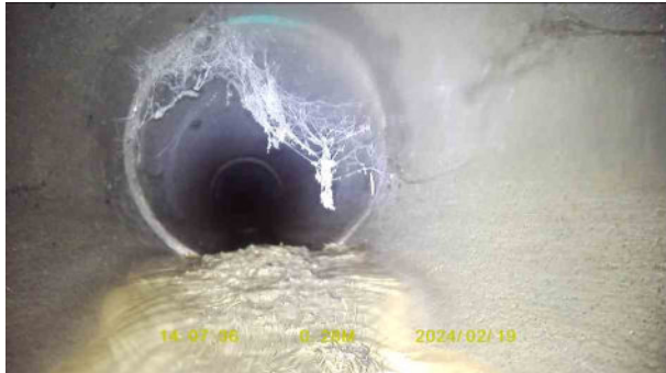
c90c49cb-90c8-4c29-b9e6-25c9edb953bc.jpg, 00:00:15, 0.28 m Settled deposits, fine, 20% cross-sectional area loss
