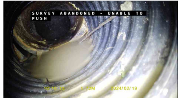
46a9c229-a384-4b90-8825-e392ff907ccf.jpg, 00:01:00, 1.72 m Joint displaced, large
