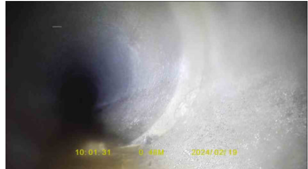
577c0377-0c71-499c-9544-72f3aa53bc83.jpg, 00:01:03, 0.38 m Joint displaced, medium
