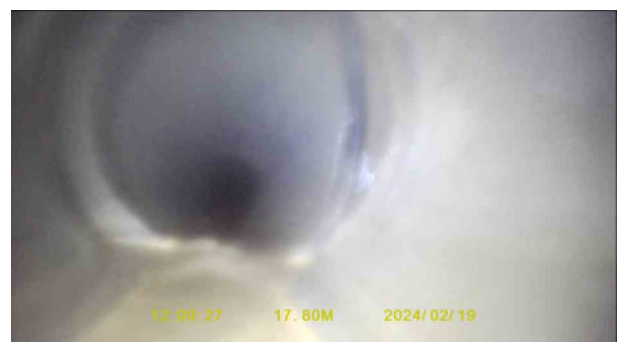
077590d8-4c9b-4e1f-9992-55e9dadfdb62.jpg, 00:02:08, 17.89 m Joint displaced, large
