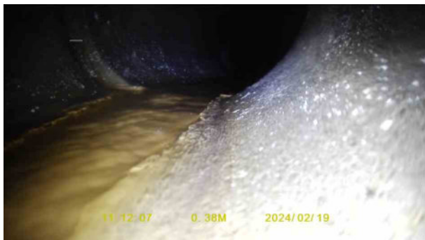
43fb38b2-6110-4a95-8fd4-09d5dc22a300.jpg, 00:00:13, 0.38 m Joint displaced, medium
