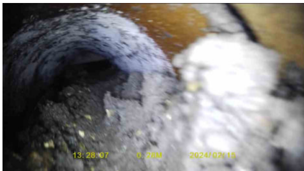
506d008a-a4ca-4920-9f11-68f6314c14b6.jpg, 00:00:21, 0.29 m Joint displaced, medium
