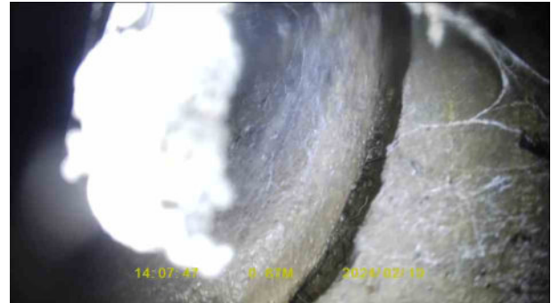
ef996390-ddfa-4960-9671-61ea9d940e87.jpg, 00:00:24, 0.67 m Joint displaced, medium
