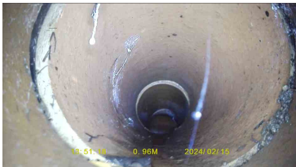
7b959420-30df-46fe-8b1c-021aa6c8dd4c.jpg, 00:00:28, 0.96 m Joint displaced, medium
