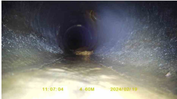
ea7c058d-daa4-4996-92bc-a8d505804fc6.jpg, 00:00:48, 4.60 m Junction at 2 o'clock, 150mm dia
