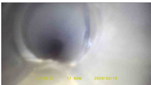
6aaf9e92-ed2e-4459-af05-5463ec3b53e4.jpg, 00:02:08, 17.89 m Roots, tap at joint
