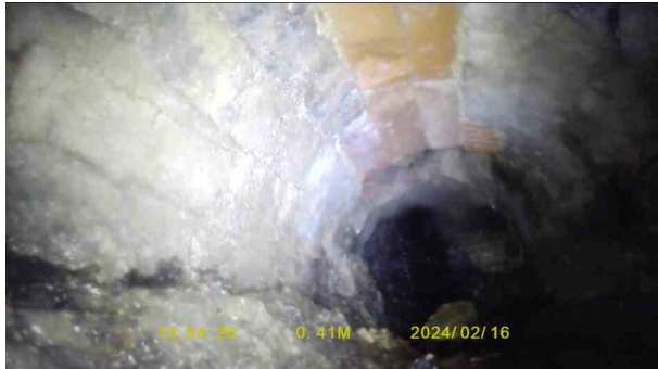
4ef6300e-2f9d-4306-95ef-b6cd0994d147.jpg, 00:00:14, 0.41 m Broken pipe from 8 o'clock to 9 o'clock, start
