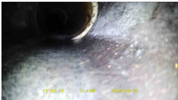
81136733-b89d-435f-a60c-a6bc873af195.jpg, 00:00:46, 3.45 m Joint displaced, medium
