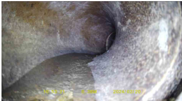
94c4cd49-8989-4d64-ba70-694f6b00c783.jpg, 00:00:15, 0.38 m Joint displaced, medium
