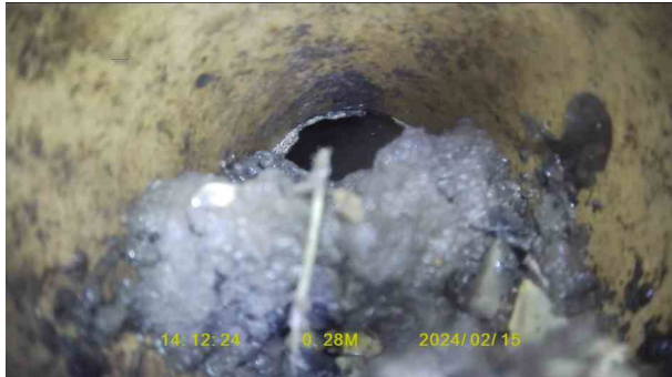
0b747a0b-873a-46c3-b4fc-464612ea82f8.jpg, 00:00:22, 0.28 m Settled deposits, fine, 75% cross-sectional area loss
