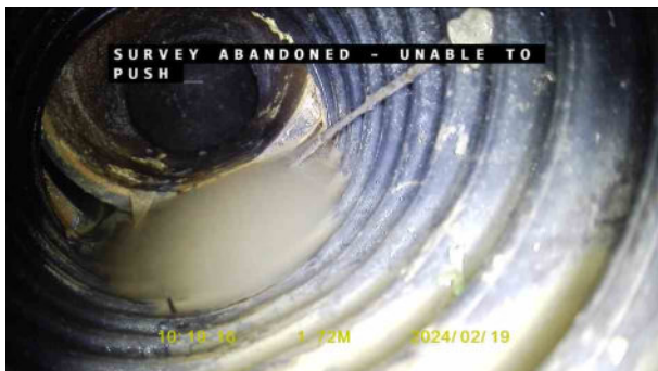
a12f9621-363e-4716-a179-4259851e7146.jpg, 00:01:00, 1.72 m Open joint, large
