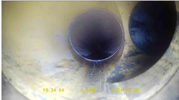
1cff4279-29bc-41d9-a284-c0b1df4fa83c.jpg, 00:01:28, 8.64 m Junction at 3 o'clock, 100mm dia
