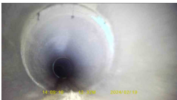
e3ef380b-964e-4a72-a3f0-f538712dbf1e.jpg, 00:01:47, 12.32 m Joint displaced, medium
