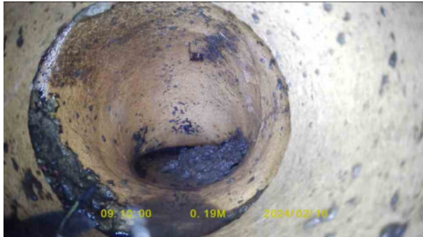
8f0bf5e6-2d78-4aa6-8b3c-8a2c8bcc296.jpg, 00:00:20, 0.19 m Joint displaced, medium
