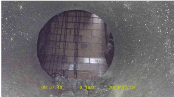
a193fc46-fa23-471b-ba4e-6ba2f7f41d1e.jpg, 00:00:14, 0.19 m Settled deposits, fine, 15% cross-sectional area loss
