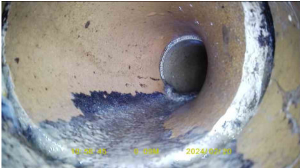
7076801a-6240-41d9-a416-603246e932b2.jpg, 00:00:10, 0.09 m Joint displaced, medium
