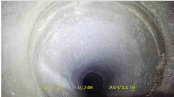
665fee94-ec28-4250-ae46-7b492f39d699.jpg, 00:00:39, 0.28 m Joint displaced, medium
