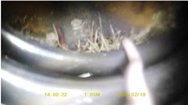
75738fd2-057a-42e3-8af6-84ea17b29526.jpg, 00:00:21, 1.05 m Roots, fine at joint
