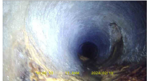
3d116580-de87-4474-93a6-ef091f7398f8.jpg, 00:05:39, 17.84 m Junction at 2 o'clock, 150mm dia
