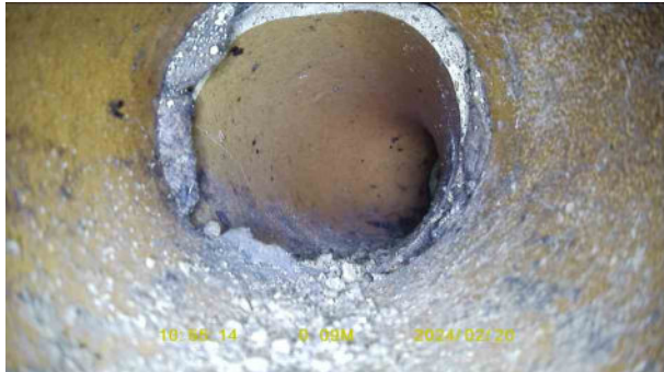
c9179bda-0f0a-4f25-a2db-2d0fef5be277.jpg, 00:00:13, 0.09 m Attached deposits, encrustation at joint from 7 o'clock to 11 o'clock, 15% cross-sectional area loss
