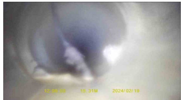
5bc5e9c3-7372-459e-bec9-e99023f639ba.jpg, 00:01:44, 15.51 m Joint displaced, large
