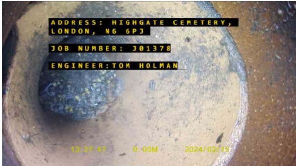
397b982f-a76e-453f-83c7-2e7946c7e29a.jpg, 00:00:01, 0.01 m Broken pipe at joint from 8 o'clock to 11 o'clock
