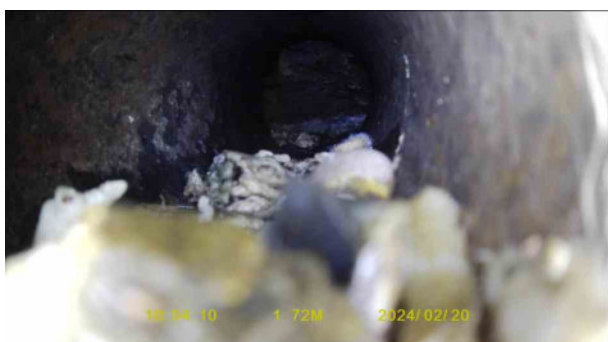
1dff81b8-6366-44e7-99e8-c7580857e882.jpg, 00:01:04, 1.82 m Survey abandoned, Camera unable to pass debris
