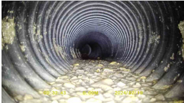
a2dc3797-f61a-4ba7-bb9a-1e1d3a959971.jpg, 00:00:11, 0.01 m Settled deposits, fine, 20% cross-sectional area loss, start
