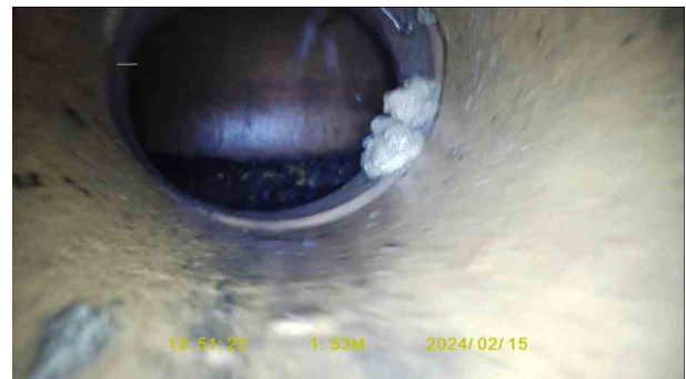
f1f2450b-46f3-4ac6-8aa2-235a2dc617f9.jpg, 00:00:34, 1.53 m Attached deposits, encrustation at joint from 3 o'clock to 4 o'clock, 15% cross-sectional area loss
