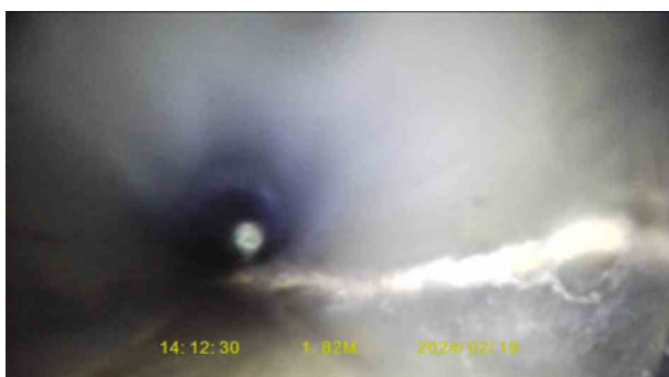
5769829f-e1f7-44b6-84d6-26706f8fbbf2.jpg, 00:00:46, 1.82 m Roots, tap at joint
