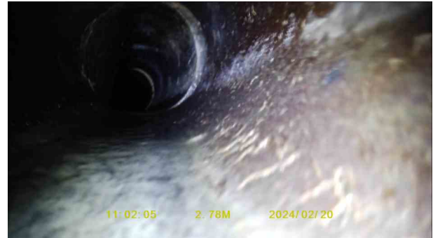
f655621c-2490-4b57-b90c-2478f909dfd8.jpg, 00:00:39, 2.78 m Joint displaced, medium
