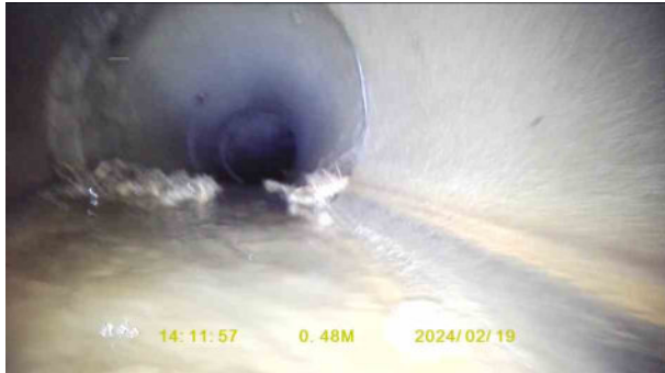
9ef8f719-6f34-4061-9c71-530c3ecf69fb.jpg, 00:00:12, 0.48 m Joint displaced, large
