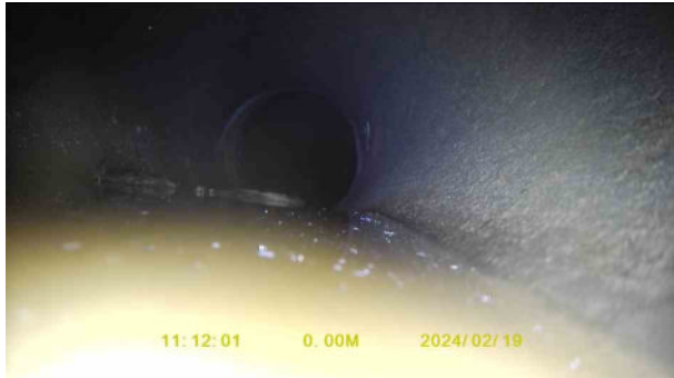
8baffc00-1084-4684-bc2b-f94469492d02.jpg, 00:00:08, 0.01 m Water level, 15% of the vertical dimension
