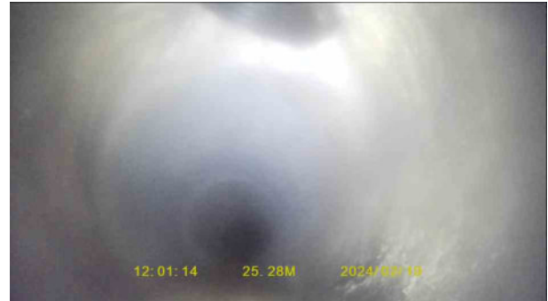
5c7aa283-64f9-4da0-b400-cf3cc3160b30.jpg, 00:02:54, 25.28 m Junction at 1 o'clock, 150mm dia
