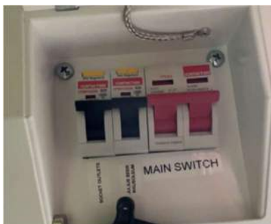
Figure 4 and 5 – North Lodge Electrical Distribution Board and Secondary Supply
