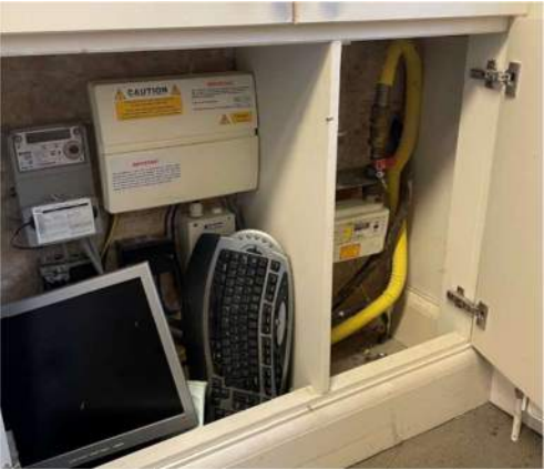
Figure 3 – South Lodge Electric Meter/ Distribution Board and Gas Meter
