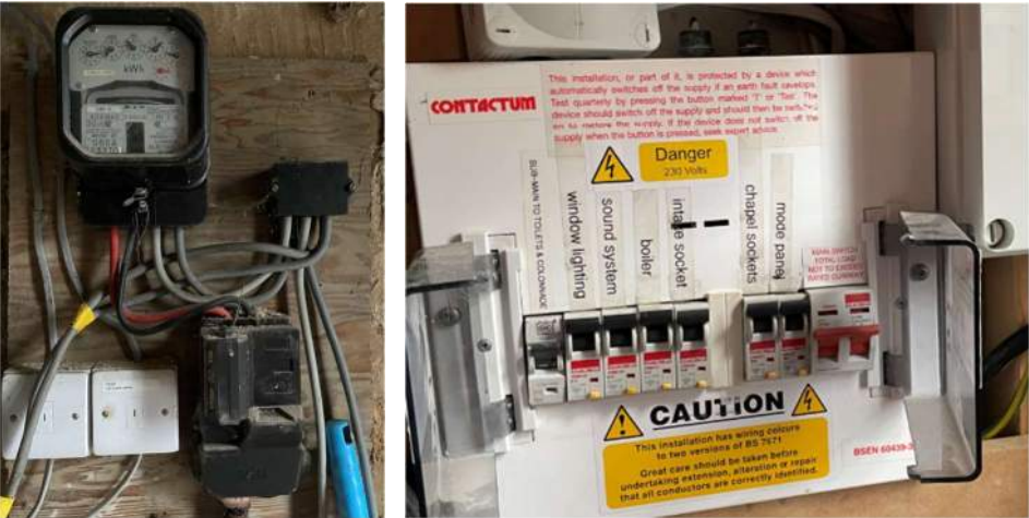
Figure 1 and 2 – Main Office Electrical Intake and Distribution Board
