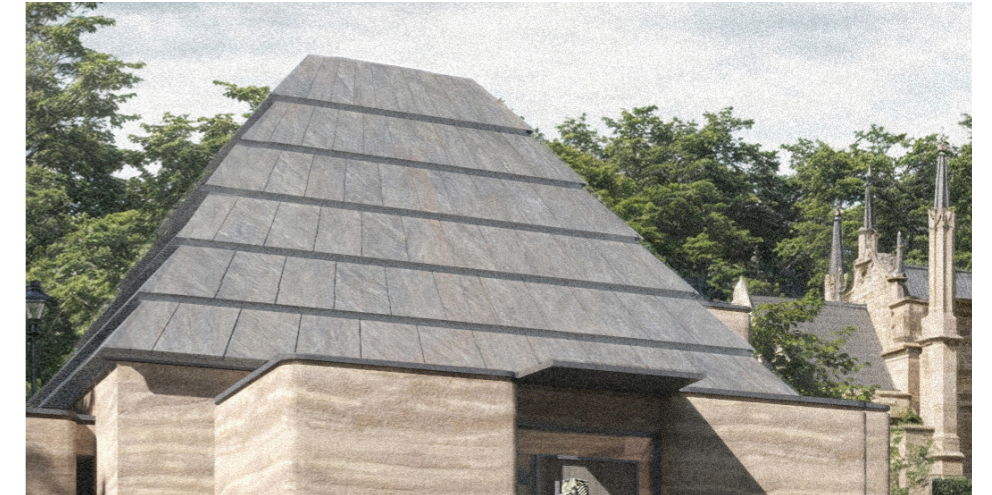
Large format slate tiles to roof of the Education and Community Building
