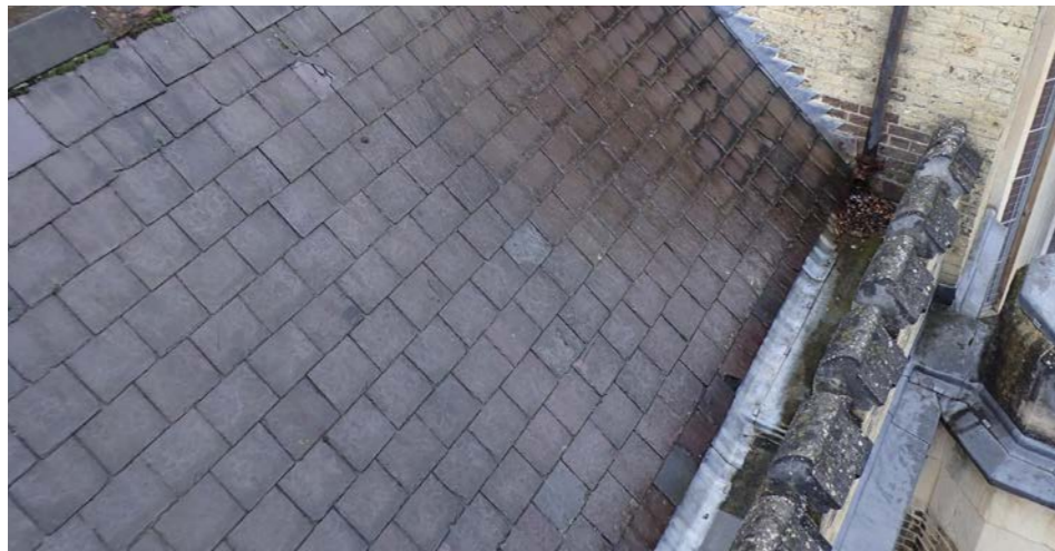
Slate shingle roof to Highgate Chapel.
