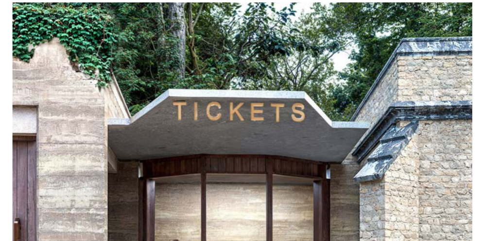
Slate canopies to Visitor and Operations Building.
