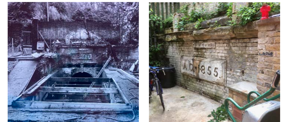
View of Tunnel during / after construction of existing compound.
