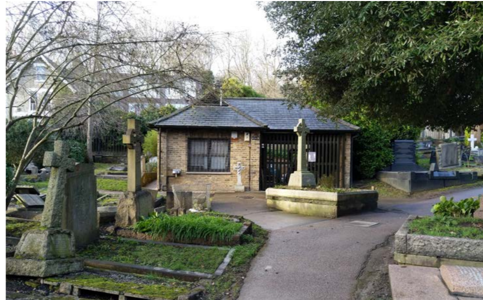
Photograph of the existing East Compound Building.
