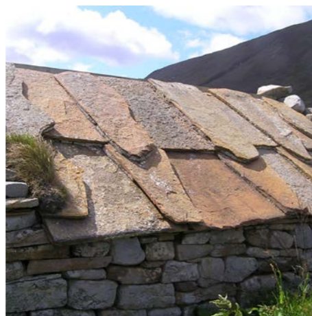
Ref: Large Format Stone Slab Roof, Hoy.
