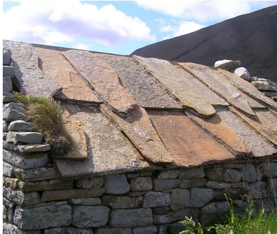
Caithness Large Format Stone Slab Roof, Hoy, Orkney
