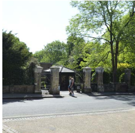
Photograph of existing Swain's Lane gate.
