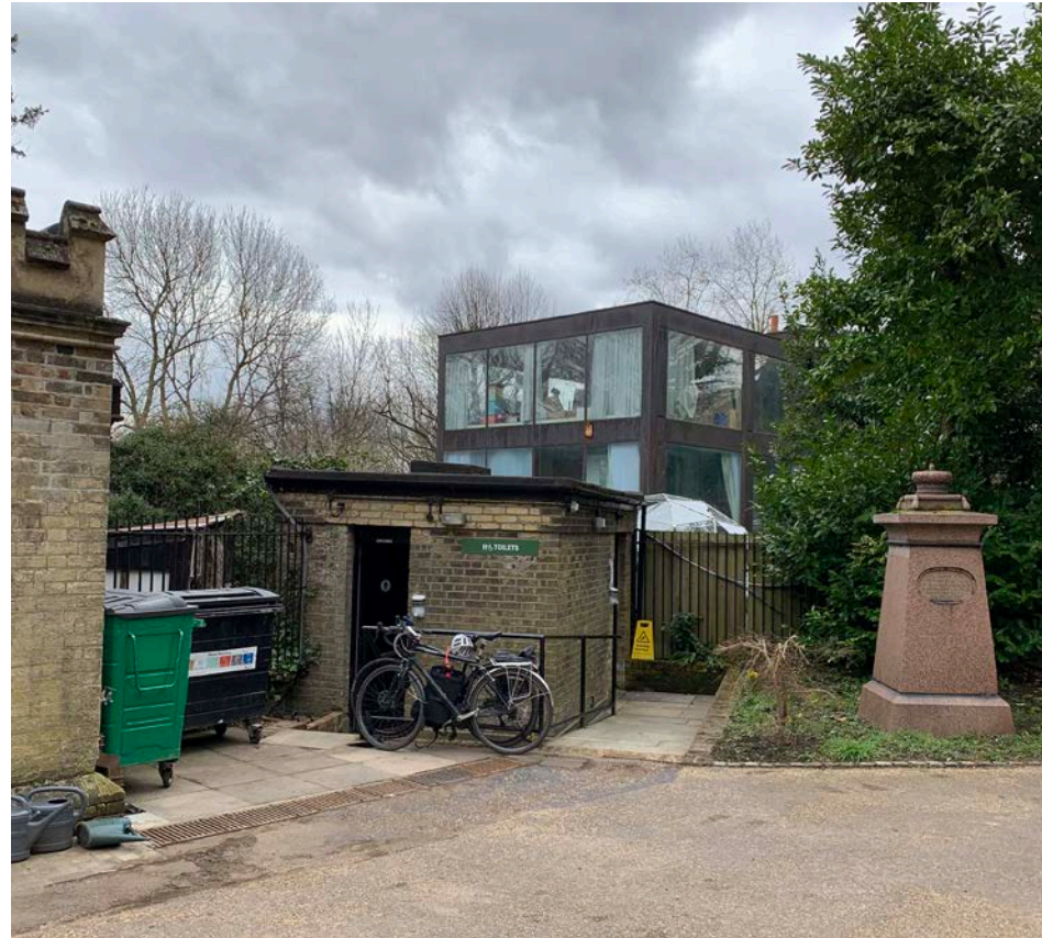
Photograph of the existing toilet block
