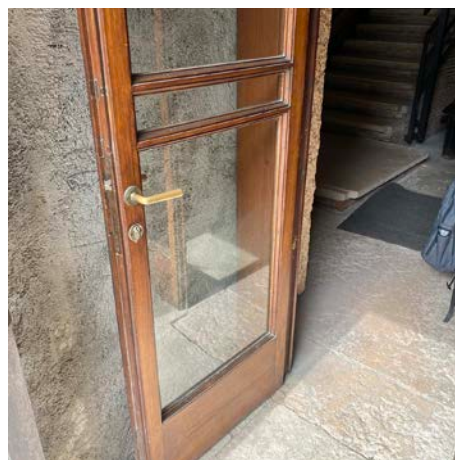
Custom Timber-framed glazing.
