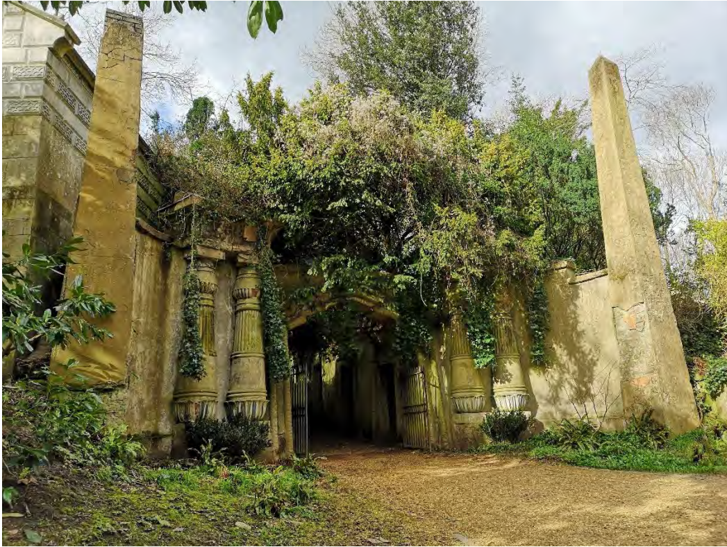
Figure 19: The Egyptian Avenue is of aesthetic value as a grand and unique monument within the cemetery. However, the imbalance caused by losing the left-hand obelisk head and the cornice has diminished this architectural interest because its original design has been made less legible.
