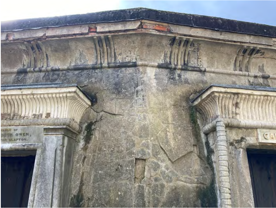
Figure 17: Original render has been pinned back to the walls of the monument. Grooves incised into the grout differentiate between old and new.
