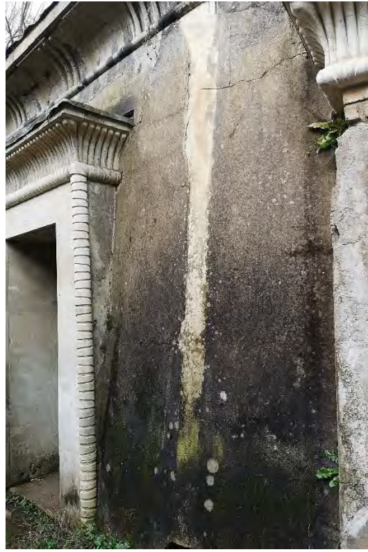
Figure 13: Drainpipe rendered over
