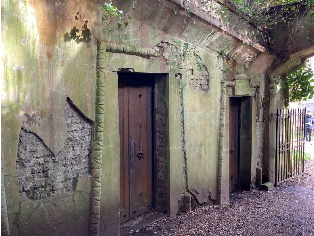
Figure 20: Exposure of the monument's brick core contributes to the aesthetic value of the Egyptian Avenue as an expression of romantic ruination. This has mostly not diminished its aesthetic value because decorative details, like its door surrounds, are still clearly legible.
