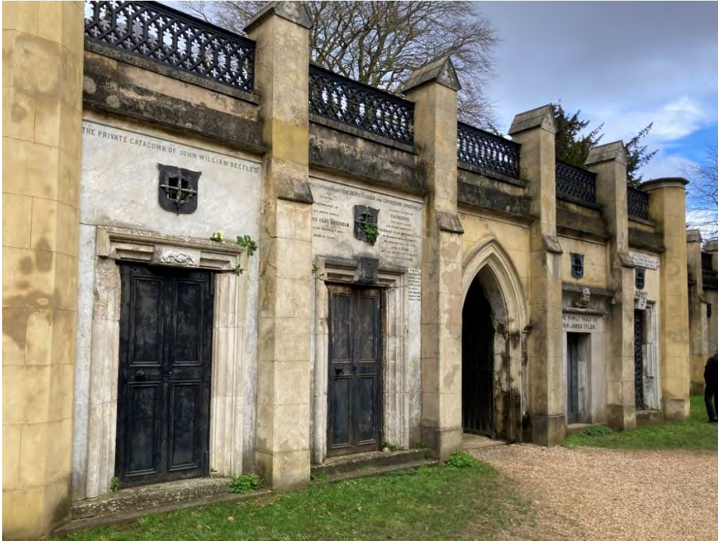
Figure 21: Modern render repairs have consolidated the Terrace Catacombs' external elevations and partly restored its original appearance. However, this is at odds with the less upkept masonry portals.
