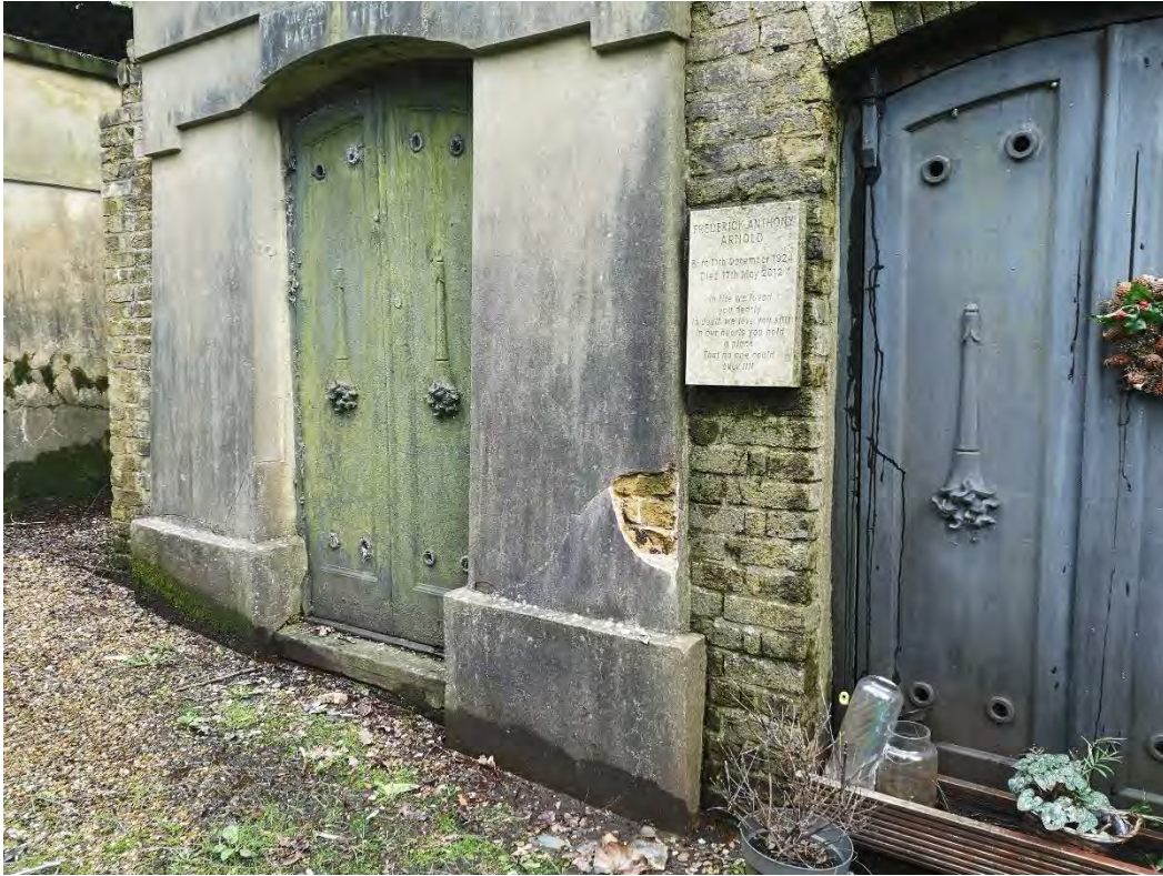
Figure 23: The exposure of underlying brickwork beneath the Cuttings Catacombs' rendered portals detracts from the illusion of masonry and gives the monument a neglected appearance. This is because the aesthetic value of the Cuttings Catacombs' original design outweighs the aesthetic value of their ruination.
