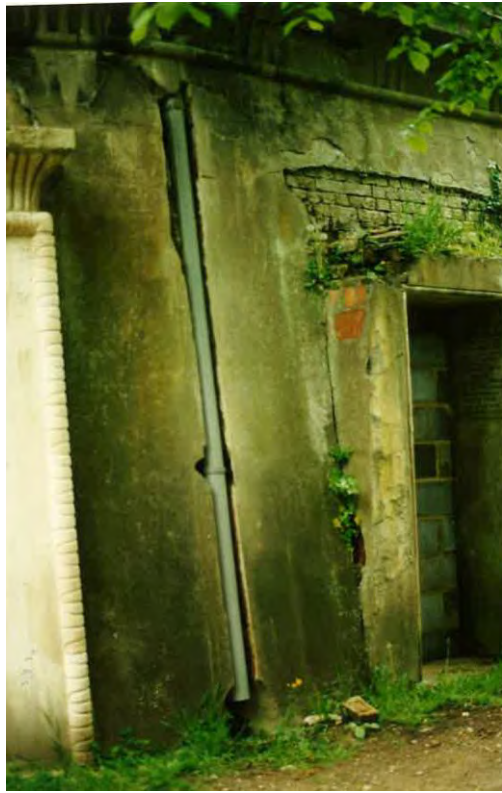
Figure 12: Exposed drainpipe
