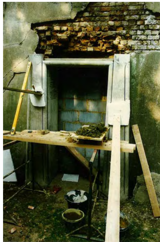
Figure 9: New marble dressings being applied to the doorcase, 1994
