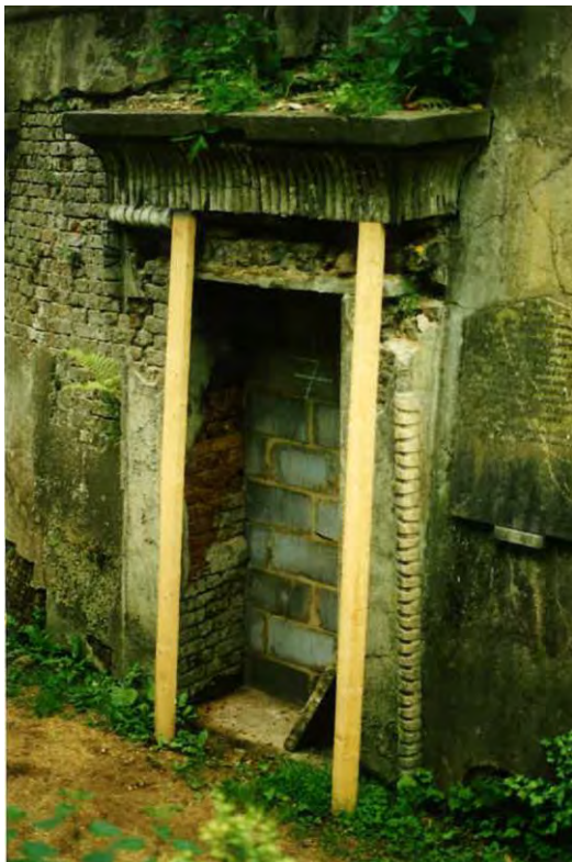
Figure 4: Portal to Vault 7 prior to conservation, cornice supported by timber posts.
