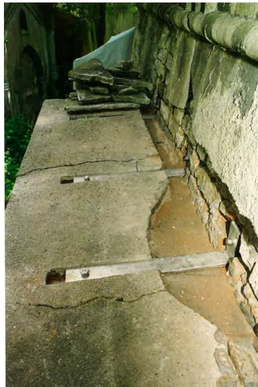
Figure 5: Inserted steel straps to fix the cornice to the wall
