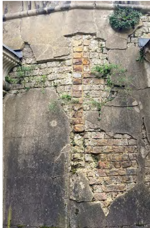
Figure 11: Filled in drainpipe trench
