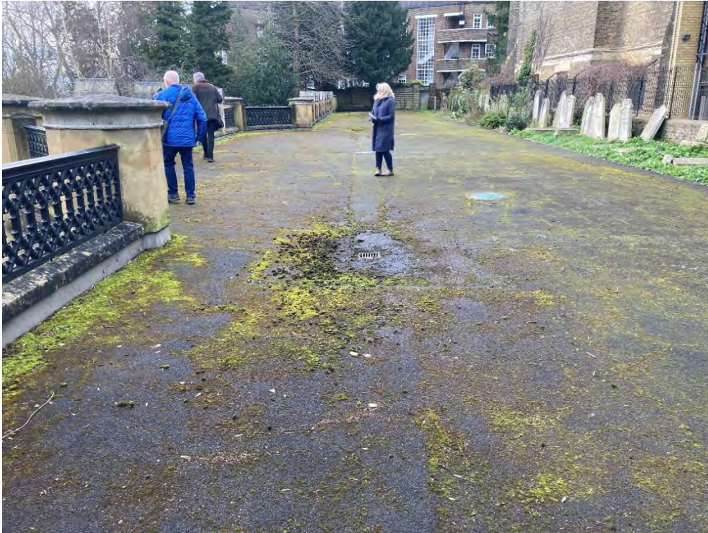
Figure 22: The modern tarmac on the roof of the Terrace Catacombs detracts from its aesthetic and evidential values because it is unsightly and presently causes water ingress problems inside the monument.
