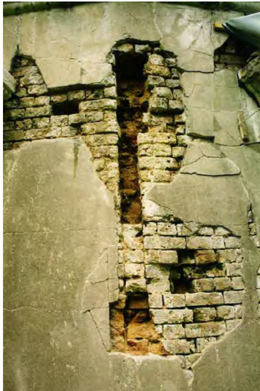
Figure 10: Exposed drainpipe trench at corner of monument
