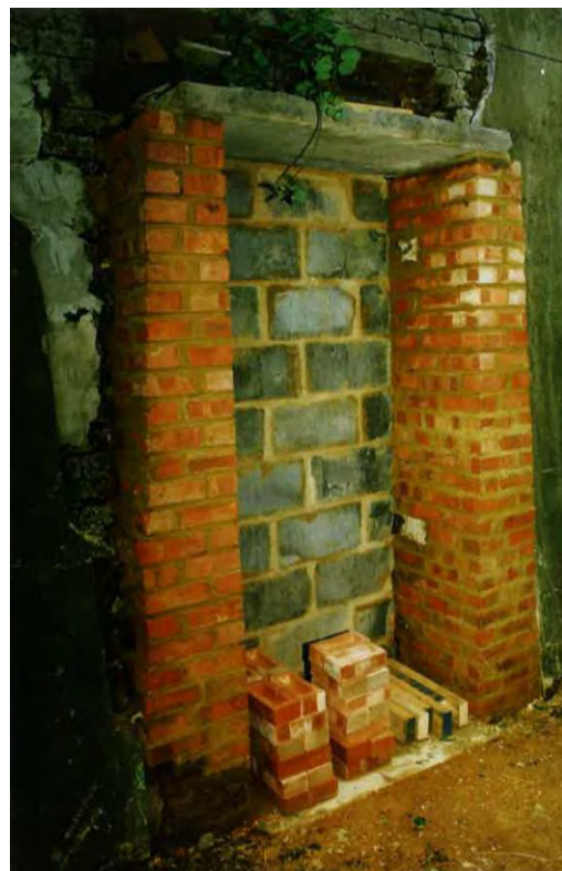
Figure 7: Rebuilt doorway to Vault 13 in 1994
