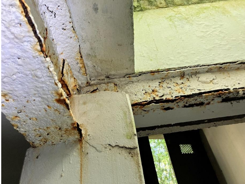
Photograph 14: Otway vault interior – entrance area
