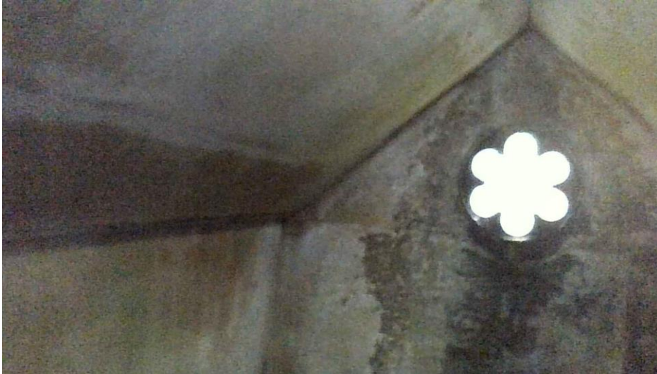
Photograph 18: Foster mausoleum – partial interior view looking west.
