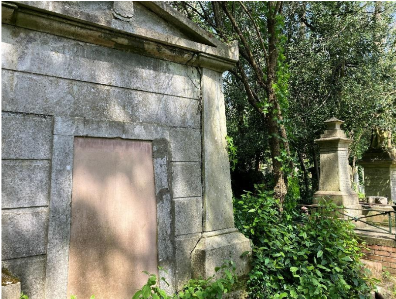
Photograph 20: Da Silva - rotational movement at the south east corner pilaster
