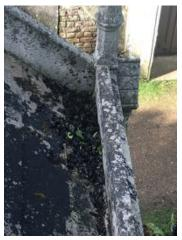
The roof slopes drain to a parapet channel each side, lined with cement mortar, there is substantial build up of leaf mould in the parapet channels.
