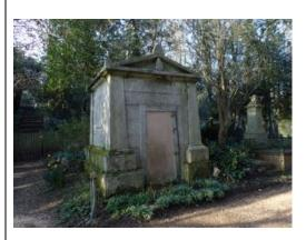
The structure has been much disrupted by tree growth invading the structure itself, some but not all of it now removed. This has left some serious structural issues that need to be addressed by conservation work of some urgency.
