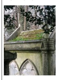
The roof channels need to be cleaned, reviewed and a new detail implemented for rain water disposal.
