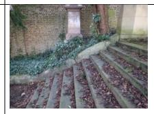
Below the steps is a slope, once surfaced in concrete, but now so degraded as to be effectively unsurfaced - and both bumpy and muddy. Any use for access would require that this is resurfaced.
