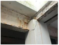
Rust staining defaces many painted surfaces, and rust jacking is starting to affect render/concrete bearings of the beams.
