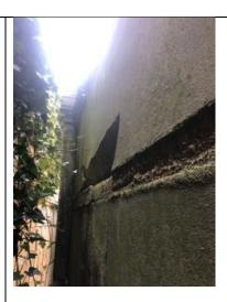
Moulded details to the entrance and corners are eroded and some exposed surfaces are unstable and still eroding.
