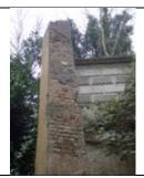
The trailing ivy is picturesque, but full review of the wall heads and the back face of structures will only be possible after full (if temporary) clearance. The most critical area is probably that at the base of the Cory-Wright mausoleum, now infested with brambles.
