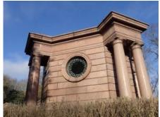
The flat roof has a parapet all round and without access to it the location of a hidden rain water pipe could not be identified. There is a central circular rooflight with a glass dome.
