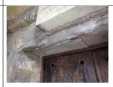
Future repairs should concentrate on water management, with a review of details, drainage and the weatherings to wall heads and cornices. Render repairs will be concentrated on the entrances, to be undertaken in tandem with treatment of the steel door frames.
