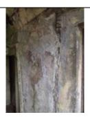
In other places the consolidation in its displaced state of earleir render has remained stable and visually effective.
