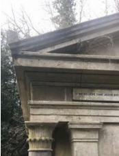
A few joints have mortar loss, notably at cornice/pediment level, where some plants rooted in open joints are starting to have an effect by displacing the masonry. The vegetation is as yet young and light, but it will not take long to become woody and disruptive. It needs to be removed and the pointing made good before that happens.
