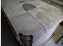
The central one has loose and slightly displaced and cracked slabs in the top, but repair to address these will be minor.
