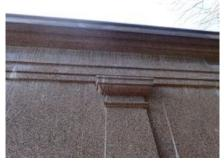
There are rusty steel channels mounted above and below the rear windows which are the remains of a security shutter. These are unsightly, and likely to cause damage, so they should be removed.
