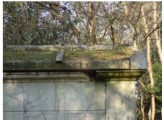
Stone strips mimic lead rolls, and those have broken and slipped down the roof slope. The rear part of the ridge roll is missing. All of this needs to be secured and stabilised, and open joints secured and pointed, even if the situation is simply to be maintained as status quo.
