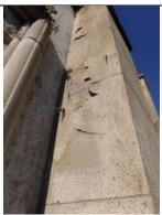
Defects to the surrounds of openings are largely due to corroding ironwork, and they DO need attention. Render door surrounds are cracked, and the stone doorcases have broken stones, notably to WV1 and WV2 where corroding iron door frames have triggered the worst cases. Repairs including rust treatment and isolation are needed. Similarly the steps to vaults WV1, WV2, EV1, EV2 all have open joints which need to be repaired to prevent escalating defects.
