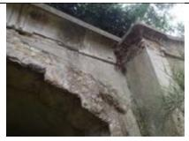
On the outer side of the portal the wall head forms a substantial parapet to the footpath above. There are some cracks in coping joints but only minor repairs are essential. This parapet, at approx. 900mm high, does not meet current regulations for the context but it is substantial and safe in the context of the Cemetery. The protection of the dangerous drop to the other side (into the Avenue cutting) is only a low iron railing and a split lath fence, and this needs to be reviewed.
