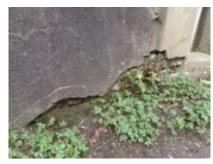
The doorcases are generally in good order other than the abutment of the steel door frames (see below) and they have neat and sound lead capping which will discharge the rainwater effectively if they are cleared of vegetation debris.
