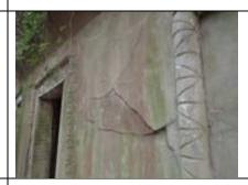
The worst degradation is to the vault entrance reveals and soffits where moisture above drains out through the structure and where the steel door frames abut. Several door soffits are affected, the worst at EA15 where render is detaching in lumps now.
