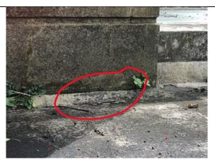
This could and should be improved, using a contractor with sophisticated skills in asphalt work. It drains to a simple outlet at the 'uphill' end.
