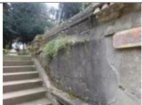
The vault facades are less damaged than those to the Inner Circle, and as there the previous conservation works have served well. Vegetation taking a secure hold should be removed and holes stopped up. Minor render defects can be addressed by ongoing cyclical repairs.
