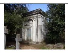
The sides are plain below a large projecting cornice. The back elevation has two flat lonic pilasters flanking two windows with cast iron grilles. The front elevation has two engaged but round lonic pilasters set in antis either side of a pedimented door case.
