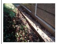
The perimeter wall and steps are sound enough in themselves, but there has been some substantial movement of the steps and joints between them and the plinth have opened by nearly 40mm. This needs to be monitored and stabilised. The steps remain entirely usable.
