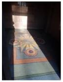
The floor is elaborately patterned in coloured ceramic mosaic, with a central lifting panel for access to vault below. The interior is empty.
