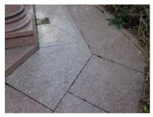
However, there are extensive open joints and a programme of regular minor repairs should delay the onset of any serious defects.
