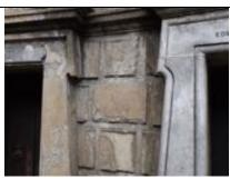
Diagonal cracking in the upper corner to steps (2) clearly allows water through it as there are heavy calcium deposits, but it does not appear to be progressive.
