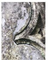
Here the movement has also disrupted the sealing and fixing of the adjacent inscription slab. This, and others, may need refixing and grouting of voids.
