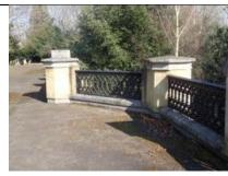
The tarmac terrace surface has cracks, cracks at joints and low points all of which encourage and harbour plants and moss. This is a self-perpetuating and escalating problem which needs to be addressed. Each low point relates to a drain, but the organic growth makes it apparent that these hold water, at least temporarily.
