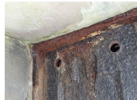
Figure 17. Rust-jacked frames have made access to some vaults difficult
