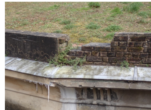
Figure 16. Evidence of previous repairs from 1990's works.
