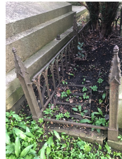
Figure 3. Damaged railings providing robust evidence
