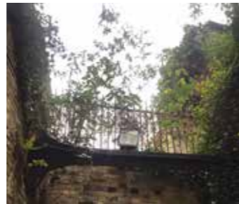
Tunnel Cutting, view up.
