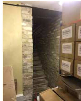
Access stair, bottom
