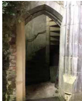
Access spiral stair
