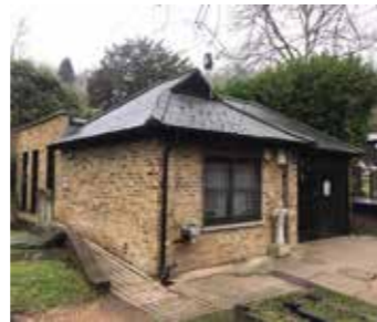
Exterior of East Compound.
