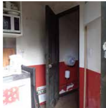
Kitchenette & WC (© WSA)
