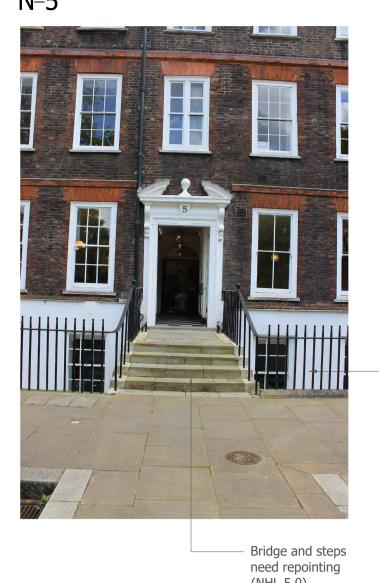
Railing repairs and redecoration. Pieced-n stone repair to damaged stone
