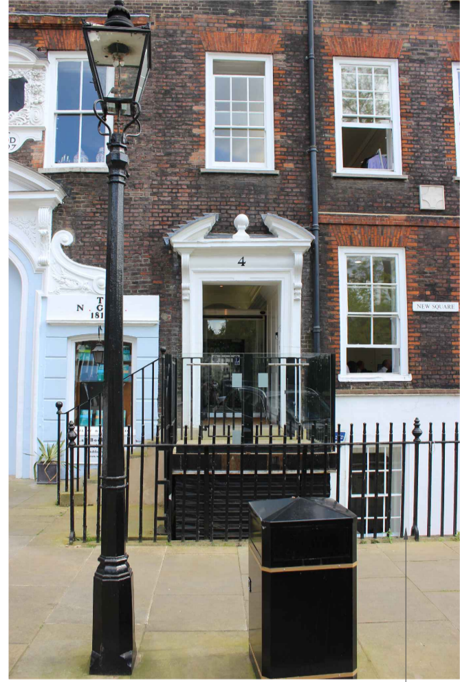
Railing repairs and redecoration. Pieced-n stone repair to damaged stone
