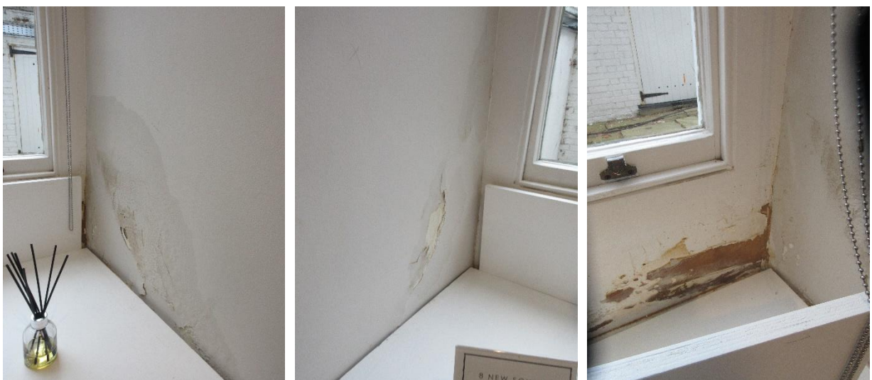
Above left: Damp to the south reveal of WB04 in Room 8BNS/B3.
