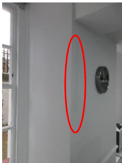
Above left: Damp patch to south side of WB04 in Room 11NS/B9.
