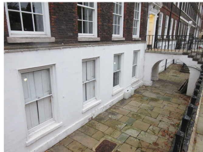
No9 New Square (South)
