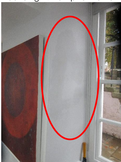
Above left: Large damp patch to the north of WB06 in Room 11NS/B10.
