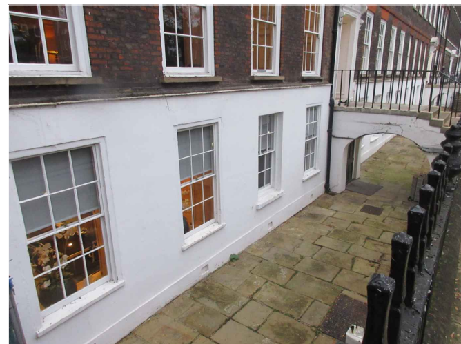
No8 New Square (South)
