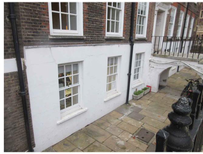
No 11 New Square (South)
