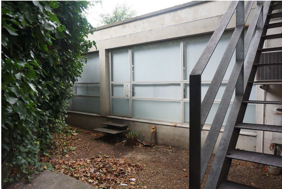
View of the West Block's south elevation facing its courtyard
