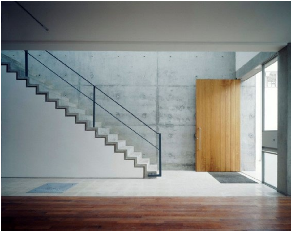
View of the entrance hall to the Central Block showing the in-situ concrete stair and spine wall
