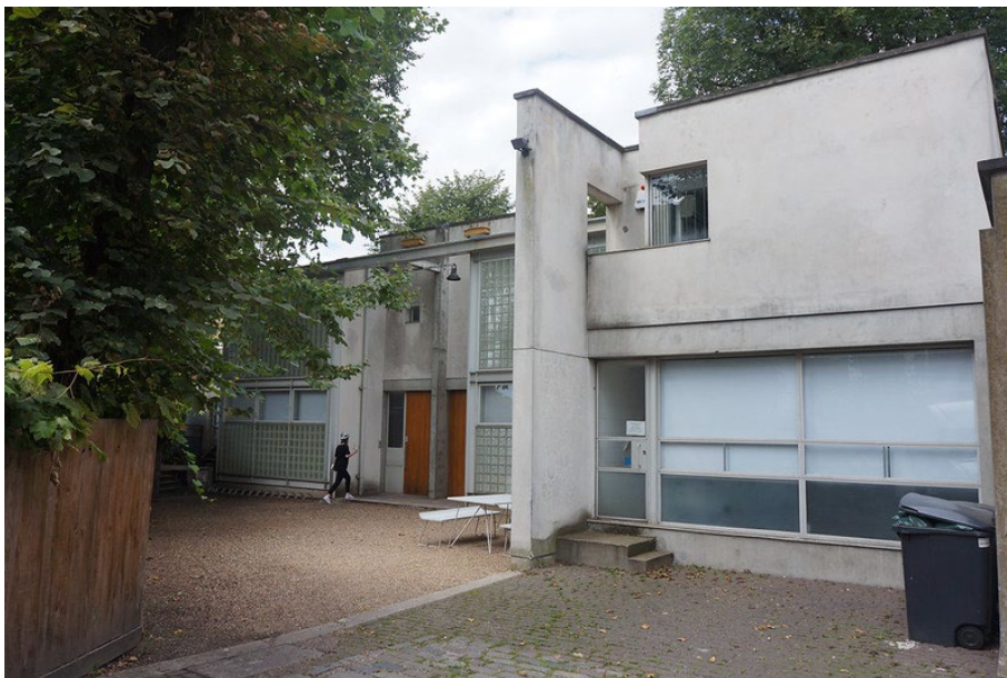
View of the small East Block with its south elevation on Cobham Mews
