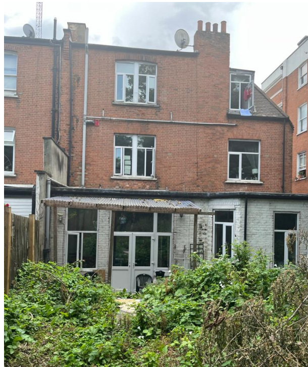
Photograph 4 Existing Rear Extension
