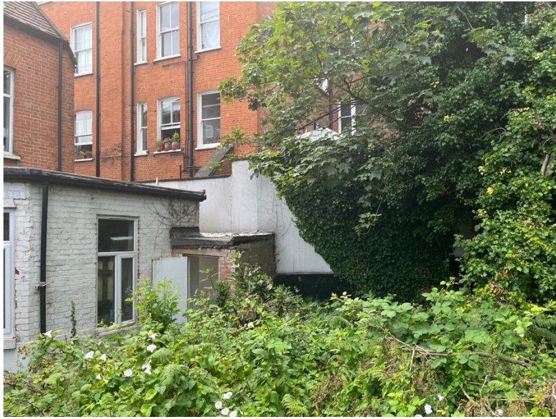
Photograph 5 Existing Rear Extension towards Lymington Mansions
