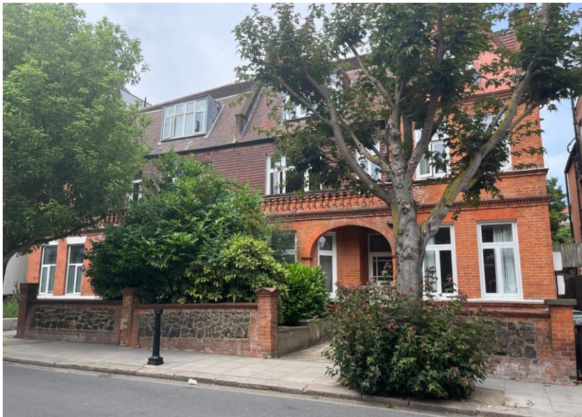
Photograph 2 Front Elevation with No.3
