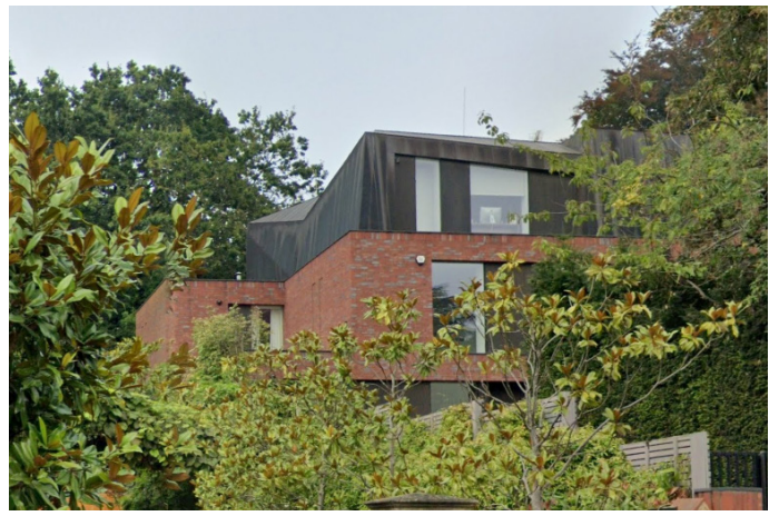
17 Templewood Avenue - Large single paned 'frameless' glazing, with 'floor to ceiling' appearance
