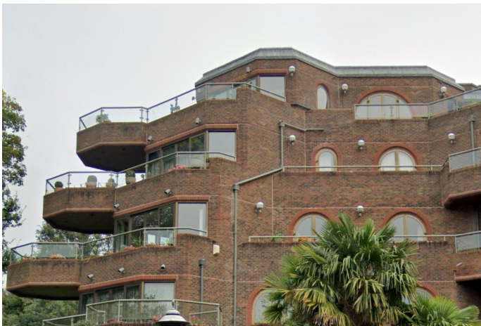
Heath Park Gardens - Large single paned windows with bronze frames, and occasional arched lintels
