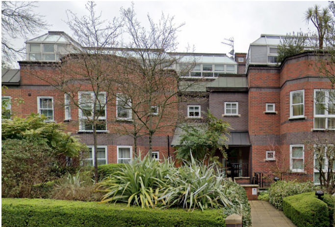
Temple Heath Lodge with white timber frame windows + white aluminium curtain walling to the roof extension
