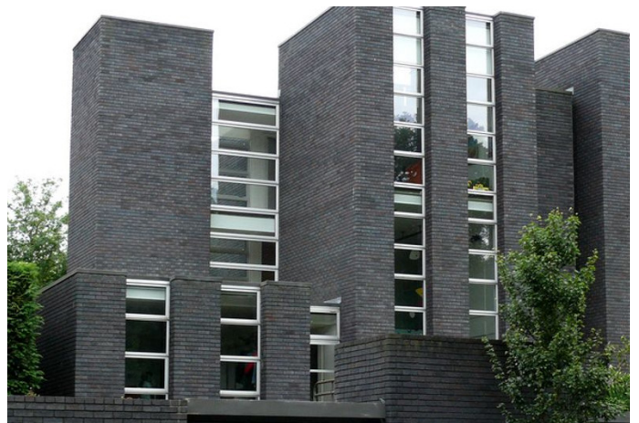
Schreiber House (Adjacent Site) - Horizontally oriented galvanized frames
