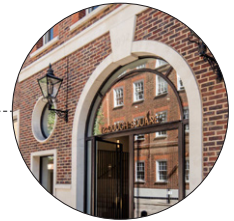
Bronze coloured, metal-framed windows
