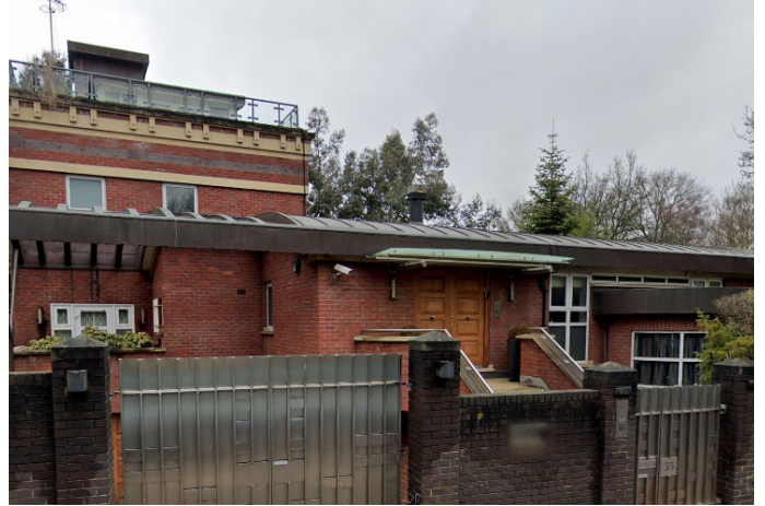
"The Site" 35 Templewood Avenue with a mix of white aluminium and PVC windows
