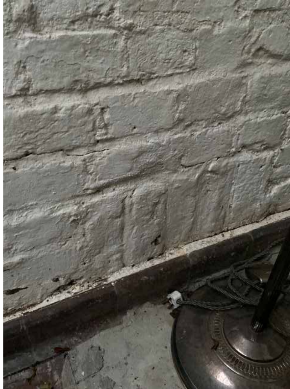
Figure 3.7 Photograph of brick arch in the rear ground floor extension of 28 Charlotte Street.
