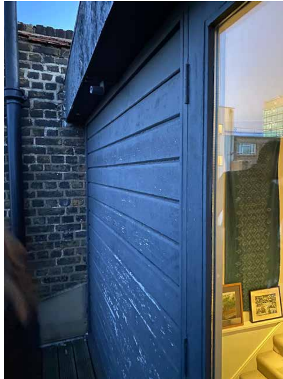
Figure 3.20 Steel door on fourth floor attic conversion.
