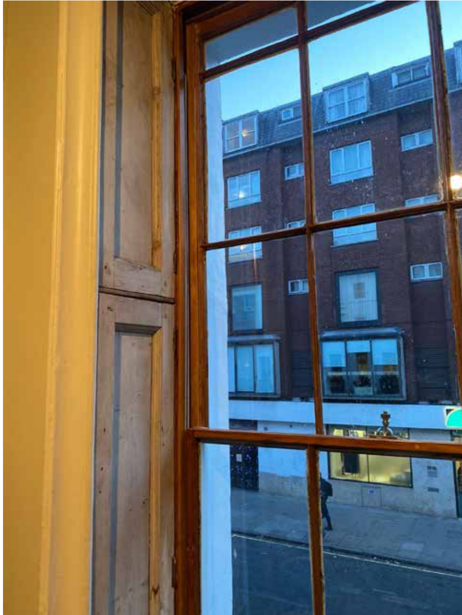
Figure 3.14 Photograph showing the original timber sash windows, shutters and architrave surrounds.
