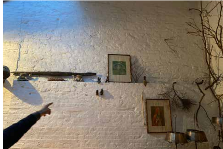
Figure 3.10 Masonry step in wall of 28 Charlotte Street.
