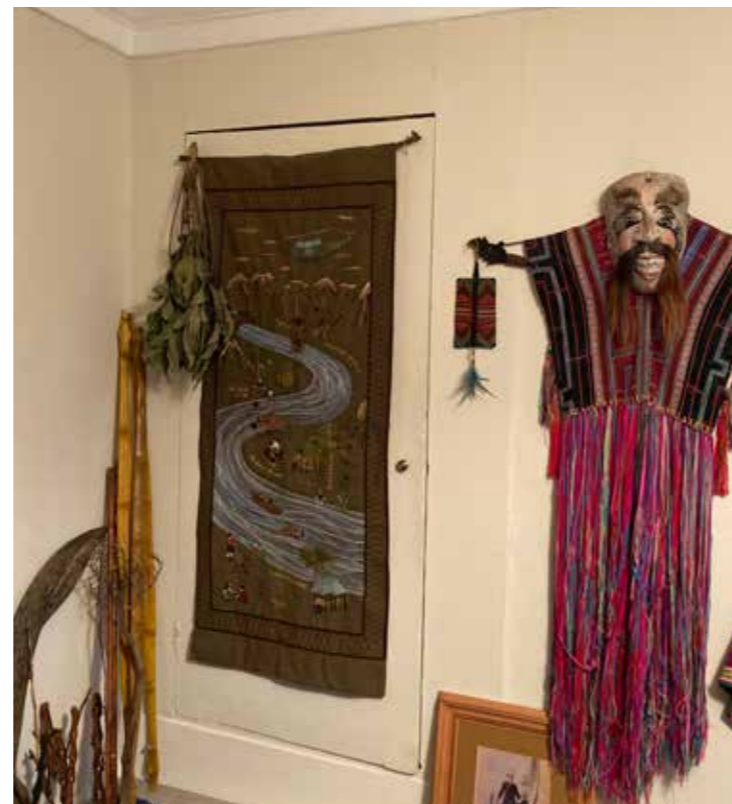
Figure 3.18 C19 fire place cupboard which survives in the second-floor rear room.
