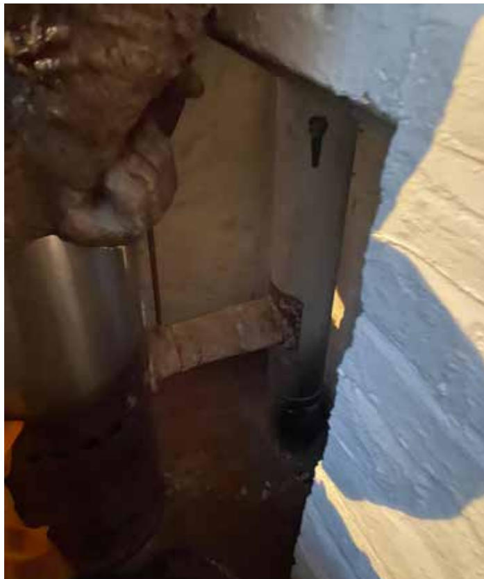
Figure 3.9 Fireplace in rear extension of 28 Charlotte Street.
