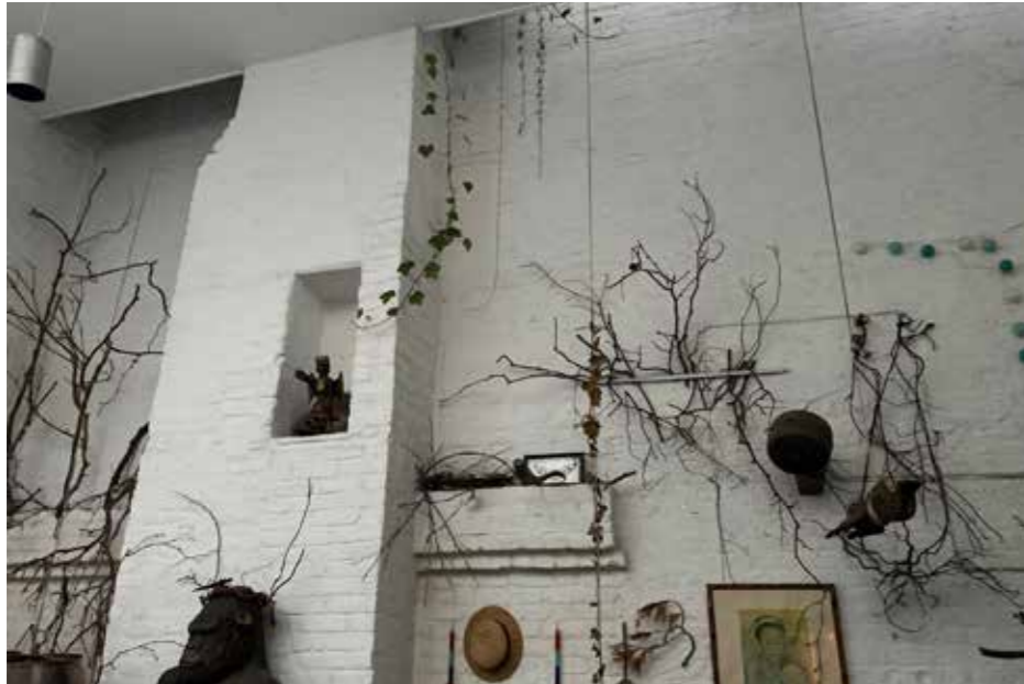
Figure 3.8 Chimney breast in rear extension of 28 Charlotte Street.
