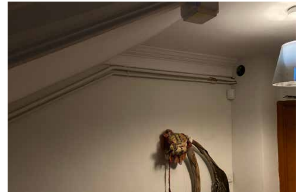
Figure 3.19 Original cornicing on second floor landing.
