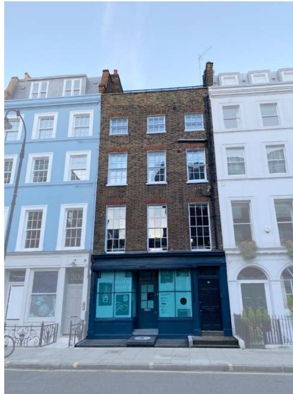
Figure 1.1 Photograph of the front elevation to 28 Charlotte Street and in context as part of the terrace
