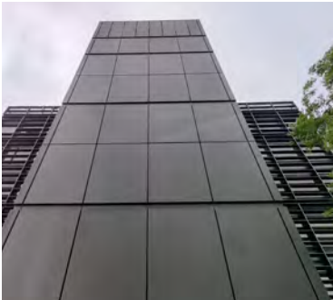
Exterior Alu flat panel removal
