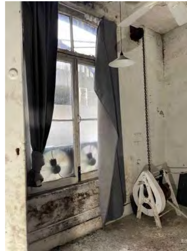
Existing winch mechanism
