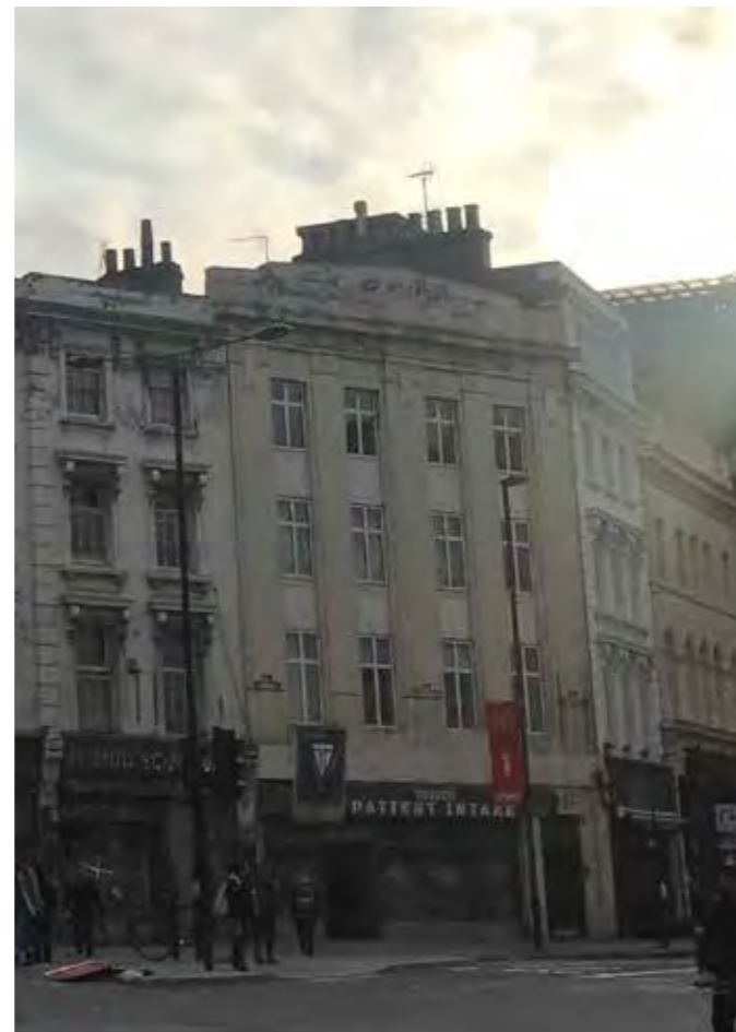
Existing Facade Overview
