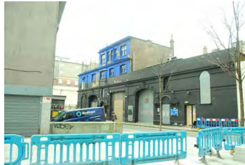
Existing Facade Condition as seen from Museum Street
