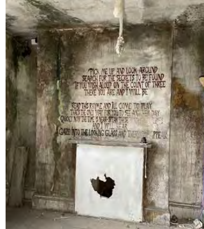
c1860 fireplace behind boarding
