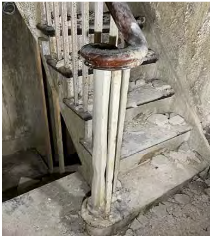
c. 1830s Staircase, Twisted mahogany handrail and stick balusters.
