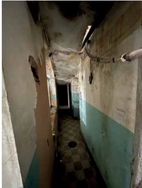
Coal vault corridor connecting 11 and 12
