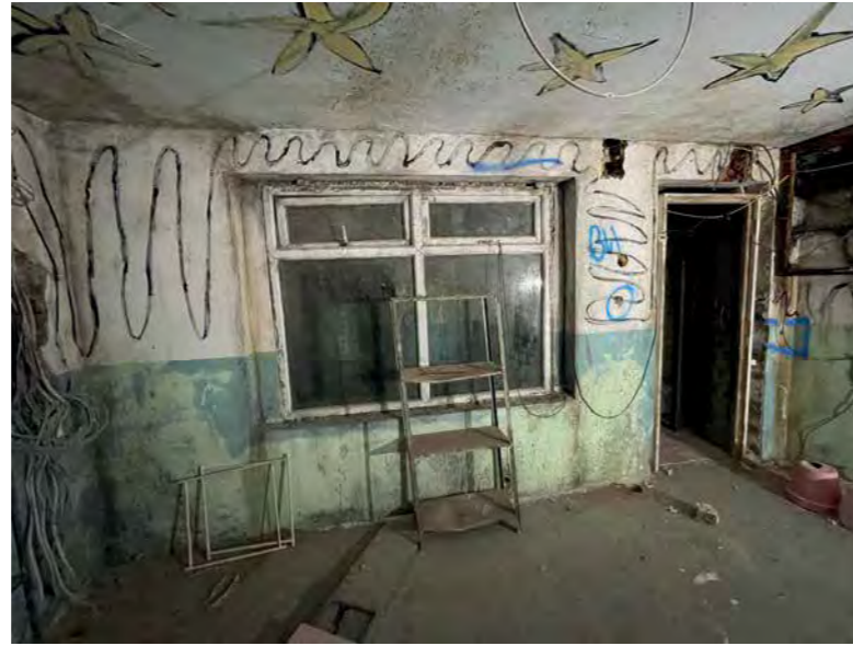
Front room. Note modern uPVC window
