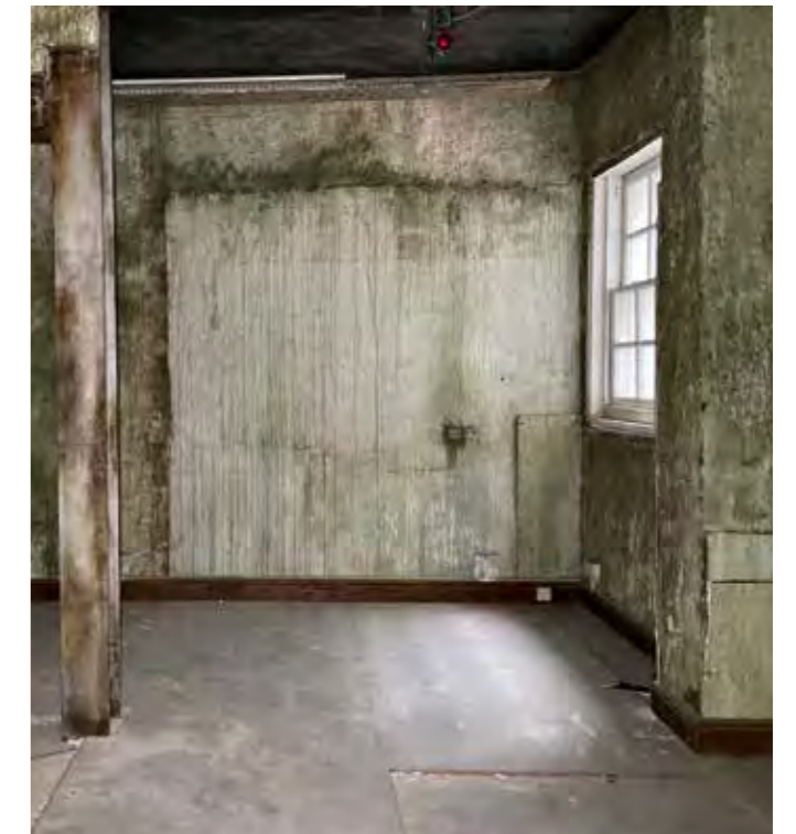
Area rebuilt in 1990s, new joinery.
