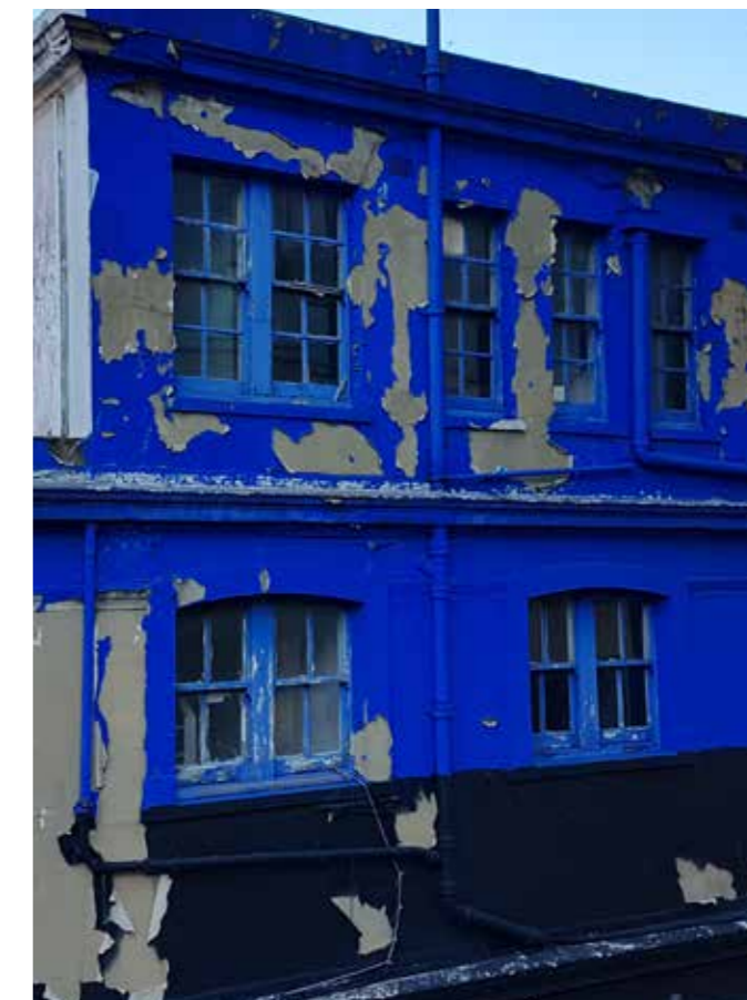
Existing Facade Condition
