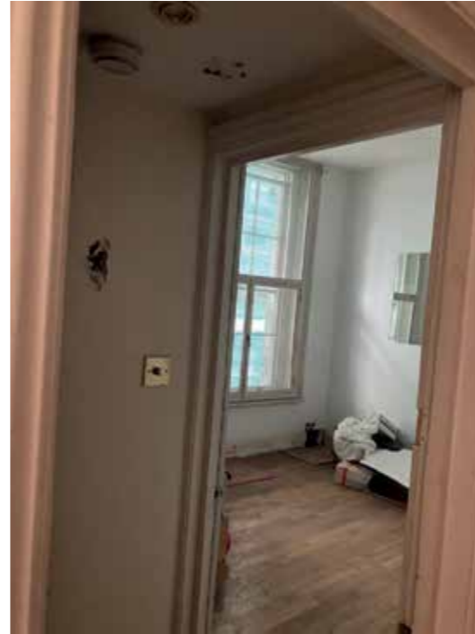
View to front studio flat of no.11 from stair landing
