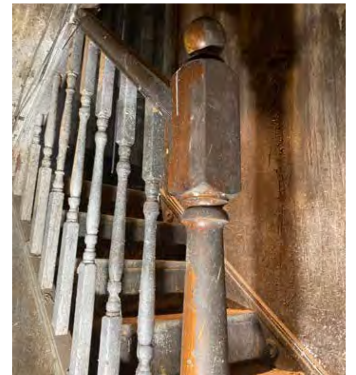
Modern balustrading, treads, risers and stringers cladding. (35 NOST.)
