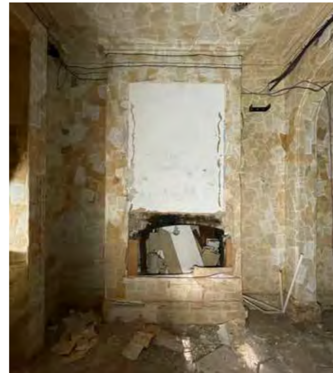
Partially infilled fireplace opening. Cornice and architraves of early phases.
