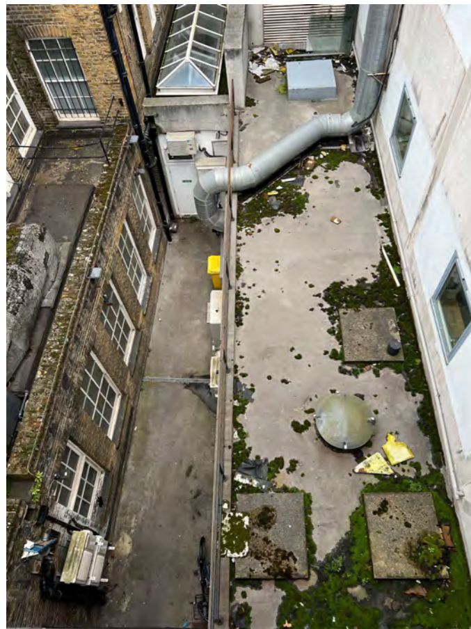
Site photo of 15 Grape St. fire escape route
