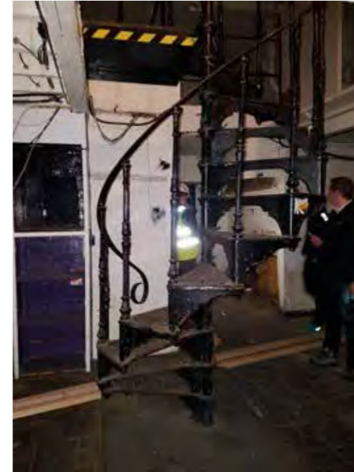
Existing cast iron staircase
