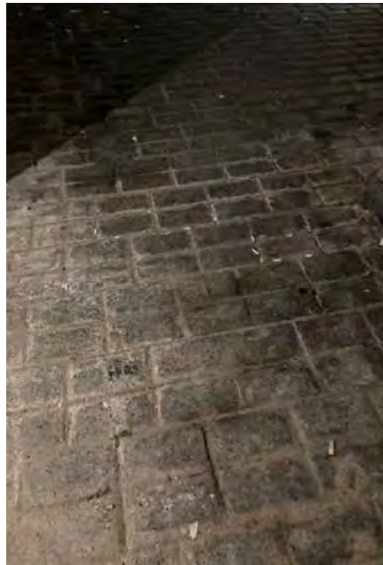
Existing floor Setts
