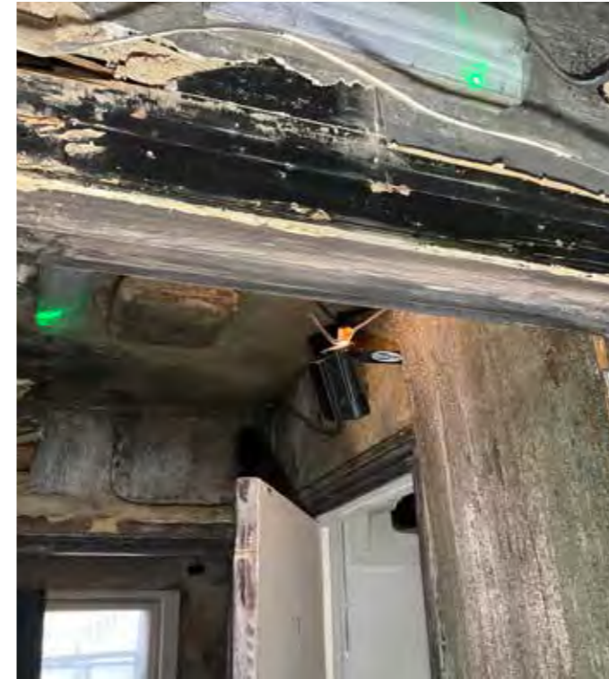
Mix of modern and historic joinery. (35 NOST.)
