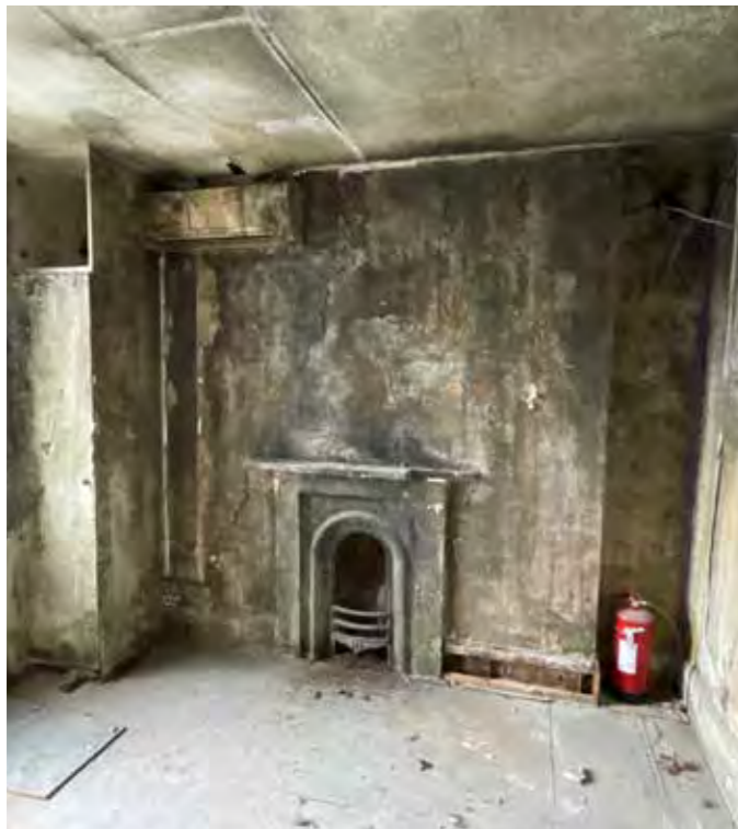
Historic fireplace including decorative arched cast-iron register grate, some joinery, lath and plaster and floorboards.
