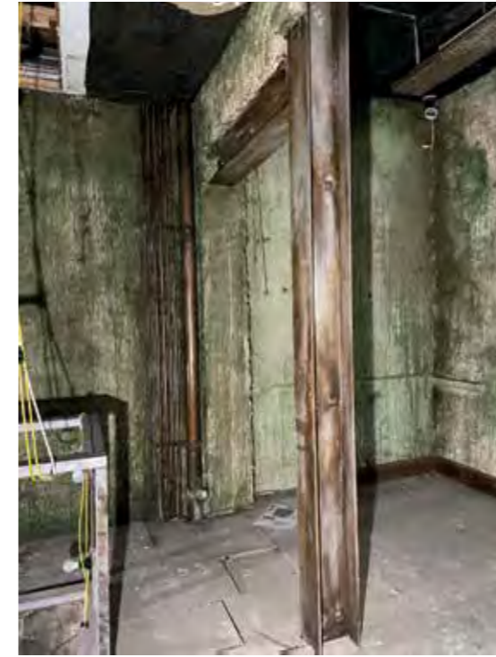
Ground floor of no. 11
