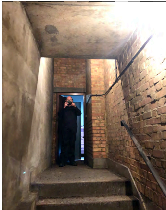
Ground floor access to stair going down to basement
