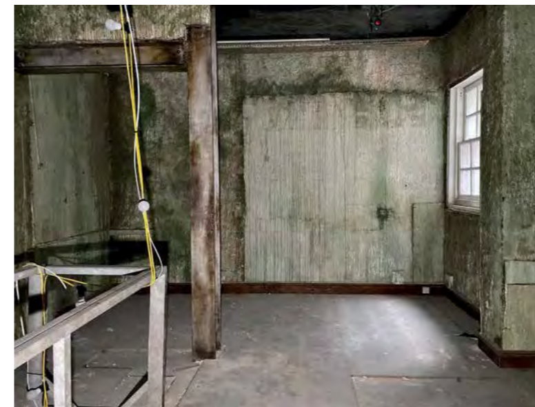
Ground floor of no. 11
