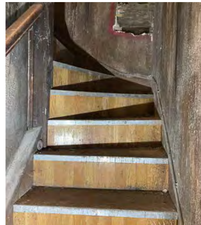
Modernised and substantially rebuilt staircase. (37 NOST.)
