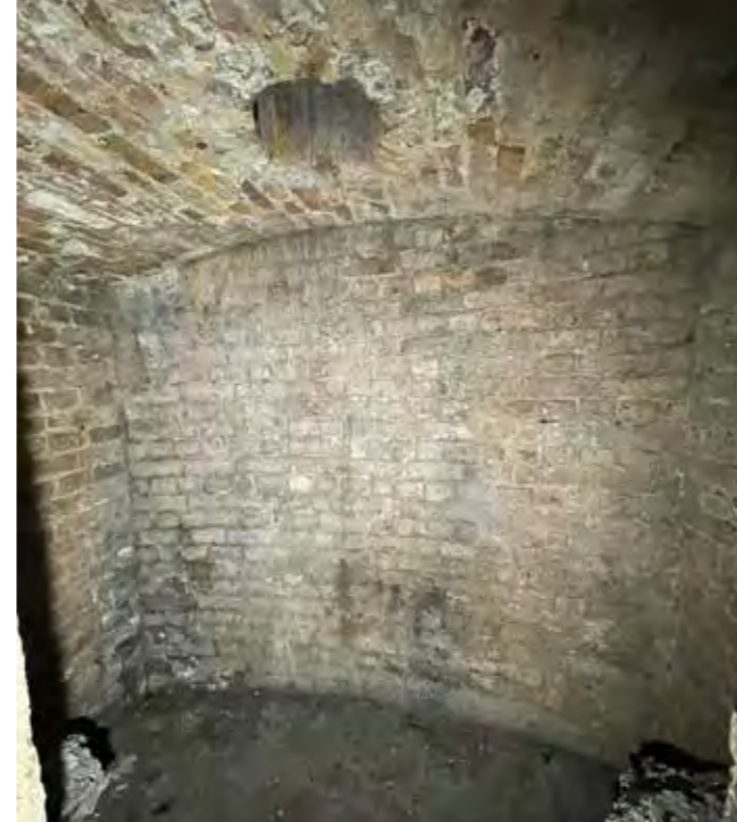
Front vaults and coal hole
