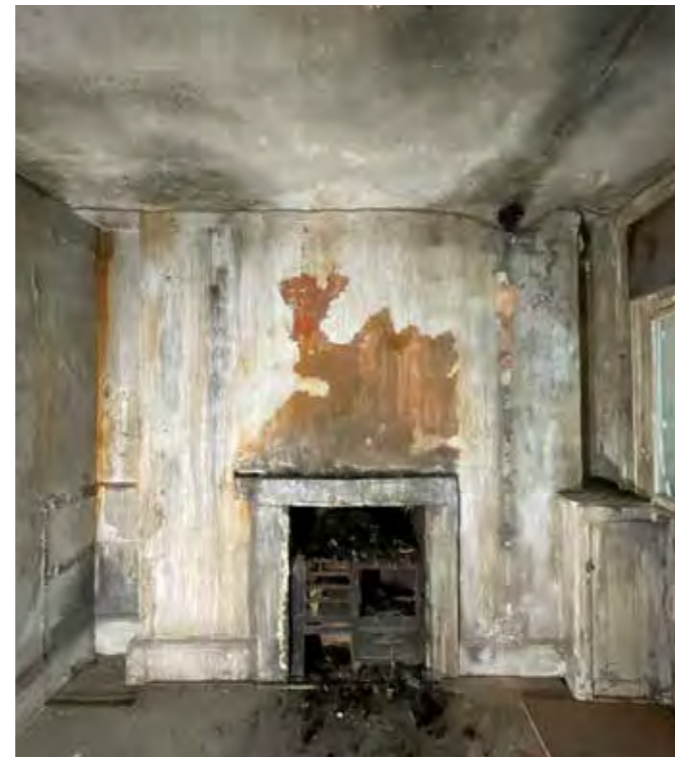
Cast-iron cooking range in front room with one surviving fitted cupboard to side
