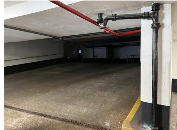
Existing car park ramped slabs
